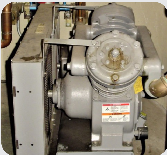
Reciprocating Piston Air-cooled Laboratory Compressor
