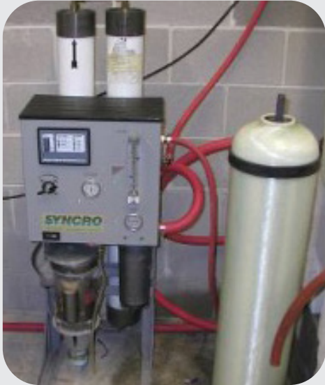
RO Filters at a Car Wash
