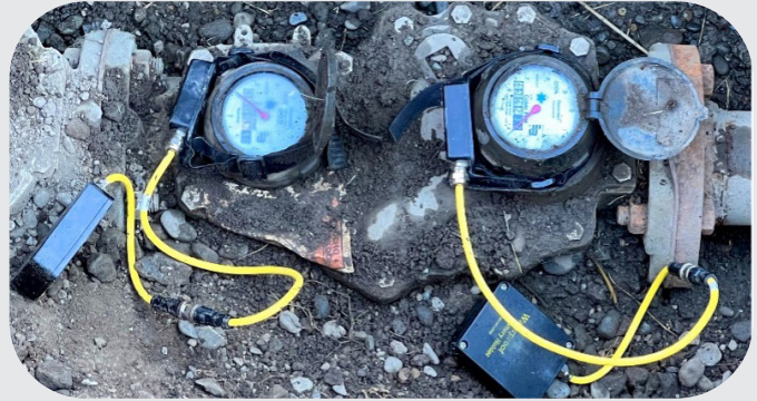
Data loggers on two water meter dials
