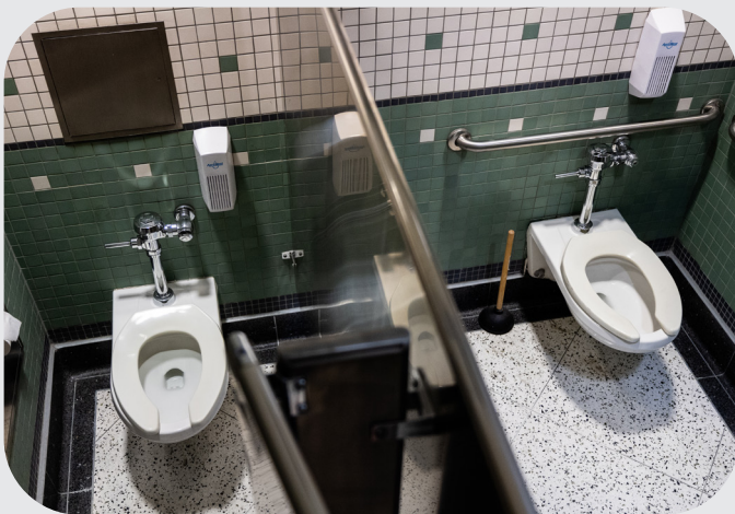
Two Flush Valve Toilets
