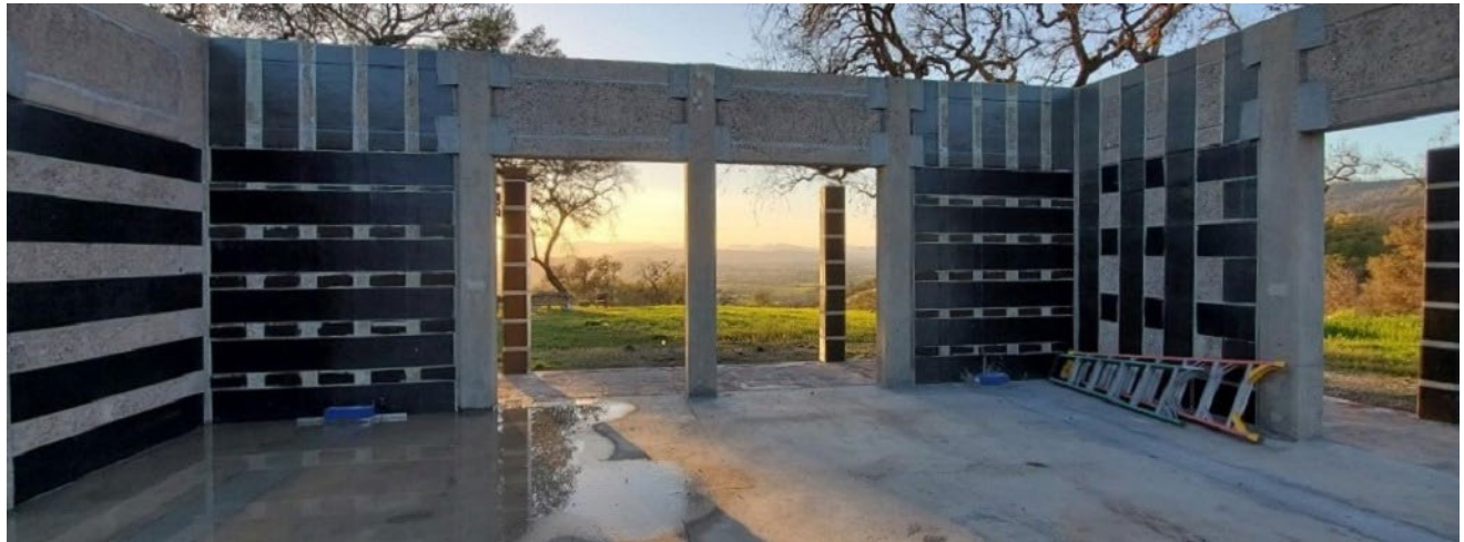
Figure 7-5. Example FRP Reinforcing; seblog.strongtie.com
