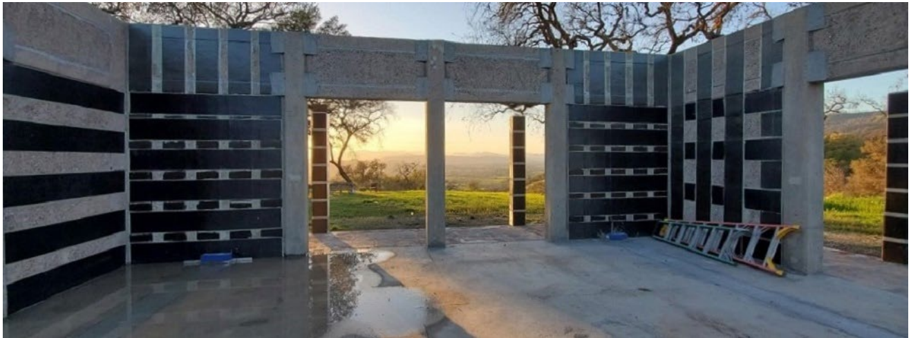
Figure 7-5. Example FRP Reinforcing; seblog.strongtie.com
