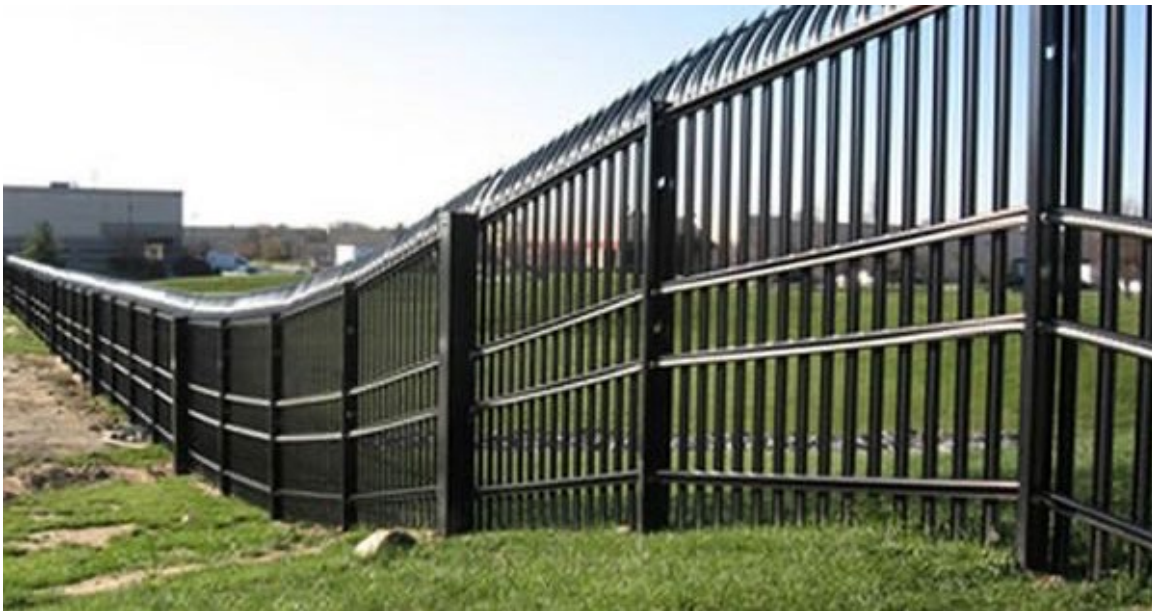
Fences with a Green Belt and sidewalk between a street as a buffer zone:
