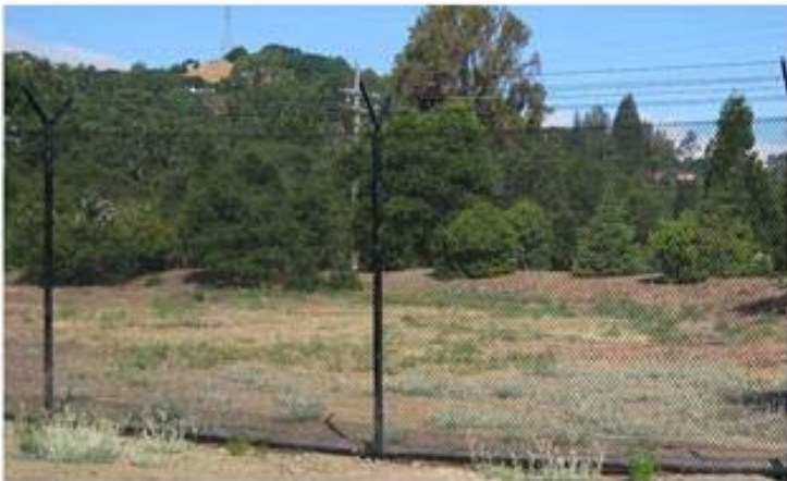
SECURITY FENCE 8-foot high, 1-inch black vinyl coated mesh with barbed wire
