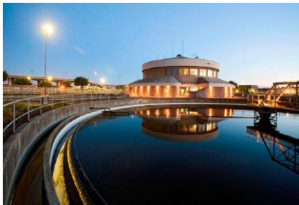
Main Wastewater Treatment Plant
