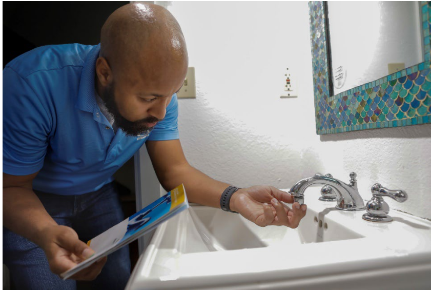
Figure 16. Installing an aerator on a bathroom faucet.
