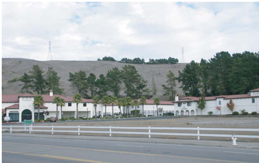
F3. Looking northeast from Moraga Road south of Rheem Boulevard
