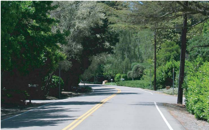
G3. Looking southwest towards the intersection of Glen Road and Nordstrom Lane
