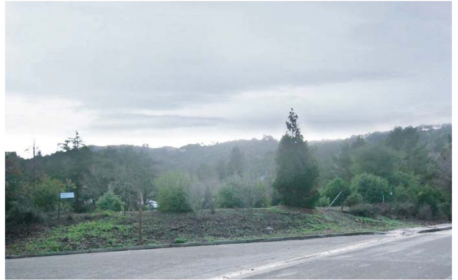
O6. Orinda WTP looking south from Manzanita Drive*
