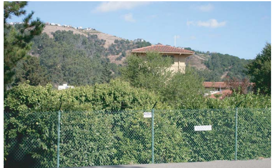
U4. Upper San Leandro WTP looking northeast from Greenly Drive
