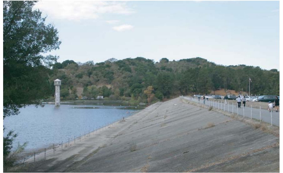
H2. Looking northwest across Lafayette Reservoir Dam
