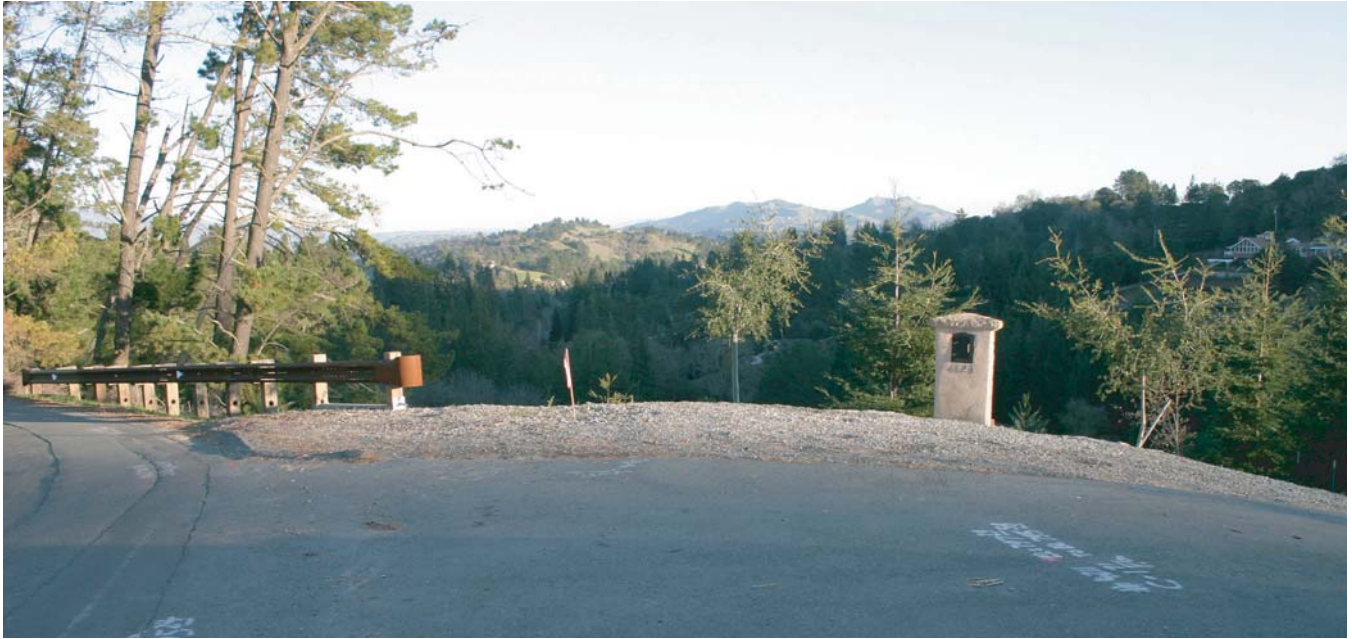
Existing View looking southeast from Happy Valley Road at Proposed Sunnyside Pumping Plant entry road
