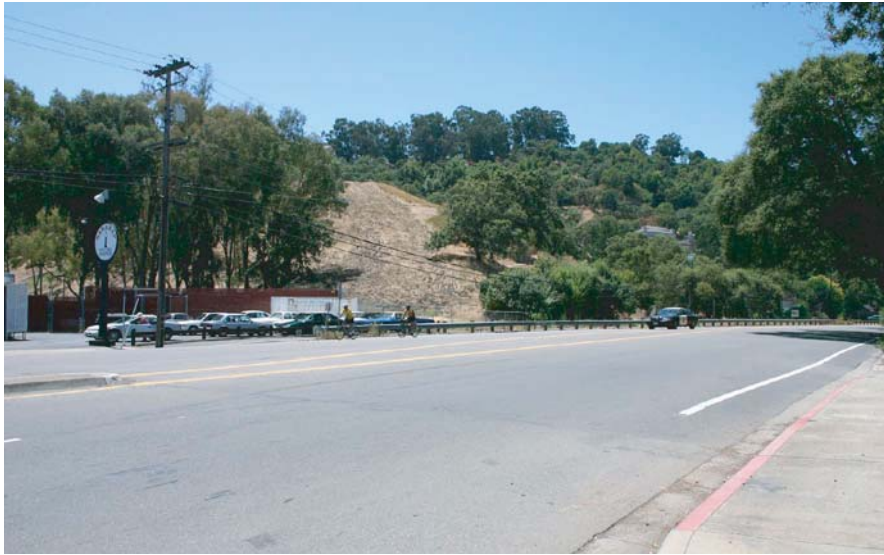
T1. Looking southwest from Olympic Boulevard at Tice Valley Boulevard
