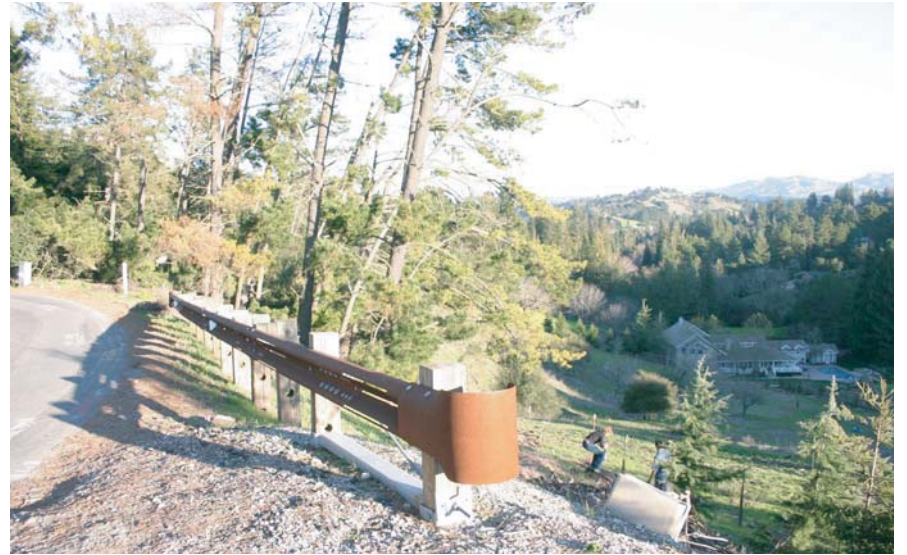
SS2. Looking southeast from Happy Valley Road
