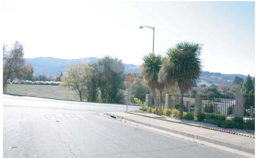
S8. Looking south from Heavenly Ridge Lane near Amend Road
