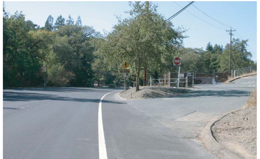
L8. Looking west from Mt. Diablo Boulevard at WTP Exit Road
