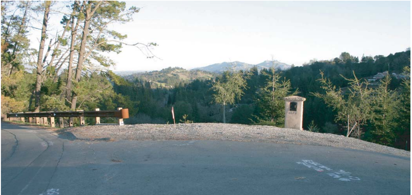
Existing View looking southeast from Happy Valley Road at Proposed Sunnyside Pumping Plant entry road
