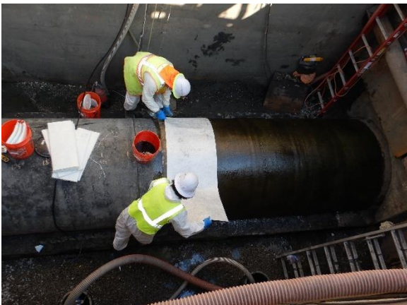
Photo 2-13. Fiberglass wrap layers were installed to reinforce the pipe.
