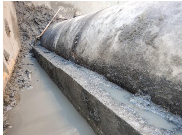
Photo 2-16 Pipe support cradle was in good condition.
