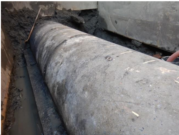
Photo 2-15. Exterior surface of pipe was in good condition.
