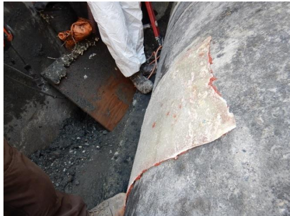
Photo 2-12. Patch over concrete breach before fiberglass repair.
