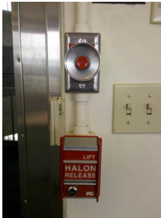
Figure 19. Halon Manual Release and Abort (typical for both Ops Control and Computer Rooms)
