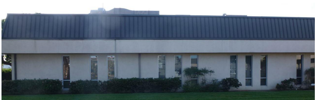
Figure 4: The Original Admin Building and Addition (left) – View from East
