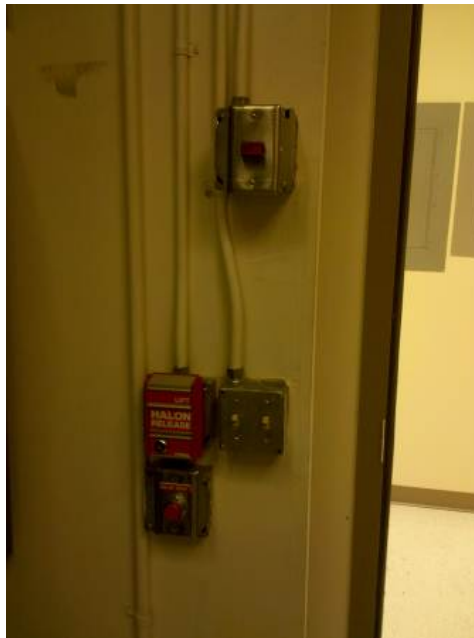
Figure 5. Halon Manual Release and Abort
