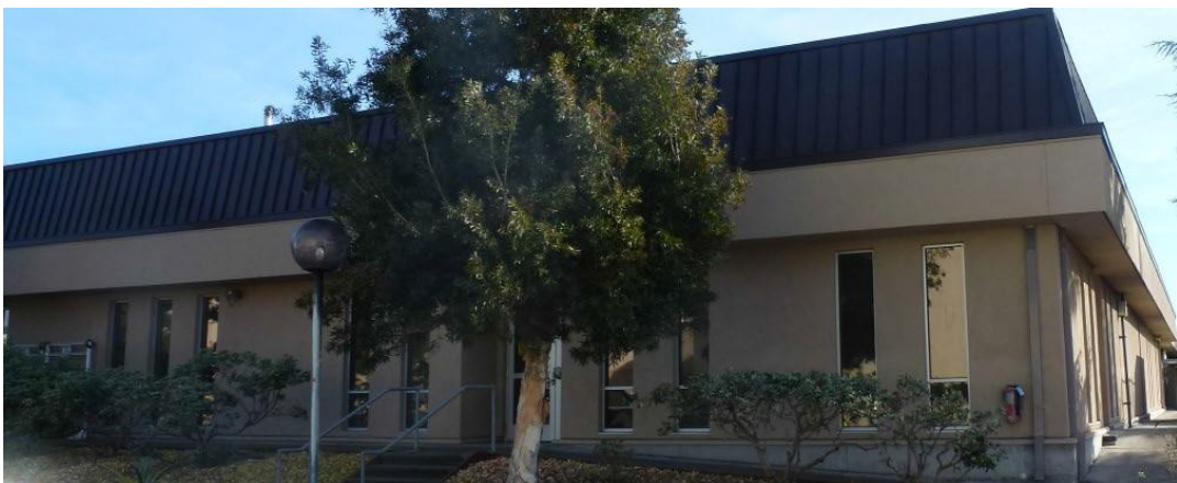
Figure 6: North Lab Addition – Northwestern Corner
