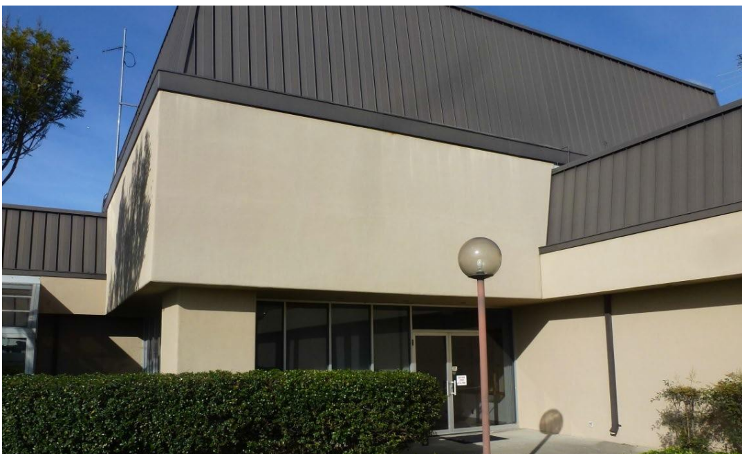
Figure 7: The Two-Story Pop-Up Portion – View from South
