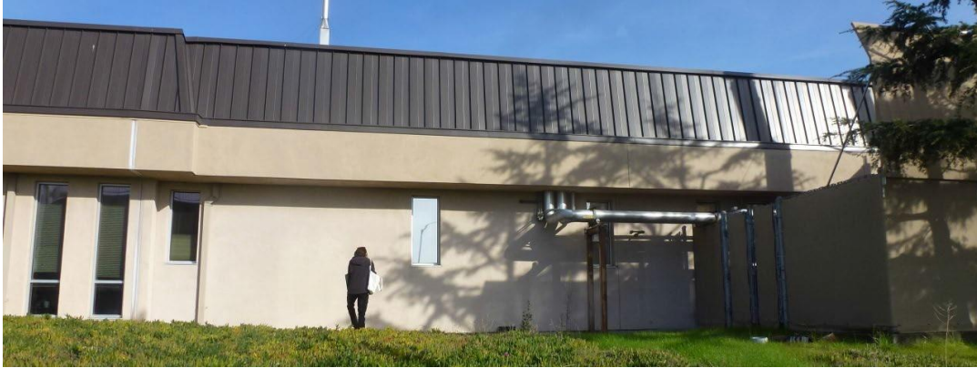
Figure 5: West Lab Addition – View from West
