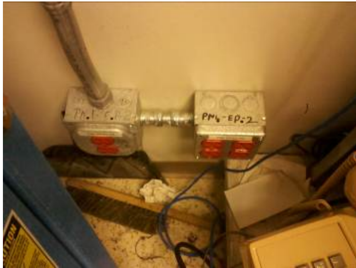
Figure 9. Emergency Generator Power Circuit (Red outlets)
