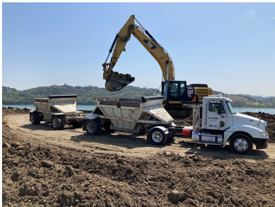
Figure 4: 13 CY Double Bottom Soil Removal Truck Loaded by Excavator
