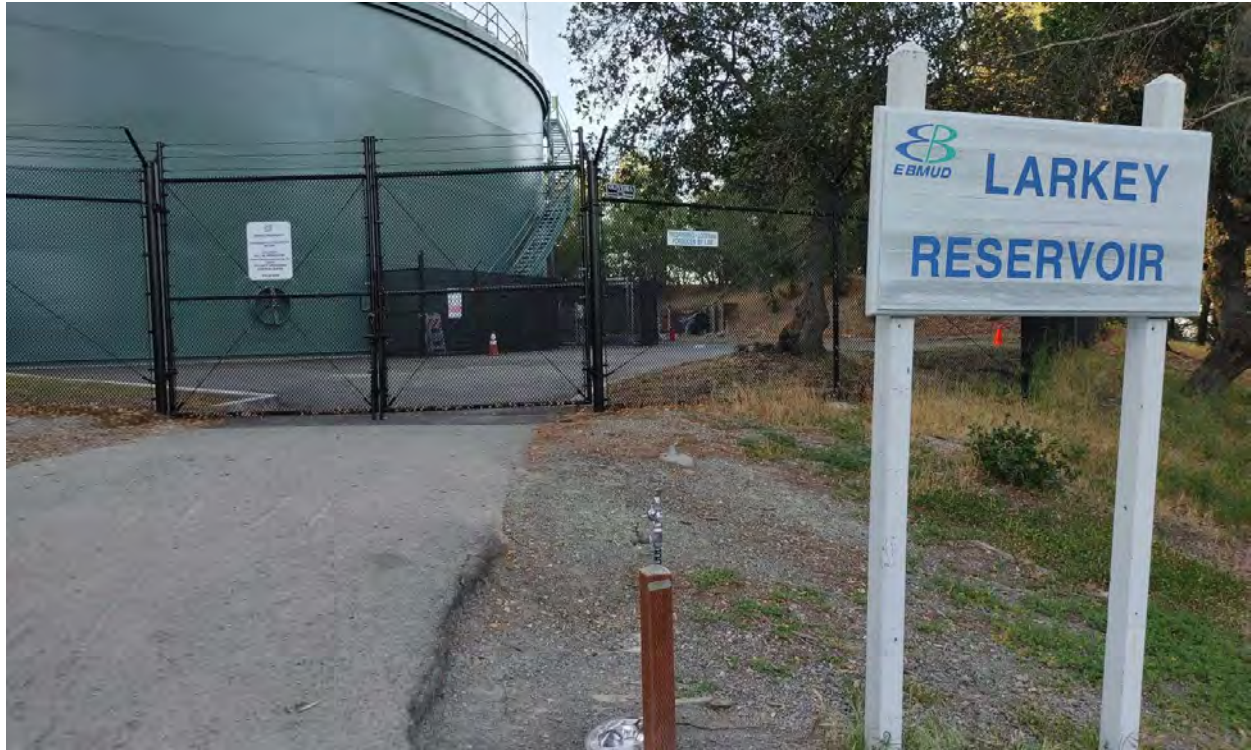
Figure I-12: Larkey Reservoir, facing north (noise meter not pictured)
