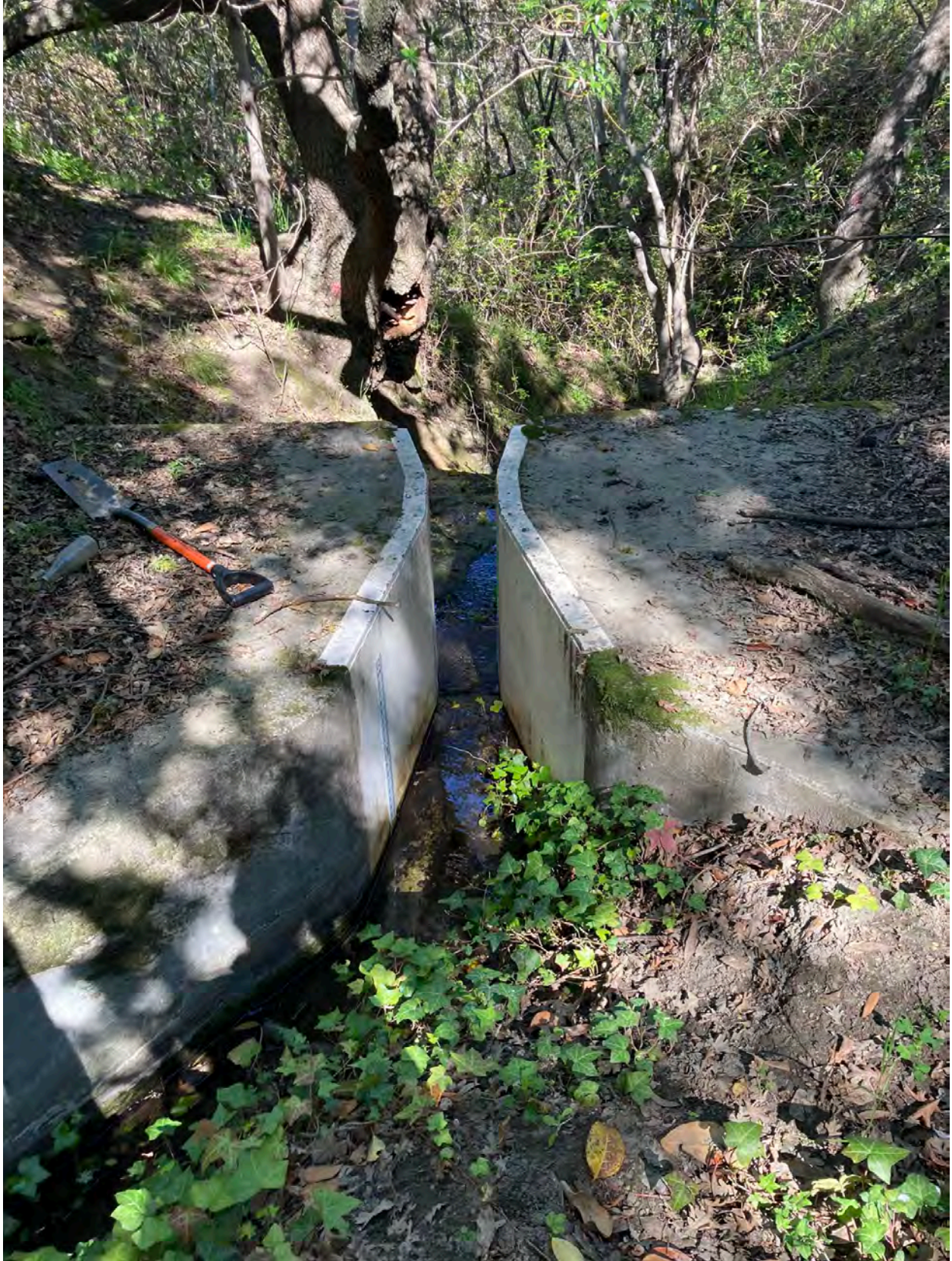
Photo 2. IC-1 flows through a concrete weir that measures water flow. Photo facing north. March 8, 2022
