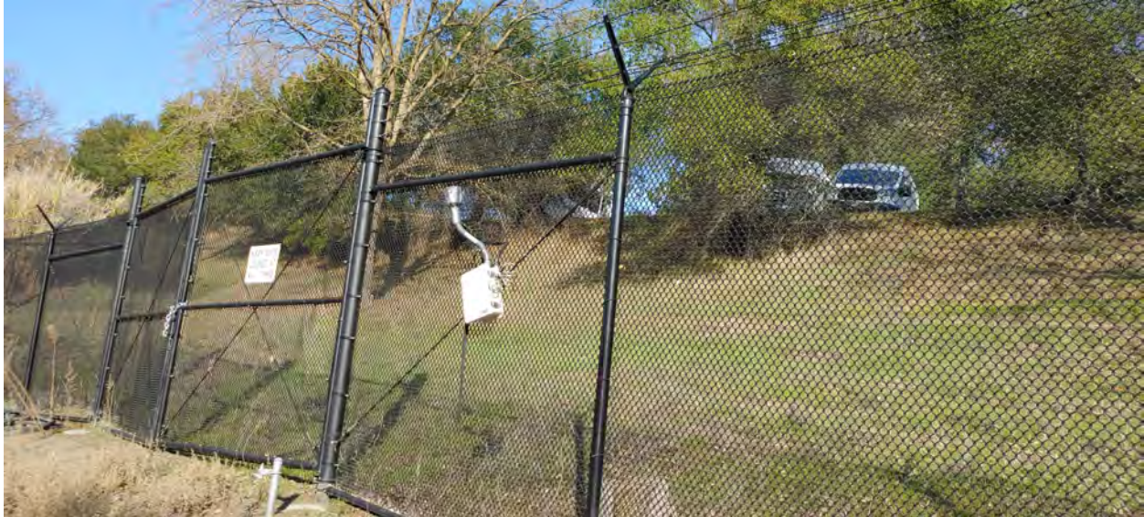
Figure I-8: LT-4 at Lafayette Water Treatment Plant, facing northeast
