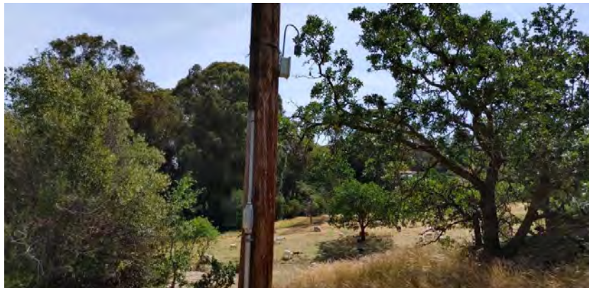
Figure I-6: LT-2 at the Briones to Mt. Diablo Trail, behind 1305 and 1309 Ramsay Circle, facing southeast
