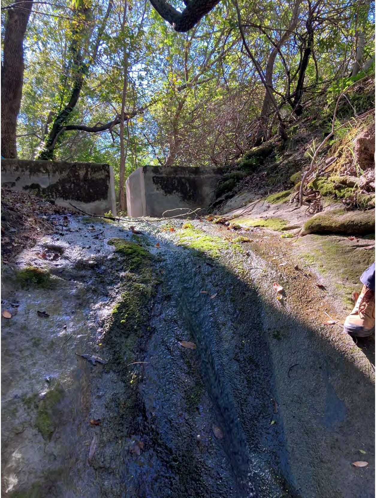
Photo 3. Through the weir IC-1 flows down a concrete lined channel approximately 10 feet high. Photo facing south. March 8, 2022
