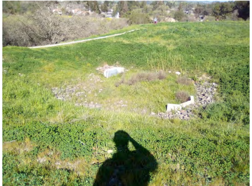
Photo 23: View of the stormwater detention basin, as viewed from the south.
