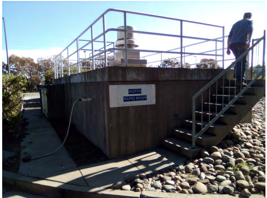
Photo 11: View of the north rapid mix, as viewed from the northwest.
