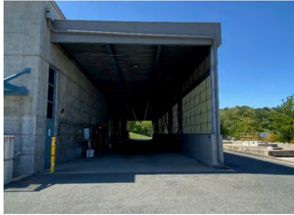
Figure 23- Metal Canopy at Chemical Storage Building
