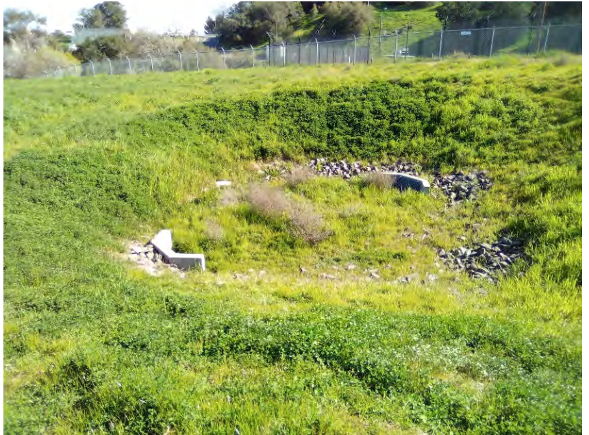
Photo 24: View of the stormwater detention basin, as viewed from the west.
