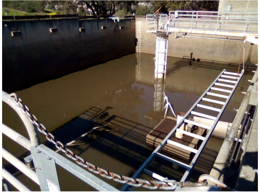
Photo 21: View the solids detention basin, as viewed from the south.
