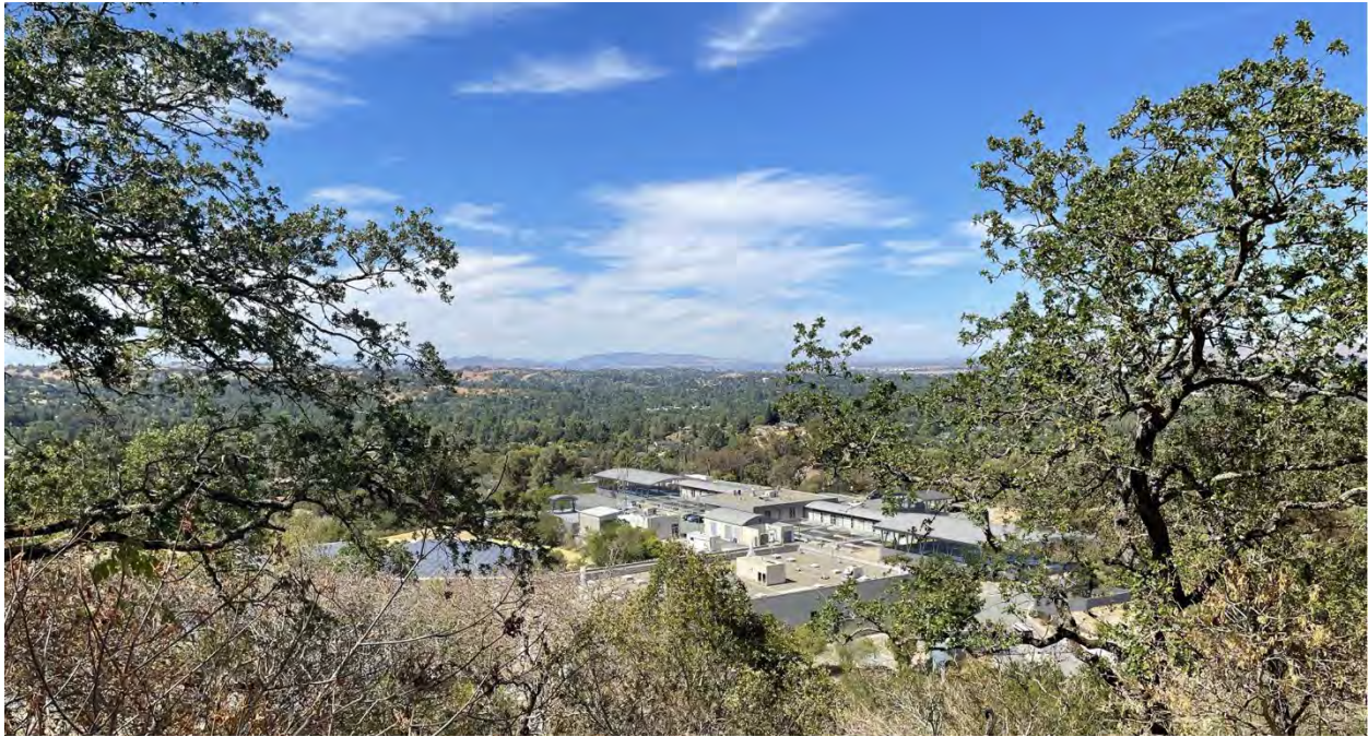
Figure 51- View 2_After Construction
