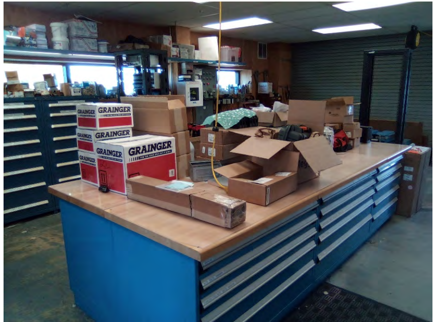
Photo 8: View of the interior of the electrical instrument control building.
