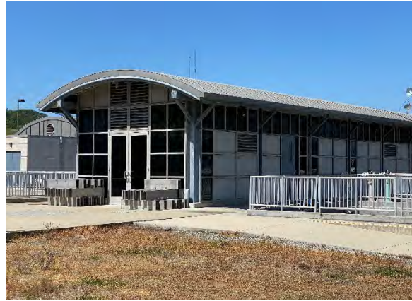
Figure 42- Standing Seam Roofing
