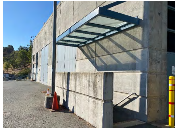
Figure 46- Steel Canopy with Glass
