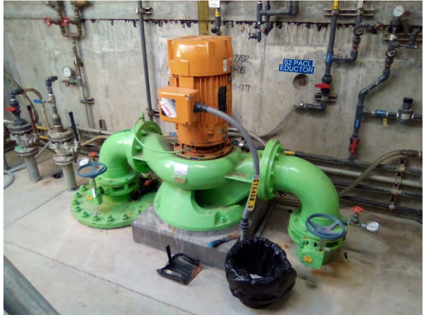
Photo 3: View of the interior of the south rapid mix.
