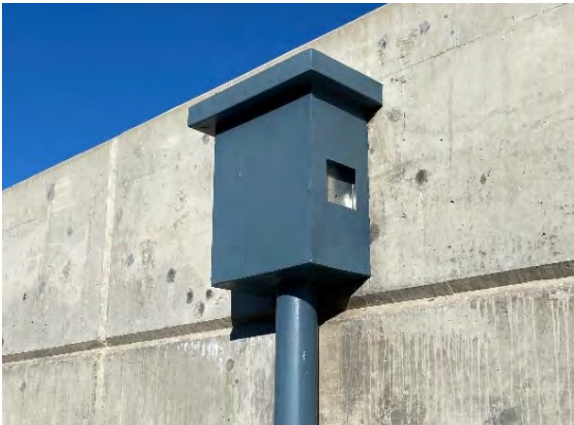
Figure 45- Scupper and Downspout
