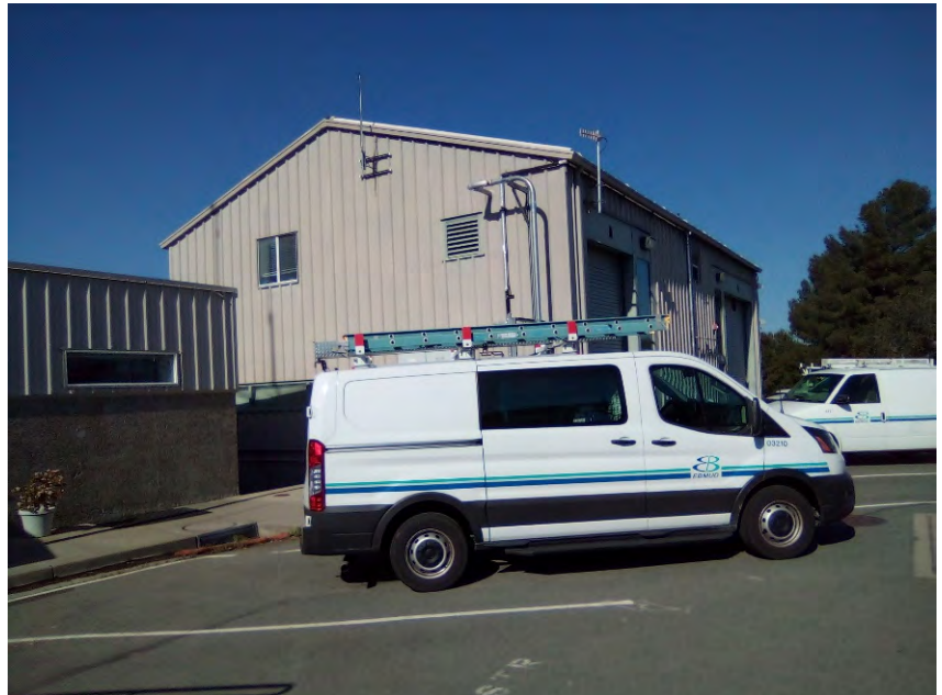
Photo 6: View of the electrical and instrument control building, as viewed from the southeast.
