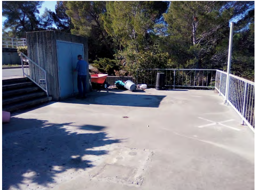
Photo 14: View of the old chemical tank pad, as viewed from the northeast.
