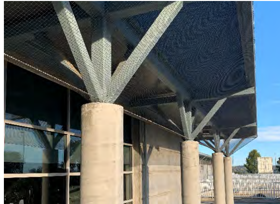
Figure 27- Steel Framed Canopy
