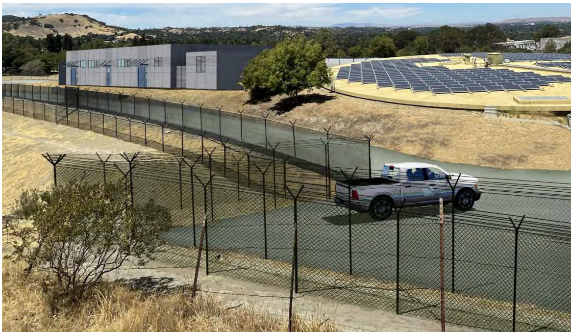
Figure 49- View 1_After Construction
