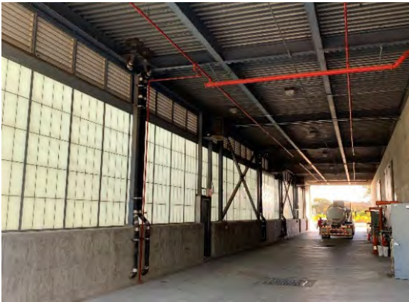
Figure 24- Metal Canopy at Chemical Storage Building
