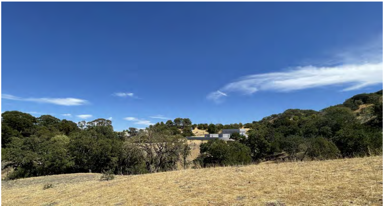
Figure 59 - View 5_After Construction
