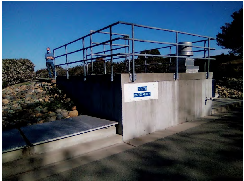
Photo 2: View of the south rapid mix structure, as viewed from the south.
