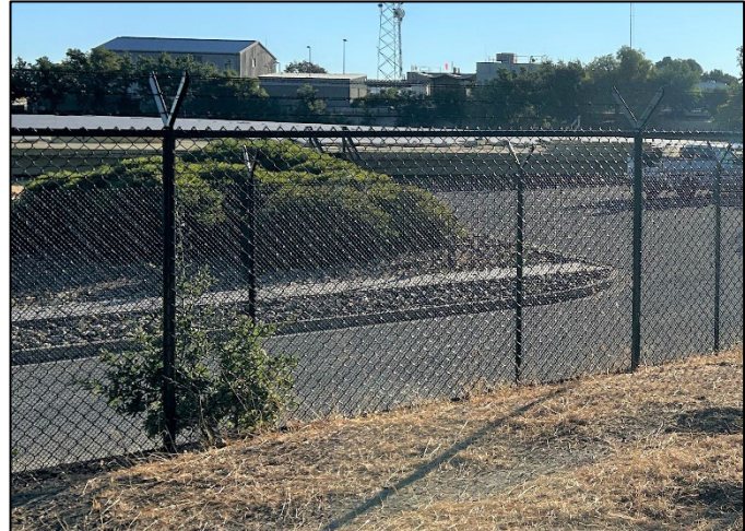
Figure 2-10: Security Fence
