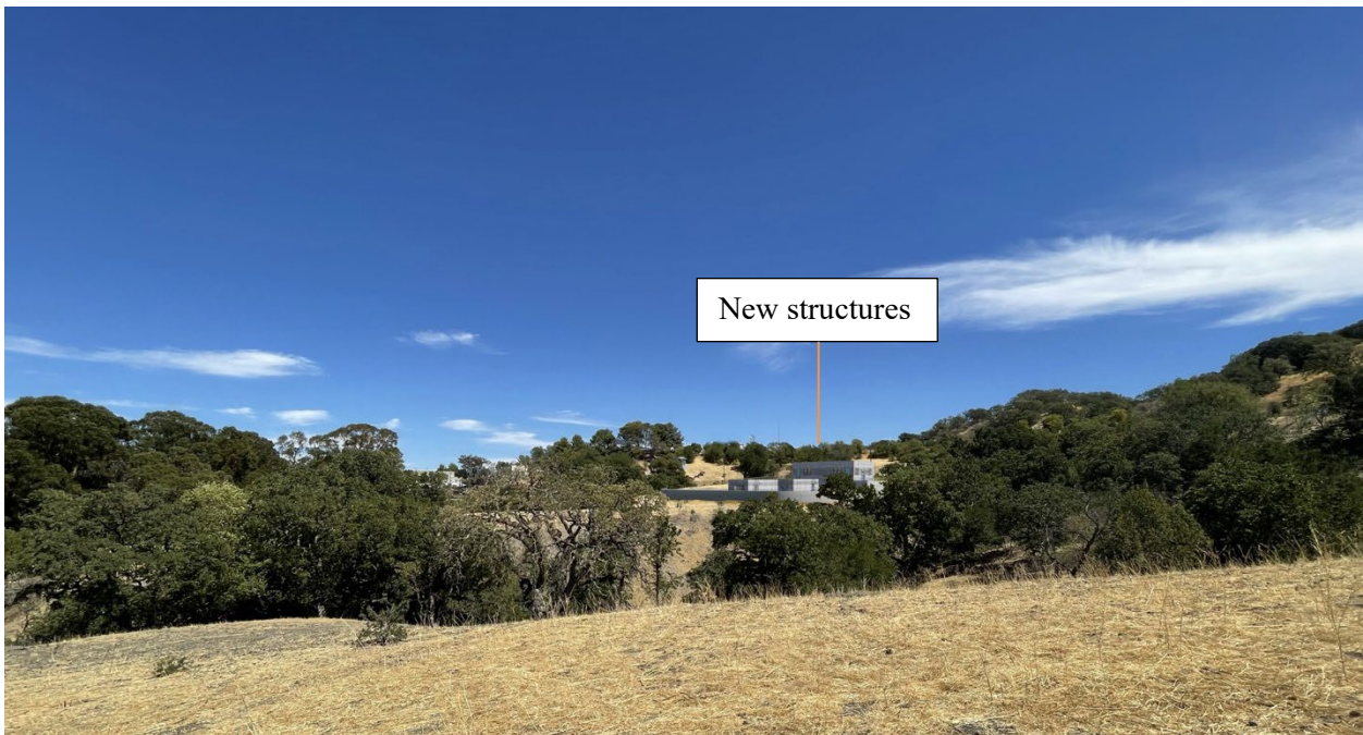
After Construction - Gravity Thickeners, Thickened Solids Pumping Plant, and Solids Dewatering Building partially visible
