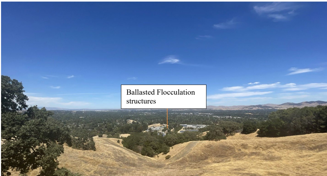
After Construction – Ballasted Flocculation Structures partially visible
