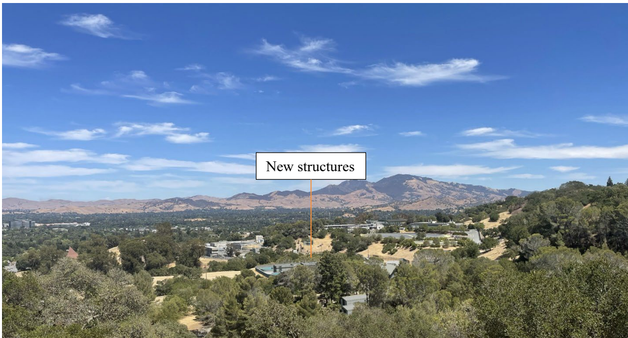
After Construction - Consolidated Maintenance Building, Pre-Ozone Pumping Plant, Thickened Solids Pumping Plant, and Gravity Thickeners partially visible
