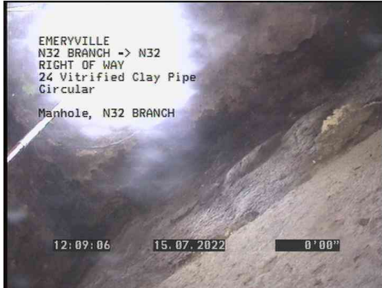
1, 00:00:25, 0.00ft Manhole / N32 BRANCH
