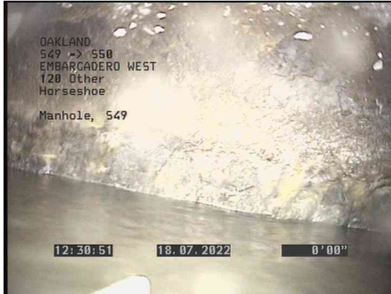
1, 00:00:00, 0.00ft Manhole / S49
