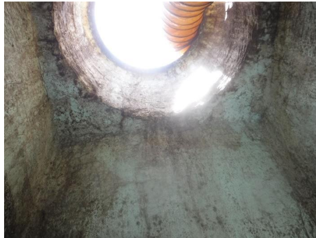
Photo 3-27. MH A47. Upper section of manhole, coating in good condition.
