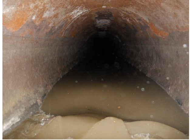
Photo S16 – 2. Upstream pipe S16
