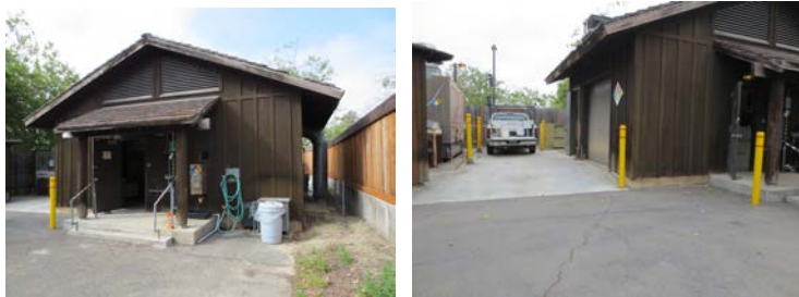
Pump Station M Photos
