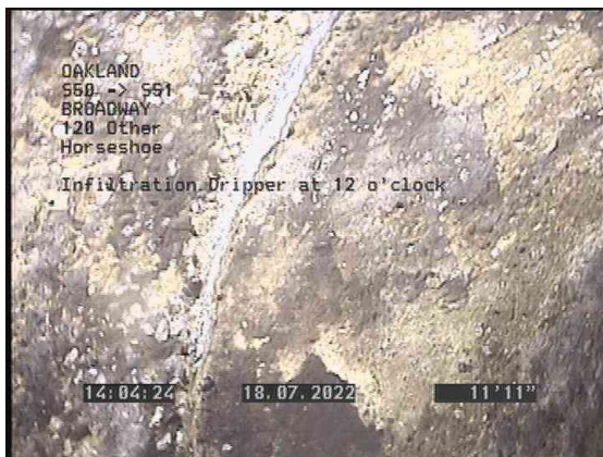
5, 00:02:52, 11.92ft Infiltration Drifter at 12 o'clock
