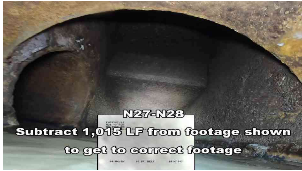
1, 00:00:00, 0.00ft Manhole / N27
