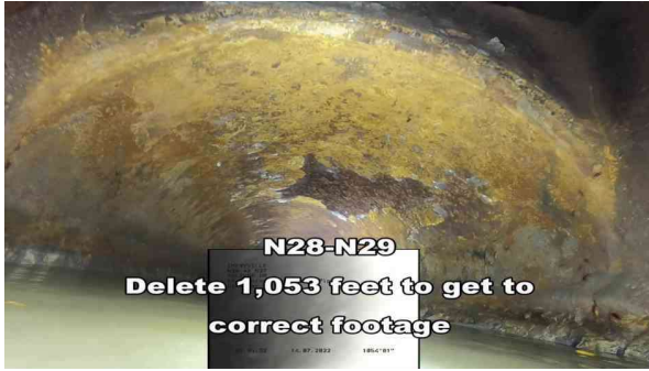
1, 00:00:00, 0.00ft Manhole / N28
