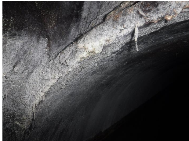
Photo 3-33. MH A48. Lower section of manhole, coating in good condition.
