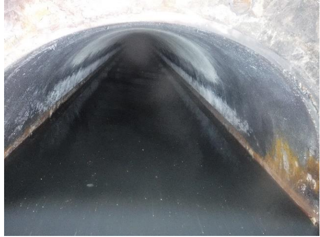
Photo A32 - 2. Upstream pipe, no visible aggregate or exposed rebar.
