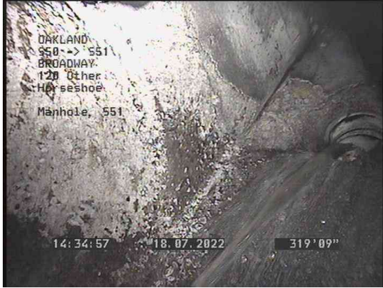
7, 00:33:25, 319.73ft Manhole / S51
