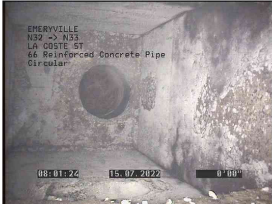
1, 00:00:00, 0.00ft Manhole / N32
