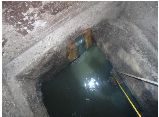
Photo N19-4. Manhole walls and bench, exposed aggregate on surfaces.
