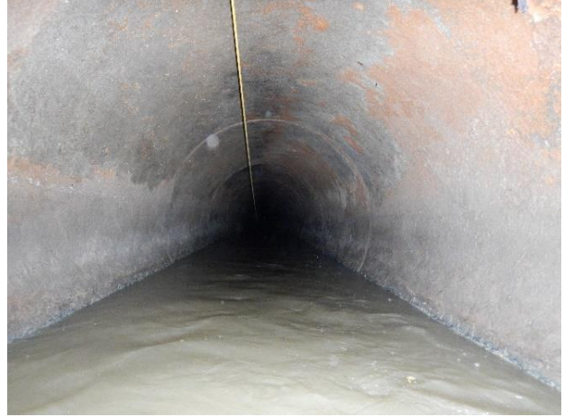
Photo S14 - 2. Upstream pipe.
