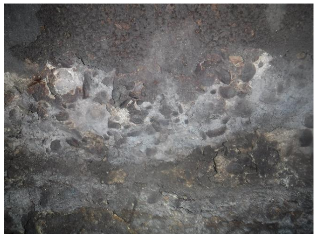
Photo S50 - 6. Large aggregate exposed on upper bench wall.
