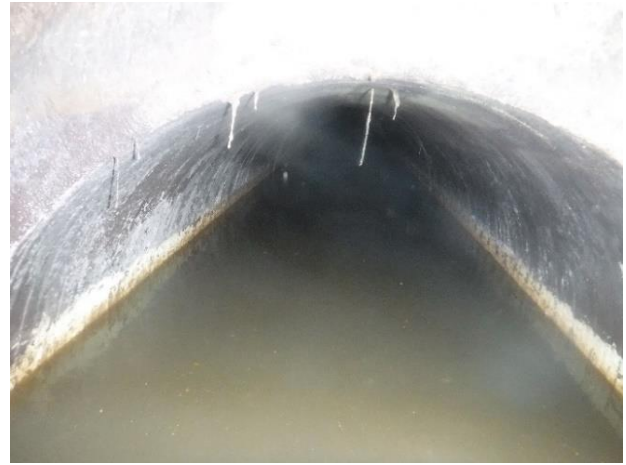
Photo A47 - 2. Upstream pipe, no visible aggregate or exposed reinforcement.
