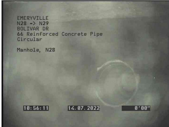
1, 00:00:00, 0.00ft Manhole / N28
