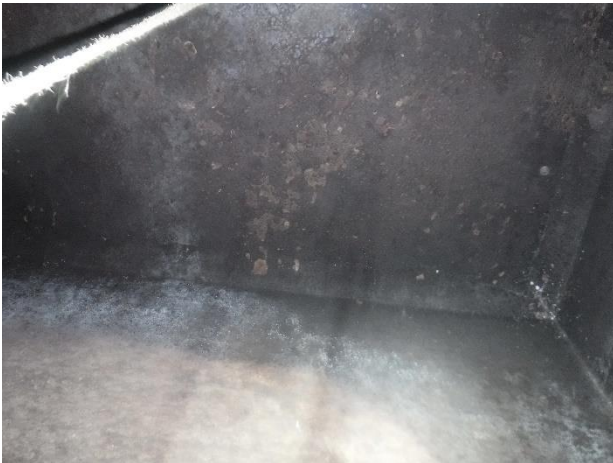
Photo N19-3. Manhole ceiling in good condition.
