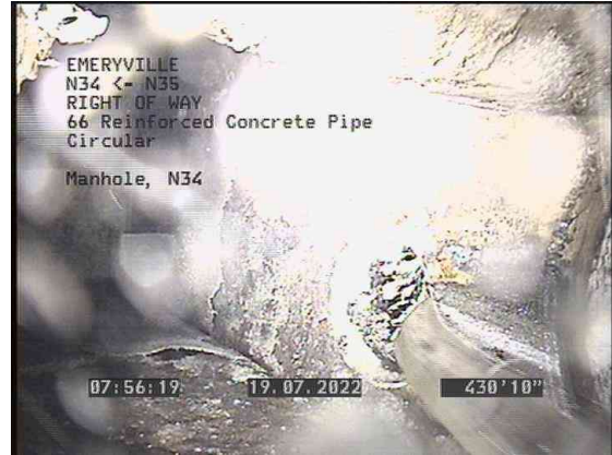
14, 00:12:14, 430.85ft Manhole / N34
