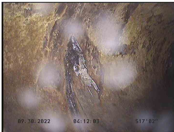
11, 00:20:59, 517.17ft Deposits Attached Encrustation, 5% of cross sectional area from 10 o'clock to 11 o'clock
