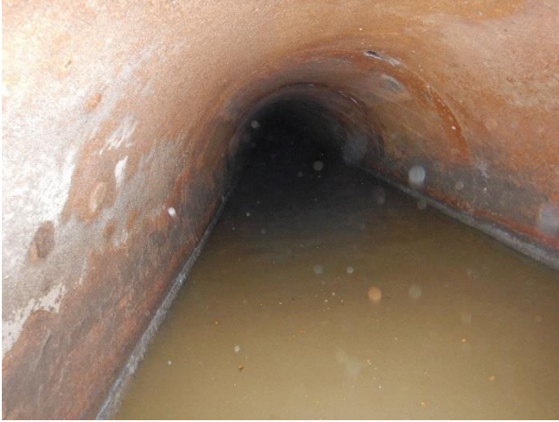
Photo S39 - 1. Upstream pipe.
