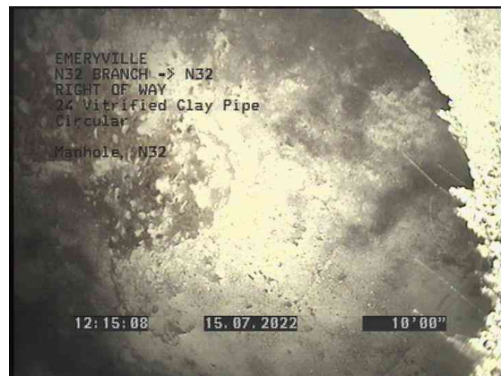
6, 00:05:57, 10.02ft Manhole / N32
