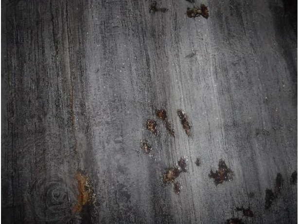
Photo 3-28. MH A48. Upper section of manhole, coating in good condition.
