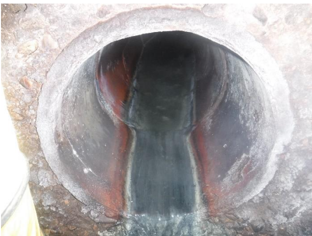
Photo S50 - 5. Lateral drop inlet pipe.
