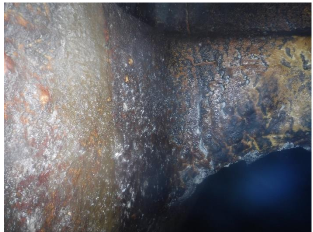
Photo A34 - 6. Manhole condition above upstream pipe.
