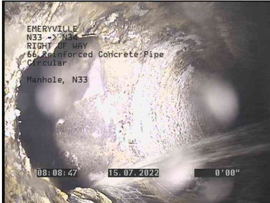
1, 00:00:00, 0.00ft Manhole / N33
