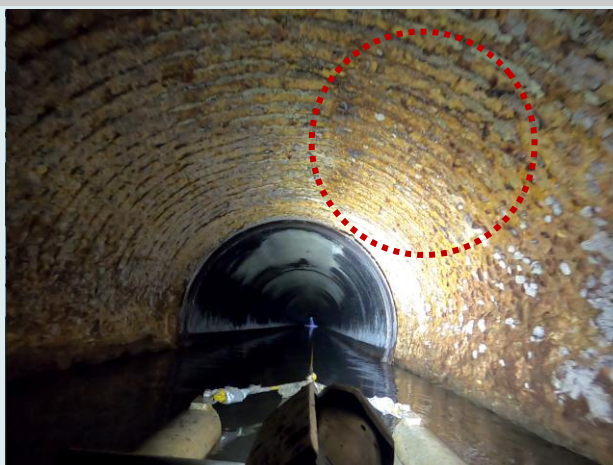
Photo 3-9. Wetness from 1:00 to 3:00 at 550 feet from A39; peaks and valleys between bars
