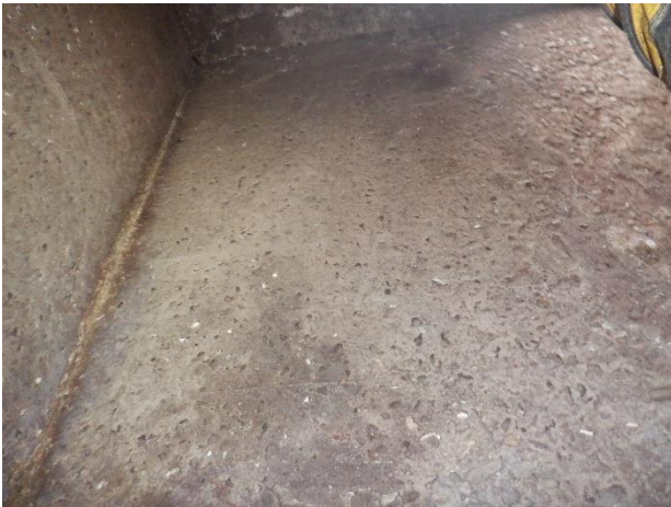
Photo N26 - 5. Manhole wall near upstream, fine exposed aggregate on surface.
