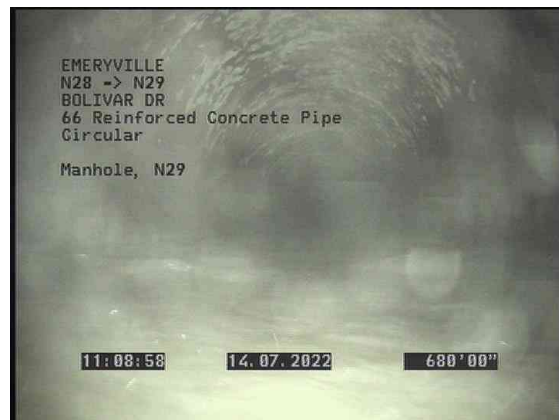
24, 00:15:34, 680.03ft Manhole / N29
