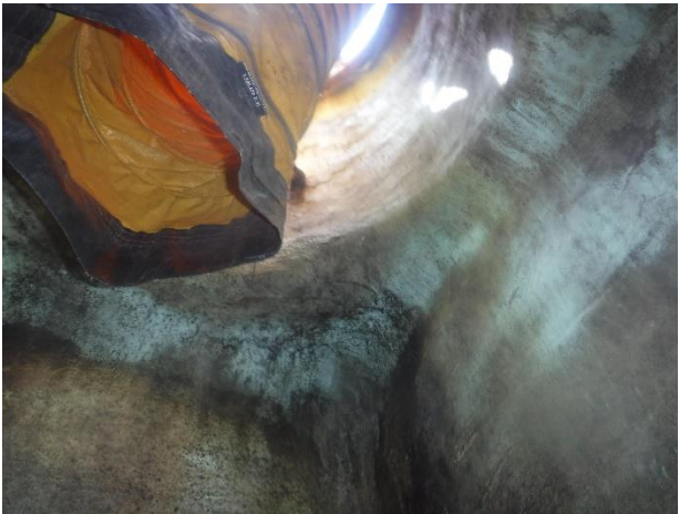
Photo 3-26. MH A47. Upper section of manhole, coating in good condition.
