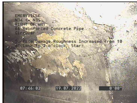
4, 00:01:57, 0.00ft Surface Damage Roughness Increased from 10 o'clock to 2 o'clock, Start
