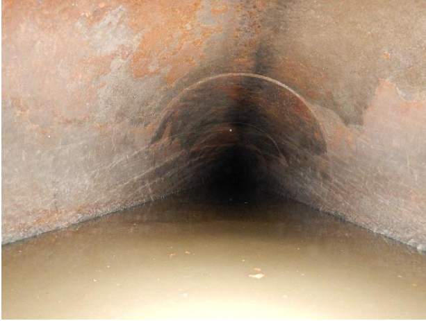
Photo S14 - 1. Downstream pipe.
