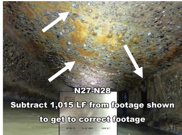
Photo 5-2. VANDA Level 4 exposed reinforcing steel in segment N27N281; 15 feet downstream of N27; infiltration at wall/ceiling interface
