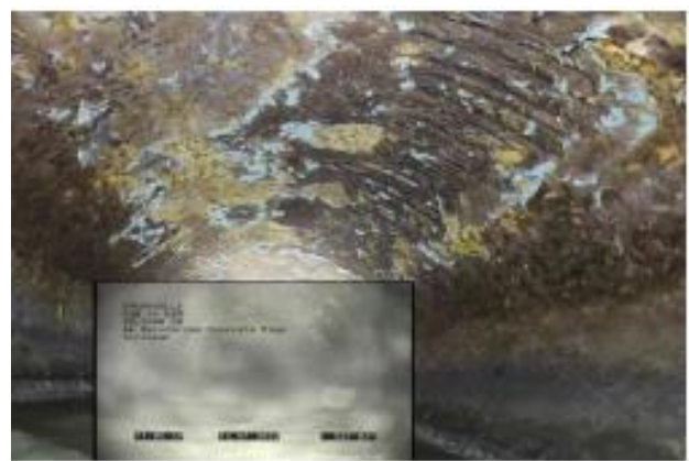
Photo 5-2. VANDA Level 4 exposed reinforcing steel in segment N27N281; 15 feet downstream of N27; infiltration at wall/ceiling interface
