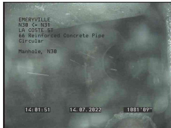
4, 00:38:35, 1081.72ft Manhole / N30
