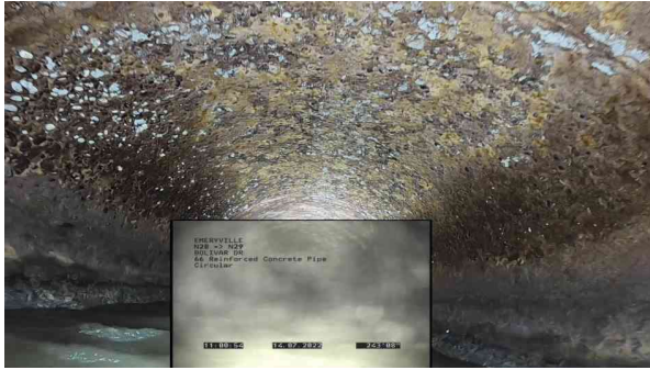
13, 00:05:32, 243.50ft Surface Damage Aggregate Projecting from 10 o'clock to 11 o'clock, within 8 inch, Start
