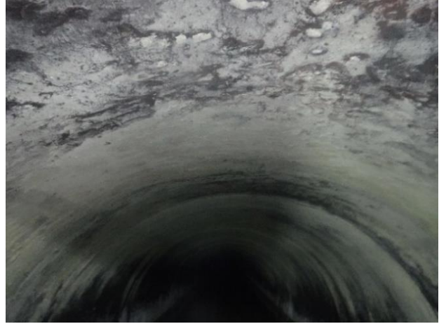
Photo A37 - 2. Upstream pipe, no exposed rebar or aggregate.
