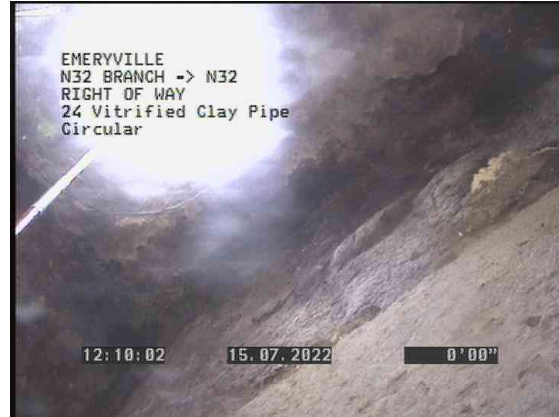
2, 00:00:25, 0.00ft Manhole / N32 BRANCH
