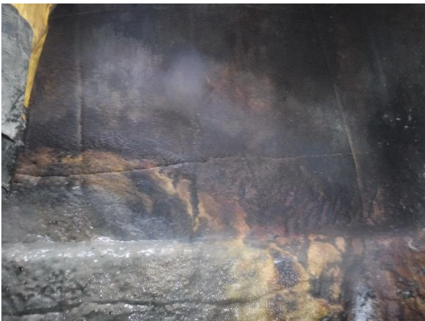
Photo A34 - 5. Manhole conditions on upper bench.
