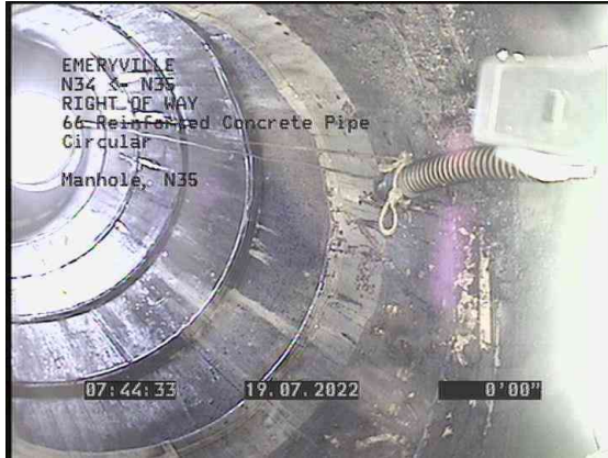
1, 00:00:00, 0.00ft Manhole / N35
