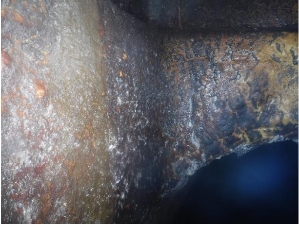
Photo 3-34. MH A34. Bench section of manhole, coating in good condition.
