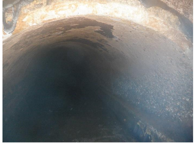
Photo S38 - 2. Upstream pipe.
