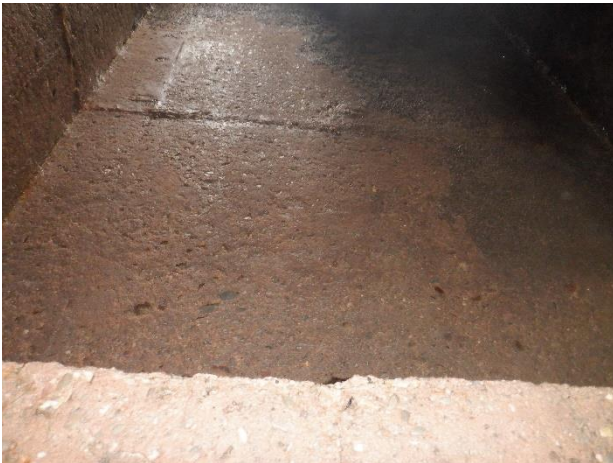
Photo N31 - 5. Manhole wall, in good condition.
