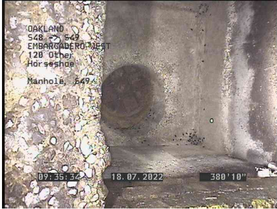
7, 00:08:00, 380.85ft Manhole / S49
