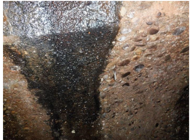
Photo N31 - 6. Manhole bench, fine exposed aggregate below drop inlet.
