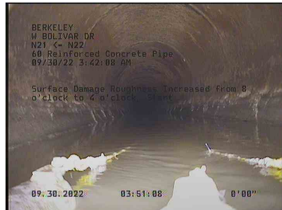
4, 00:01:25, 0.00ft Surface Damage Roughness Increased from 8 o'clock to 4 o'clock, Start
