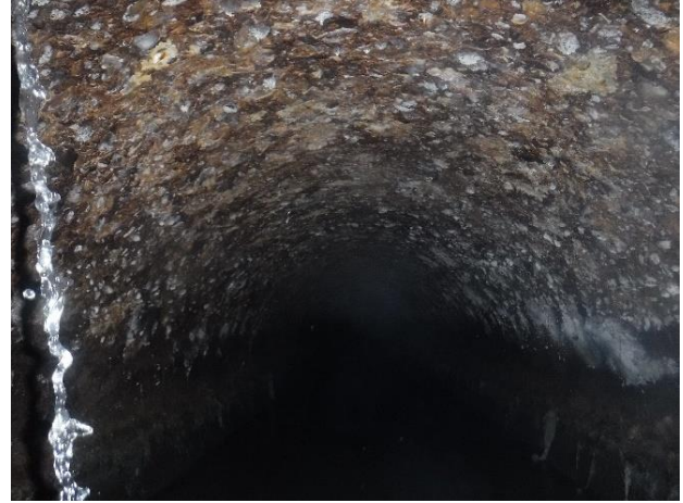
Photo S49 - 2. Upstream pipe.
