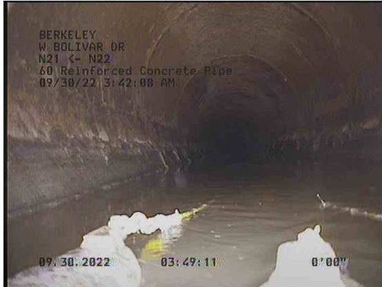
1, 00:00:22, 0.00ft Manhole / N22
