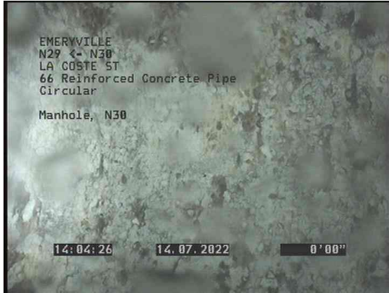
1, 00:00:25, 0.00ft Manhole / N30
