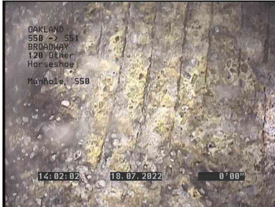
1, 00:00:30, 0.00ft Manhole / S50
