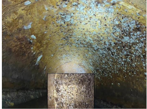
Photo 5-12. Typical VANDA Level 3 with yellowish concrete/exposed aggregate; N26N271 shown
