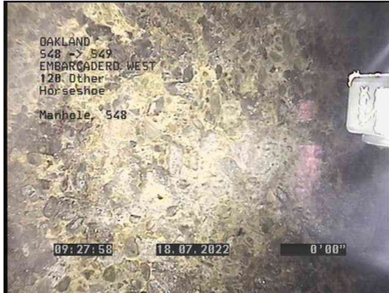
1, 00:00:00, 0.00ft Manhole / S48
