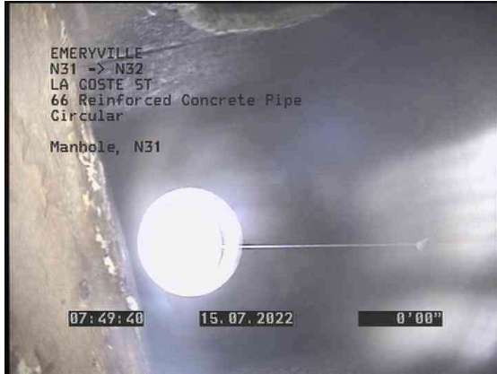
1, 00:00:47, 0.00ft Manhole / N31
