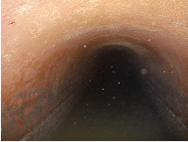
Photo S38 - 1. Downstream pipe.
