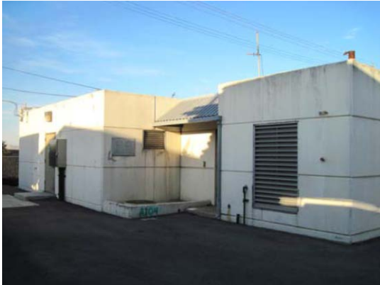
Pump Station A Bldg Photo
