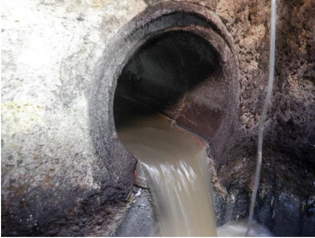
Photo S15 - 1. Lateral inlet, spraying into interceptor pipe opening.
