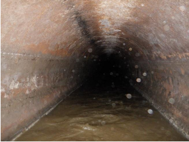
Photo S16 – 1. Downstream pipe S16.
