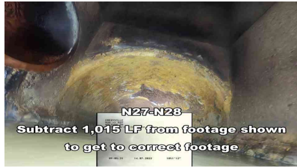
10, 00:00:37, 37.00ft Manhole / N28
