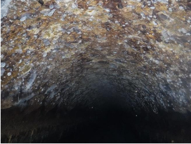
Photo S49 - 1. Downstream pipe.
