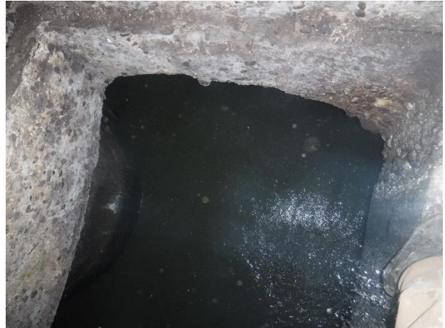
Photo S50 - 2. Interceptor pipe as seen from the manhole structure.
