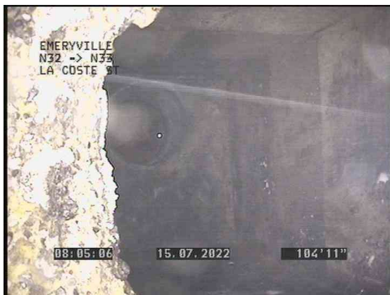
5, 00:04:13, 104.91ft Manhole / N33
