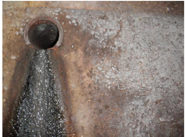
Photo N26 - 6. Fine exposed aggregate around drop inlet on bench.
