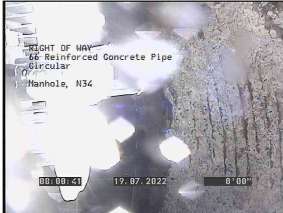
1, 00:00:00, 0.00ft Manhole / N34
