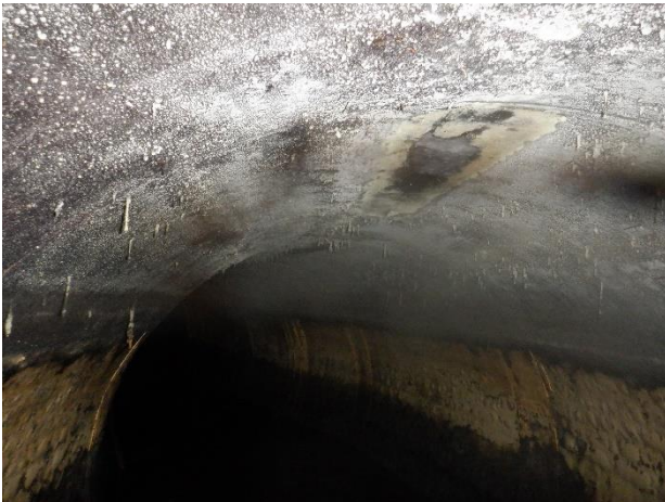
Photo N35 - 3. Lined downstream pipe in good condition
