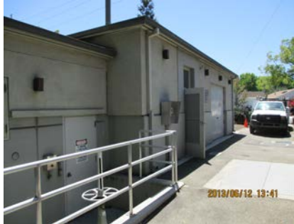
Pump Station B Site Photo
