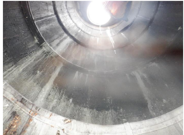
Photo N35 - 4. PVC lining in manhole in good condition.
