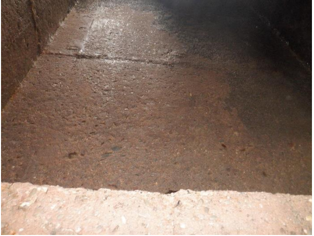
Photo 5-19. MH N31, Manhole walls in good condition.
