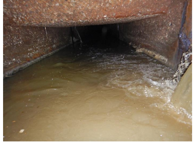
Photo S39 - 2. Downstream pipe.
