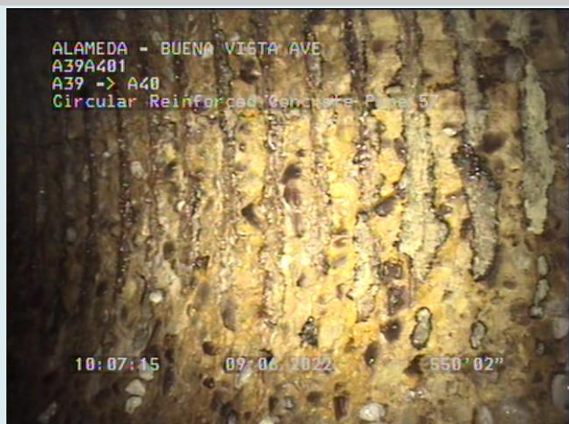
Photo 3-10. Close-up of wetness from 1:00 to 3:00 at 550 feet from A39; peaks and valleys between bars
