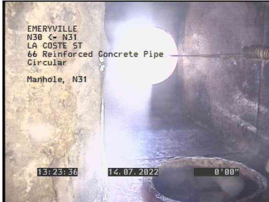
1, 00:00:22, 0.00ft Manhole / N31
