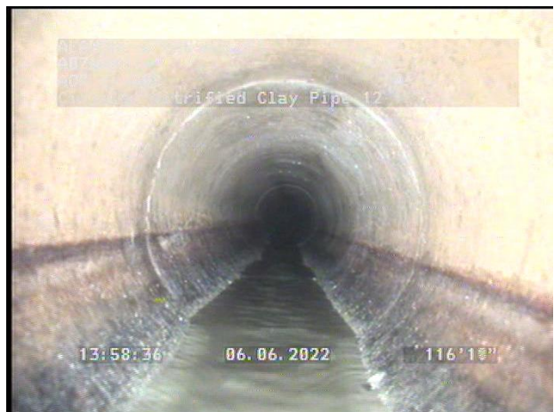
Photo 3-20. Typical VCP surfaces in good condition in majority of alignment
