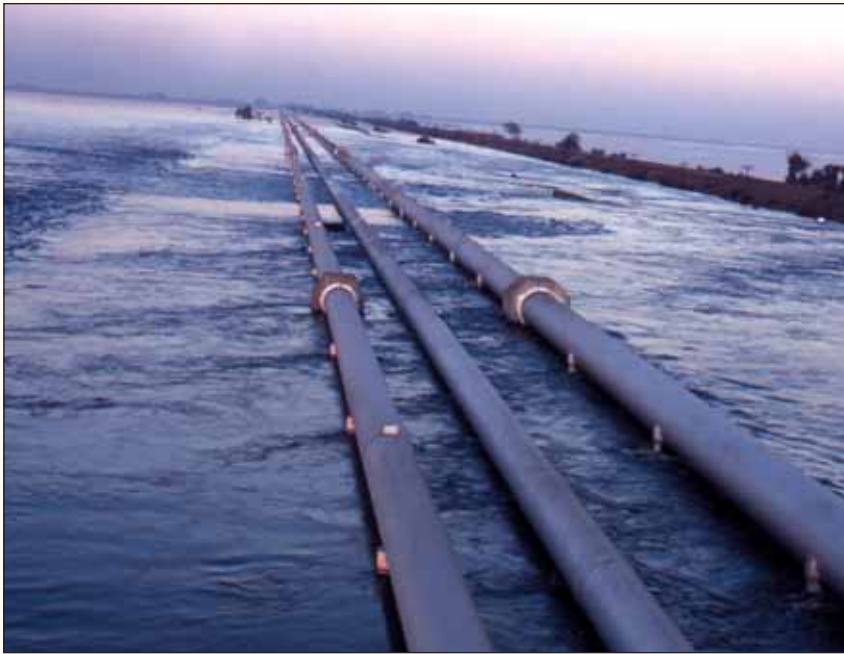
Rising sea levels threaten levees in the Sacramento/San Joaquin River Delta, home to East Bay Municipal Utility District's three primary aqueducts and much of California's water supply. A singular levee breach in 2004, shown here, submerged the district's aqueducts for more than four months.
