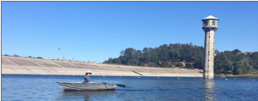
The Project involves designing a retrofit for the Lafayette Reservoir Outlet Tower to address seismic, mechanical and electrical deficiencies. Currently, the structural retrofit alternatives include: 1) adding post-tensioned anchors extending from the operating house down through the walls and into bedrock, and 2) shortening the Tower.
