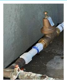
Photo of installed pressure regulator. Must be brass or bronze and installed upstream of entire irrigation system.
