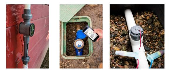
Installed new flow sensor\* (\*various acceptable flow sensors shown as example)
