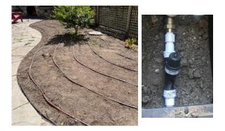
Photos of drip irrigation system, including pressure regulator and filter components, can push mulch aside to show tubing *(if drip irrigation was installed)*
