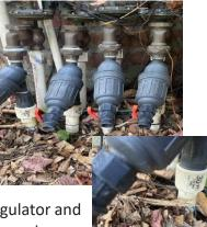
Drip pressure regulator and filter components
