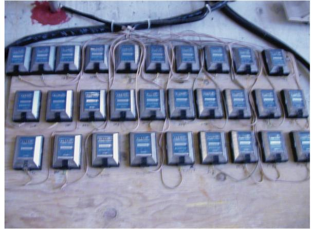
**Figure 1.1 Example of remote registers for submetering**
