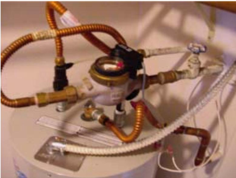
**Figure 1.2 Example of a hot water hybrid meter setup**
