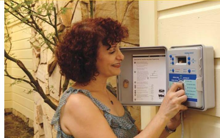
**EBMUD offers financial incentives for a new generation of irrigation controllers that automatically adjust irrigation schedules to weather conditions, preventing watering during rain and applying more water during unexpected hot spells.**
