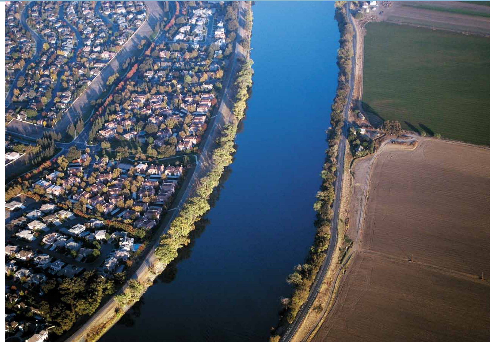
More than 30 years in the making, the Freeport Regional Water Supply Project will draw water in dry years from the Sacramento River at Freeport (above). Featuring art and poetry, the project's intake facility (partial rendering at bottom of page 2) commemorates the river and the importance of water in our daily lives.
