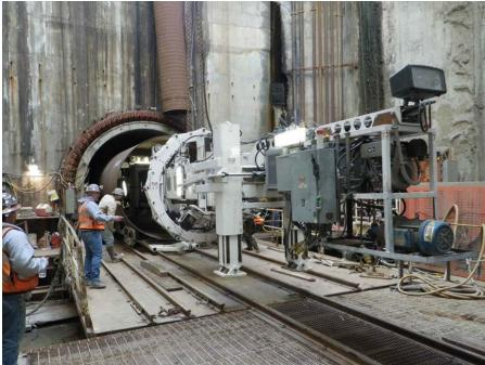
Inserting the Carrier Pipeline into the Tunnel
