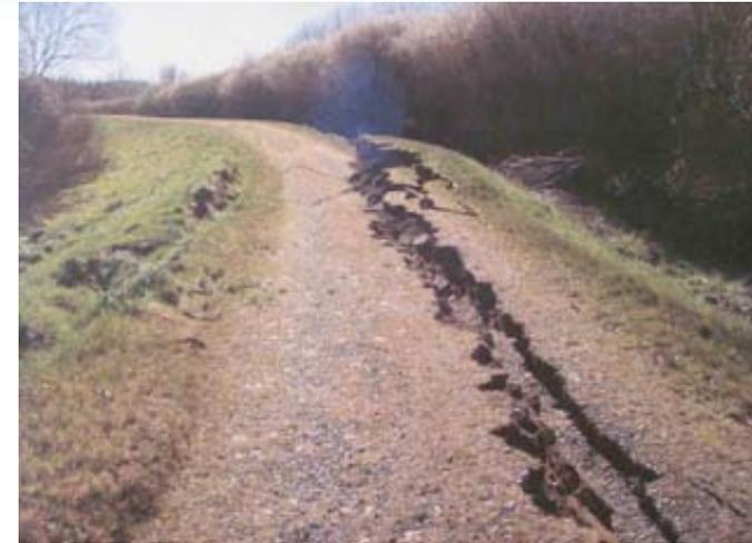
Levee Lateral Spreading Failure in 2011 Christchurch Earthquake (New Zealand)
