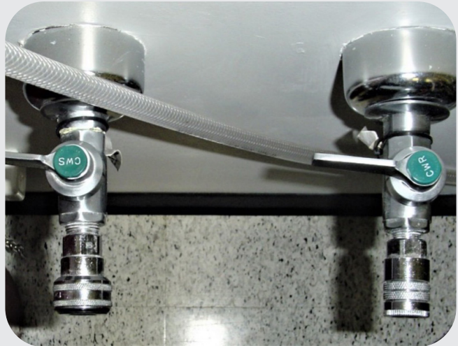
Example of a Laboratory Equipped with a Chilled Water Source and Return
