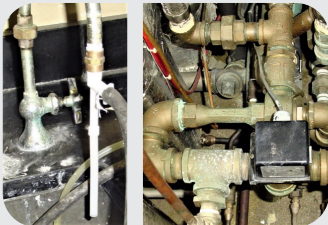
Figure 11-2: Aspirator in Lab and Venturi Vacuum on Sterilizer
