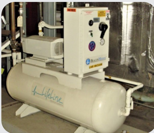
Figure 11-7: Lubricated Rotary Vane Dry Vacuum Pump
