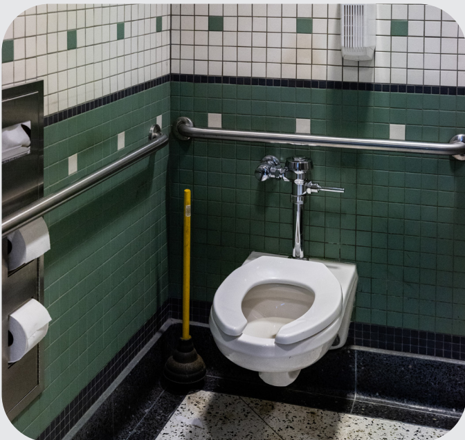
Flush Valve Toilet in a Commercial Bathroom
