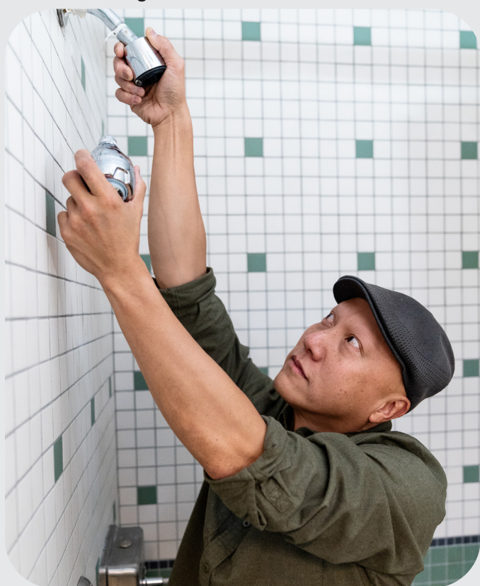
Installing a Water Efficient Showerhead
