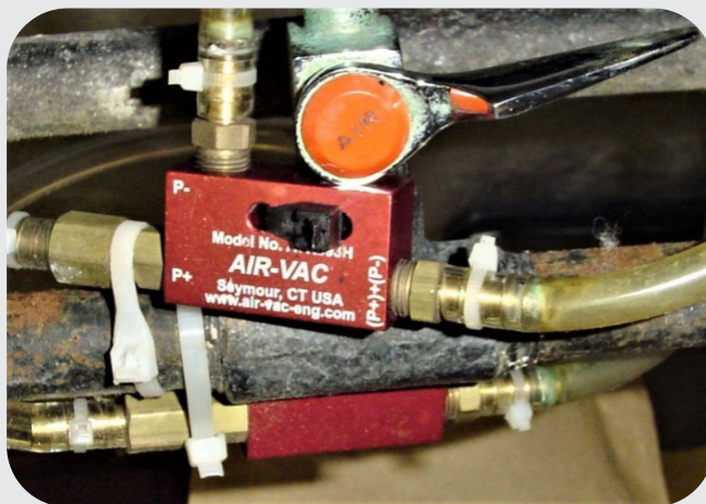
Figure 11-4: Compressed Air Venturi System
