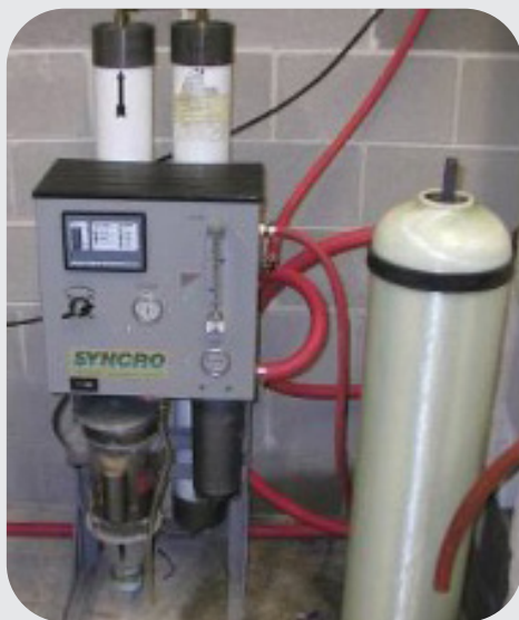
RO Filters at a Car Wash
