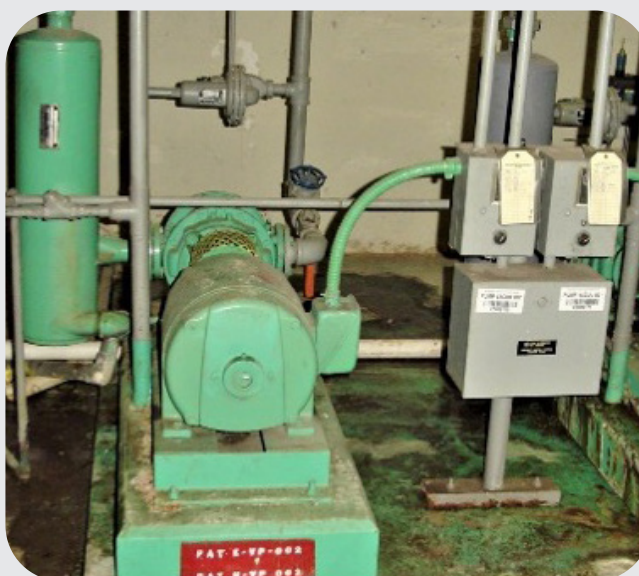
Figure 11-8: Lubricated Rotary Vane Dry Vacuum Pump
