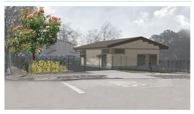
EBMUD selected Concept 2, the Residential Design concept, as the preferred architectural concept for the Fontaine PP building. The concept features beige stucco cladding with contrasting trim over cast-in-place concrete walls, covered by a steel-framed gable roof with brown asphalt shingles. This concept was determined to best meet EBMUD's design objectives and the community's aesthetic preferences.
