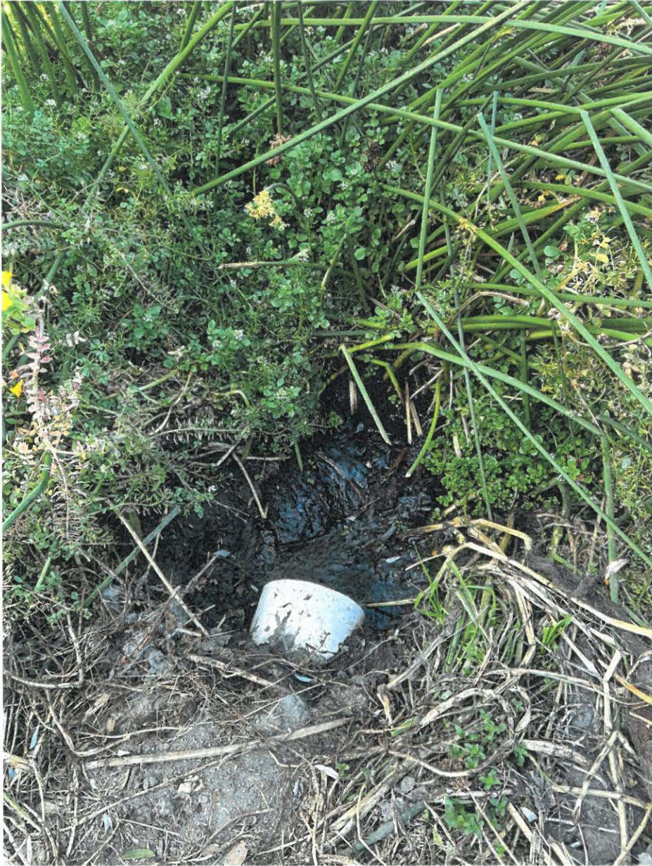
Figure 9. Culvert inlet that connects Baby Bottle Pond with the channel downstream.
