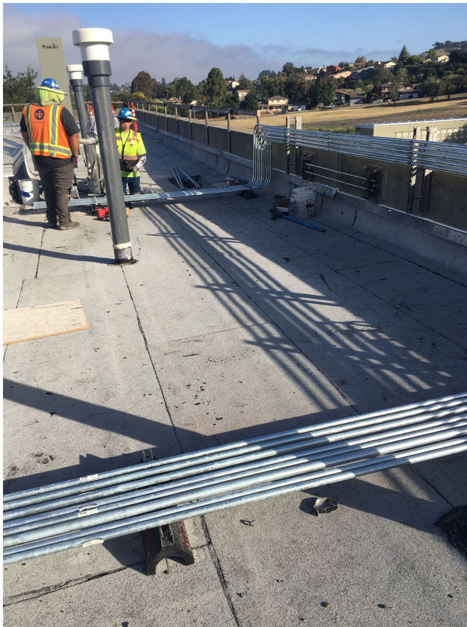
Figure 18 – Sobrante WTP Chemical Building Roof – ongoing work on electrical system for HVAC equipment.
