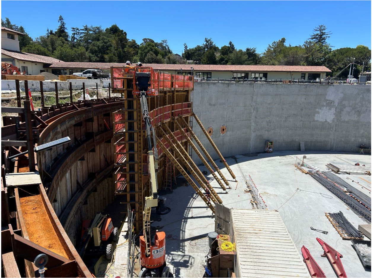
Figure 7 – CCB – Construction of exterior concrete walls.
