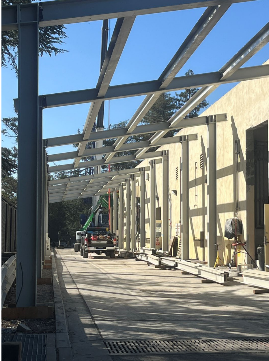
Figure 13 – USL Chemical Building – Installation of new truck unloading area canopy. The canopy will protect the environment by preventing rainwater from mobilizing chemical spills.
