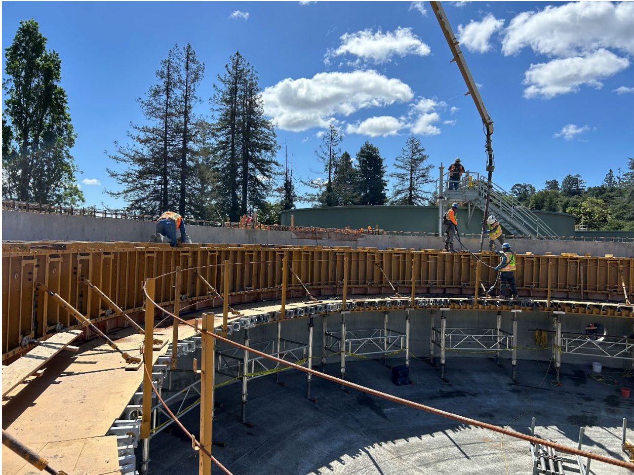
Figure 9 – Gravity Thickener – in progress concrete pour of Gravity Thickener Launde. This gravity thickener will reduce water loss at the WTP by up to 90% by reducing the amount of spent residuals to the sewer system.
