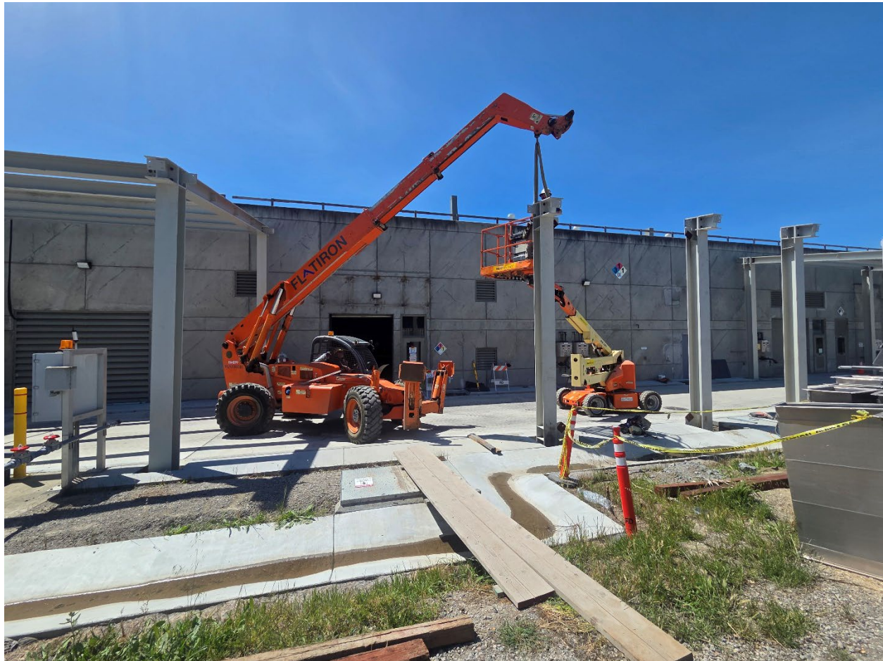
Figure 17 – Sobrante WTP Chemical Building – ongoing installation of new truck unloading area canopy. The canopy will protect the environment by preventing rainwater from mobilizing chemical spills.
