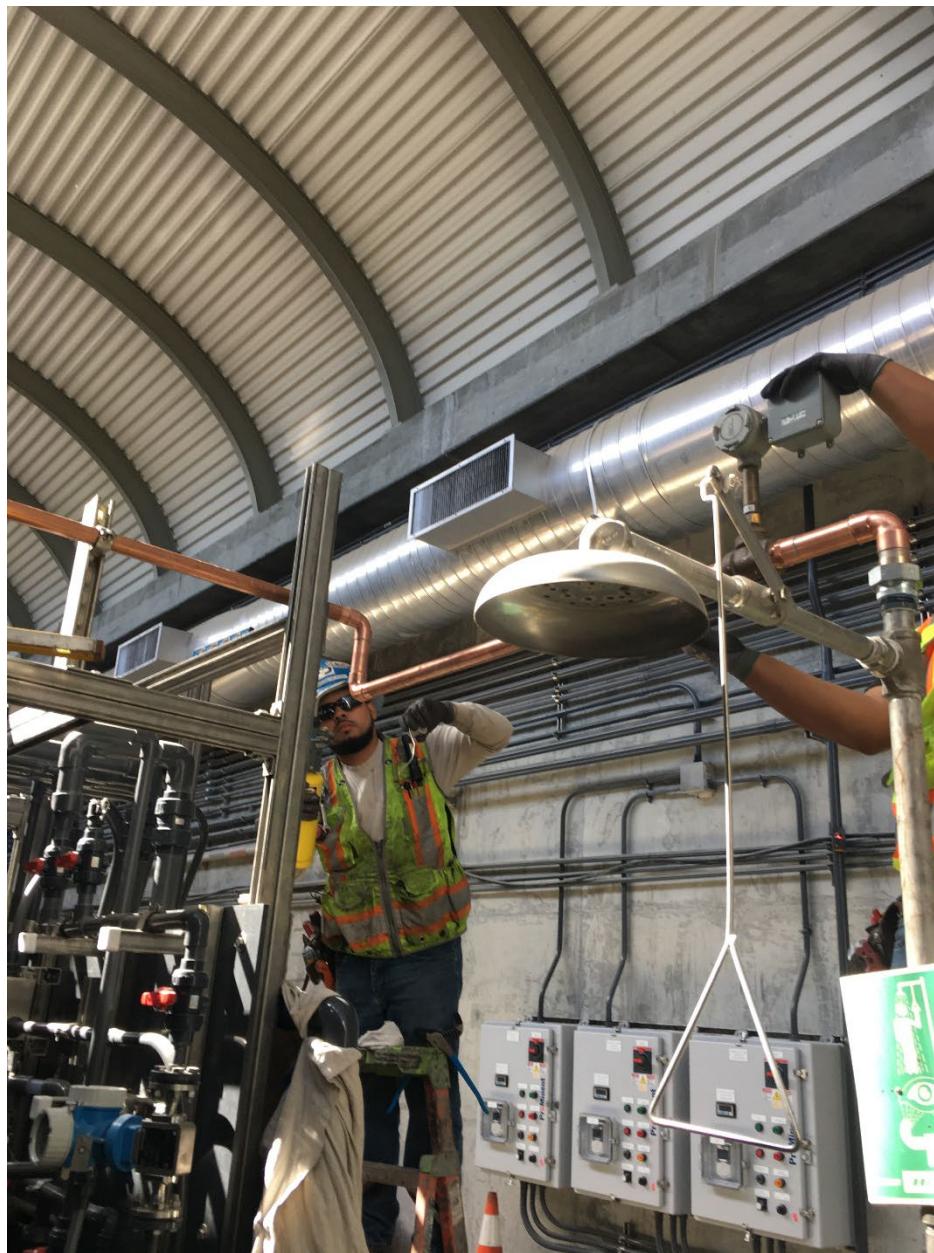
Figure 15 – Sobrante WTP Chemical Building – ongoing work for new chemical feed systems.
