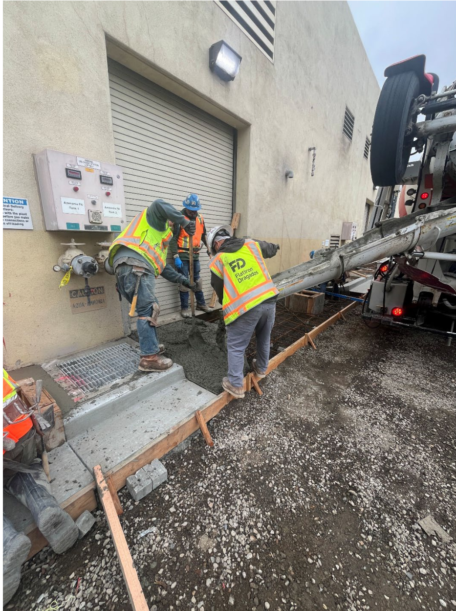
Figure 12 – USL Chemical Building - pour of new canopy footings and sidewalks.
