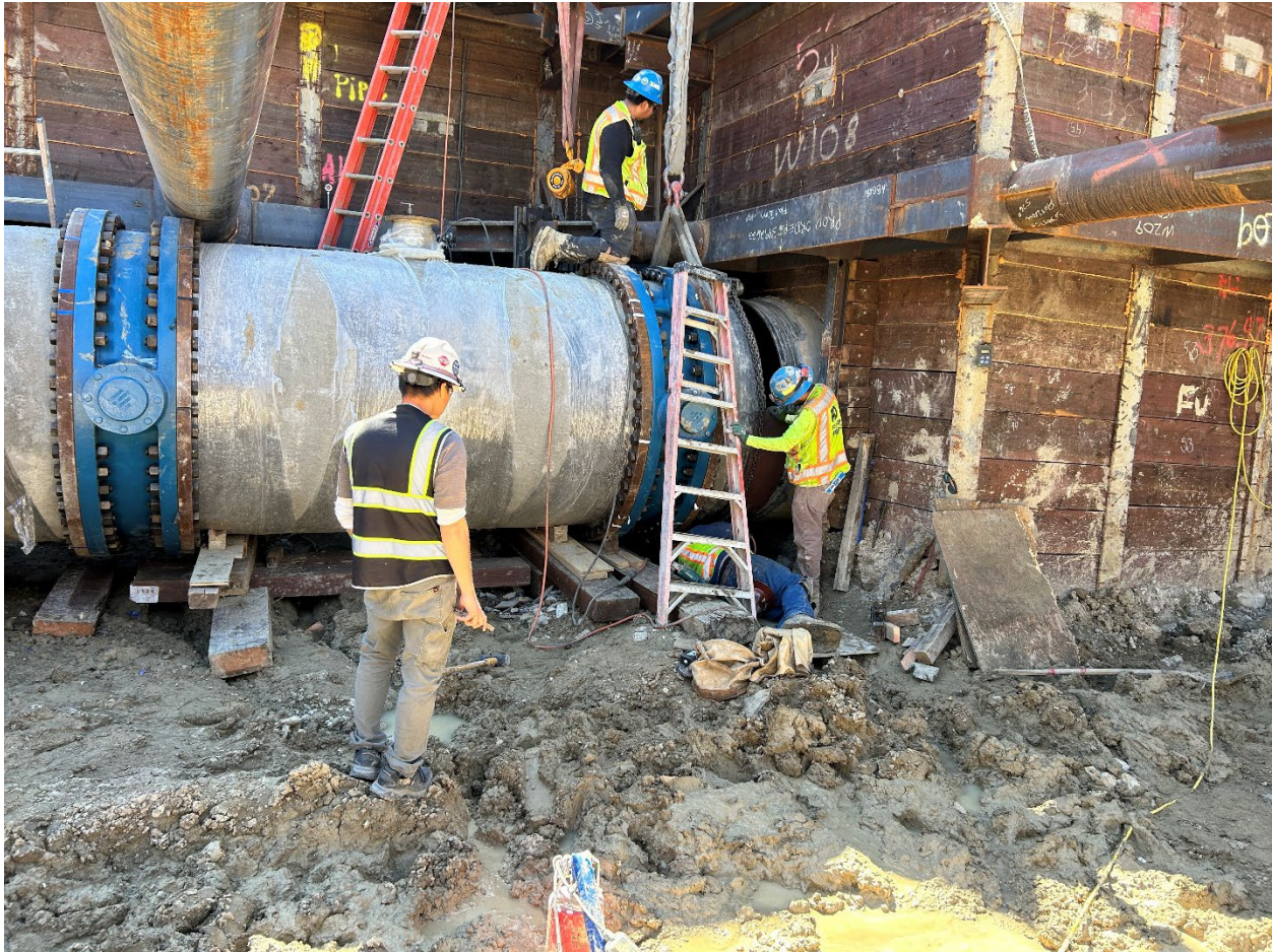
Figure 8 - Combined Filter Effluent - Workers installing the final connection to the Filter effluent. This piping connects the filtered water to the new CCB which will provide primary disinfection for the WTP.
