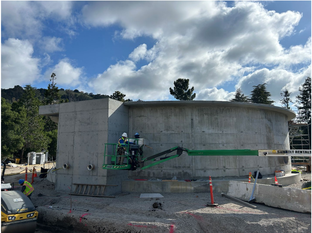
Figure 10 – Gravity Thickener completed structure. This gravity thickener will reduce water loss at the WTP by up to 90% by reducing the amount of spent residuals to the sewer system.
