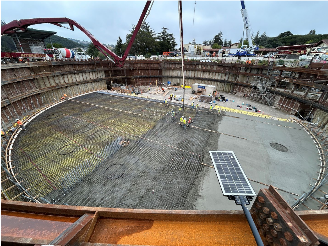
Figure 5 – CCB progress photo of the first half concrete slab pour.
