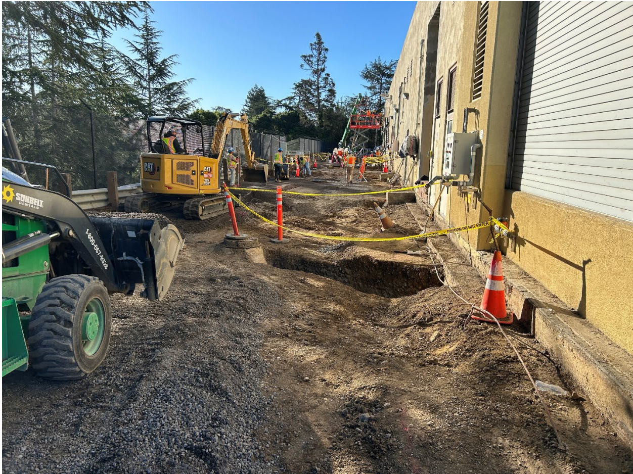
Figure 11 – USL Chemical Building - roadway prep for upcoming canopy work.
