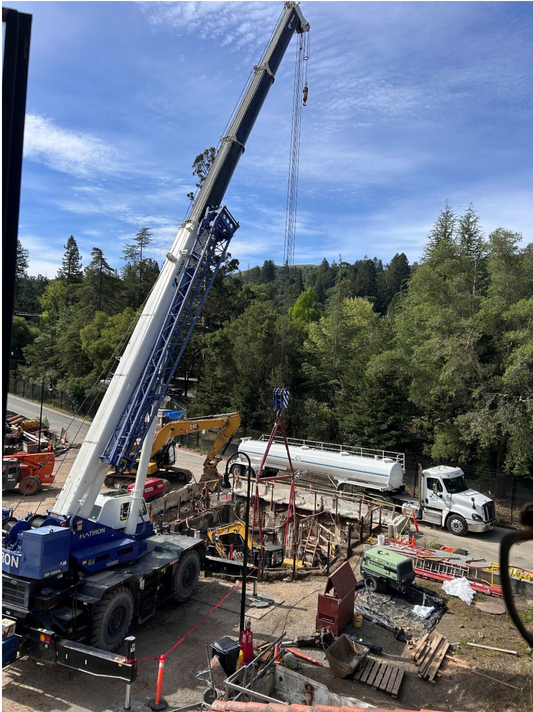
Figure 7 – View of rough terrain crane lifting an excavator from the Effluent 2 excavation to allow the ironworkers to install the next level of excavation bracing. This excavation requires six levels of bracing to get to the bottom of the 40-foot-deep excavation where the piping connections will be made. Note the EBMUD truck adjacent to the excavation showing the challenges of constructing the project at a water treatment plant which operates 24/7.
