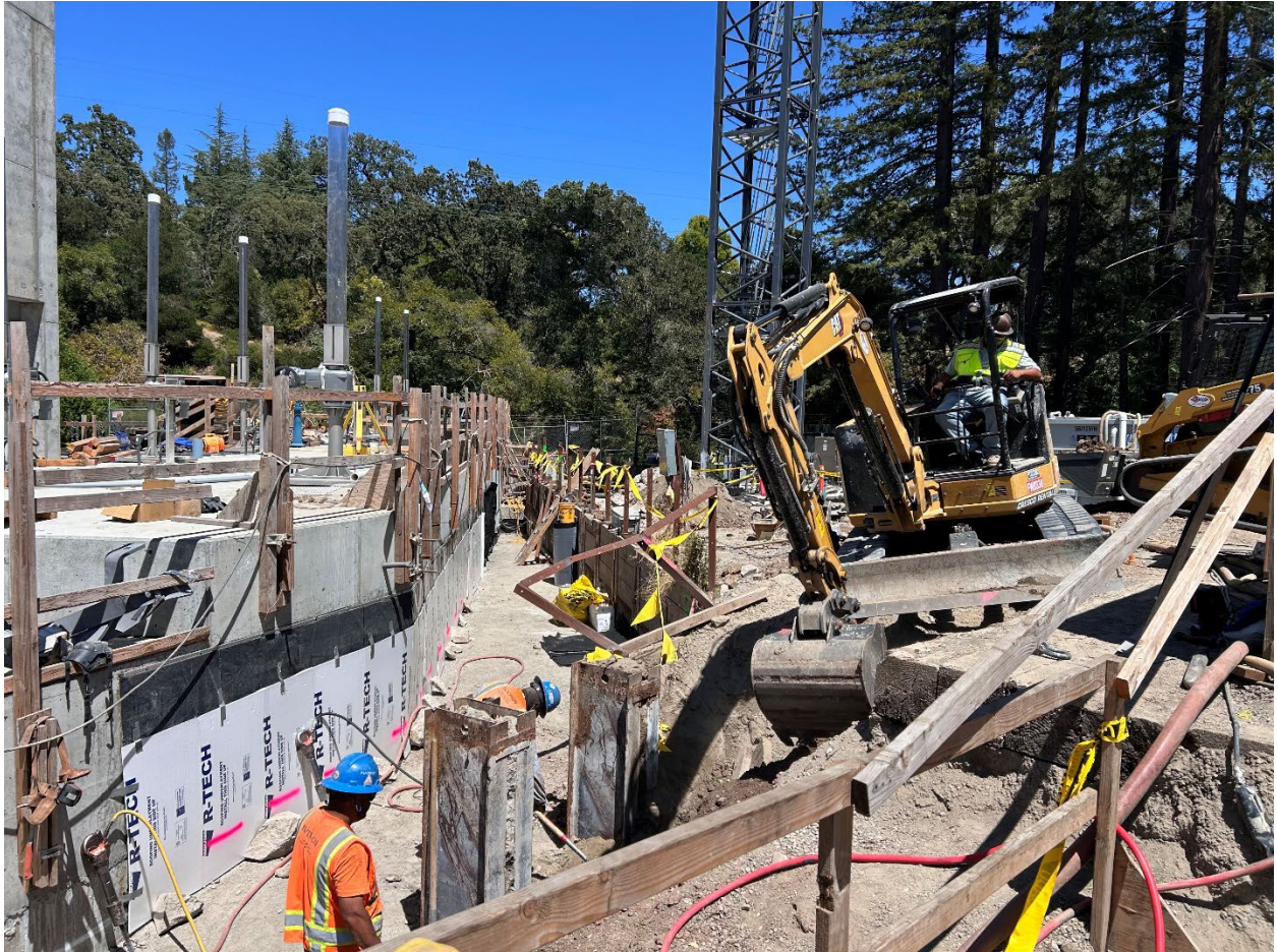
Figure 5 – View of workers excavating the top six feet of the engineered shoring system which supported the 65-foot deep excavation. This part of the shoring system is being removed to allow for installation of underground utilities. The walls of the underground Effluent Weir Structure can be seen behind the workers.
