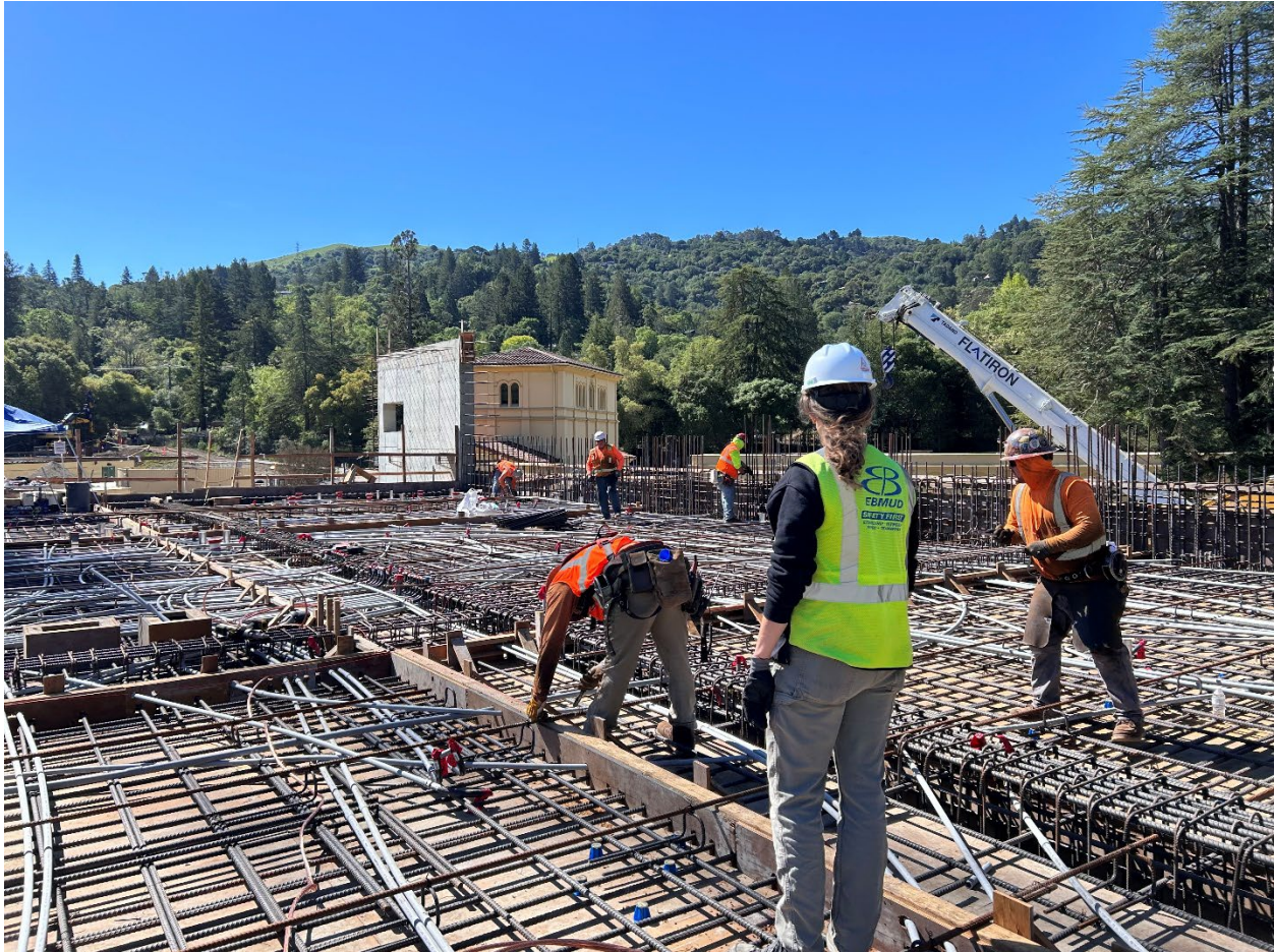
Figure 24 – Engineer inspecting ironworkers as they place the second layer of reinforcing steel for the second floor of the MAUVE Building north end.
