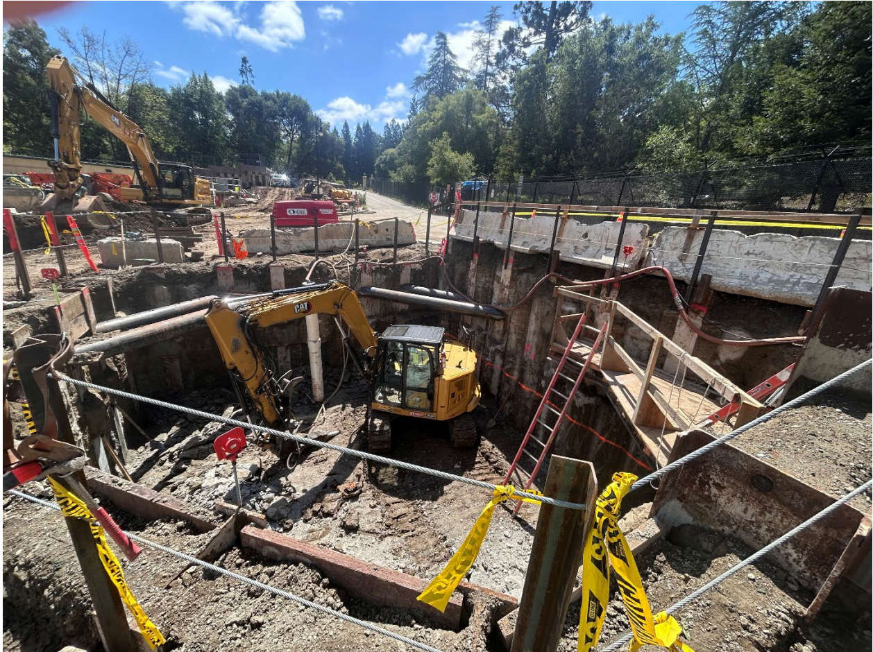
Figure 6 – View of workers beginning the excavation of the Effluent 2 engineered shoring system. The excavation is where the project will make the final piping connection to allow the water to flow from the existing water treatment plant to the new part of the plant.
