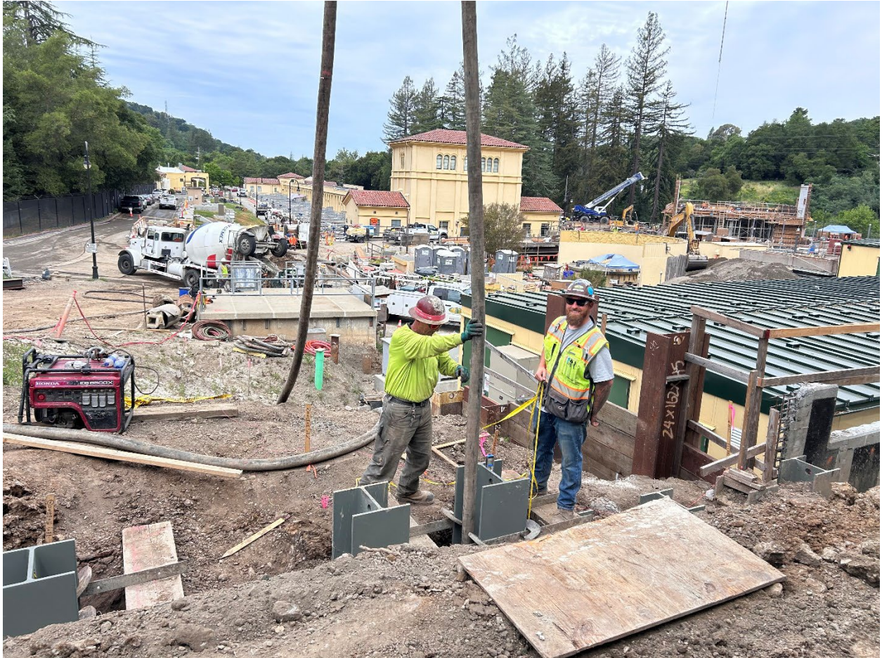
Figure 12 – Closeup view of carpenters placing concrete around underground beams as part of the retaining walls which will support the hillside during excavation.
