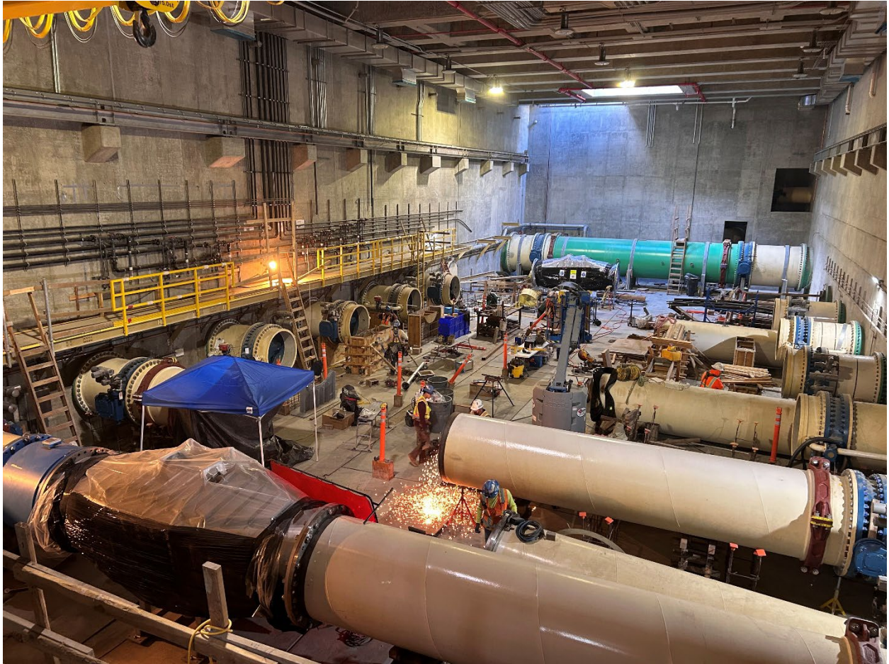
Figure 35 – Pipefitters installing connecting piping to the first UV disinfection vessel in the UV Room.
