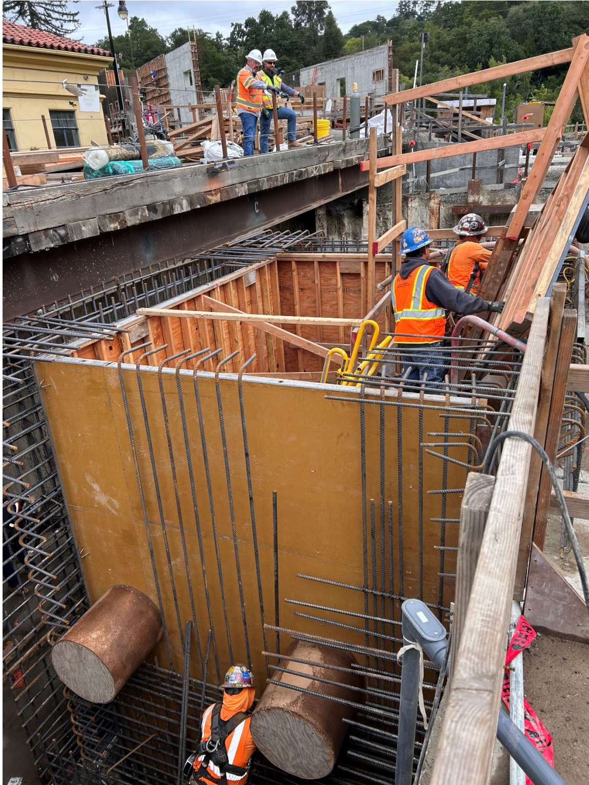
Figure 17 – View of the ironworkers installing rebar for the final wall segments for the underground Effluent 1 Valve Vault.
