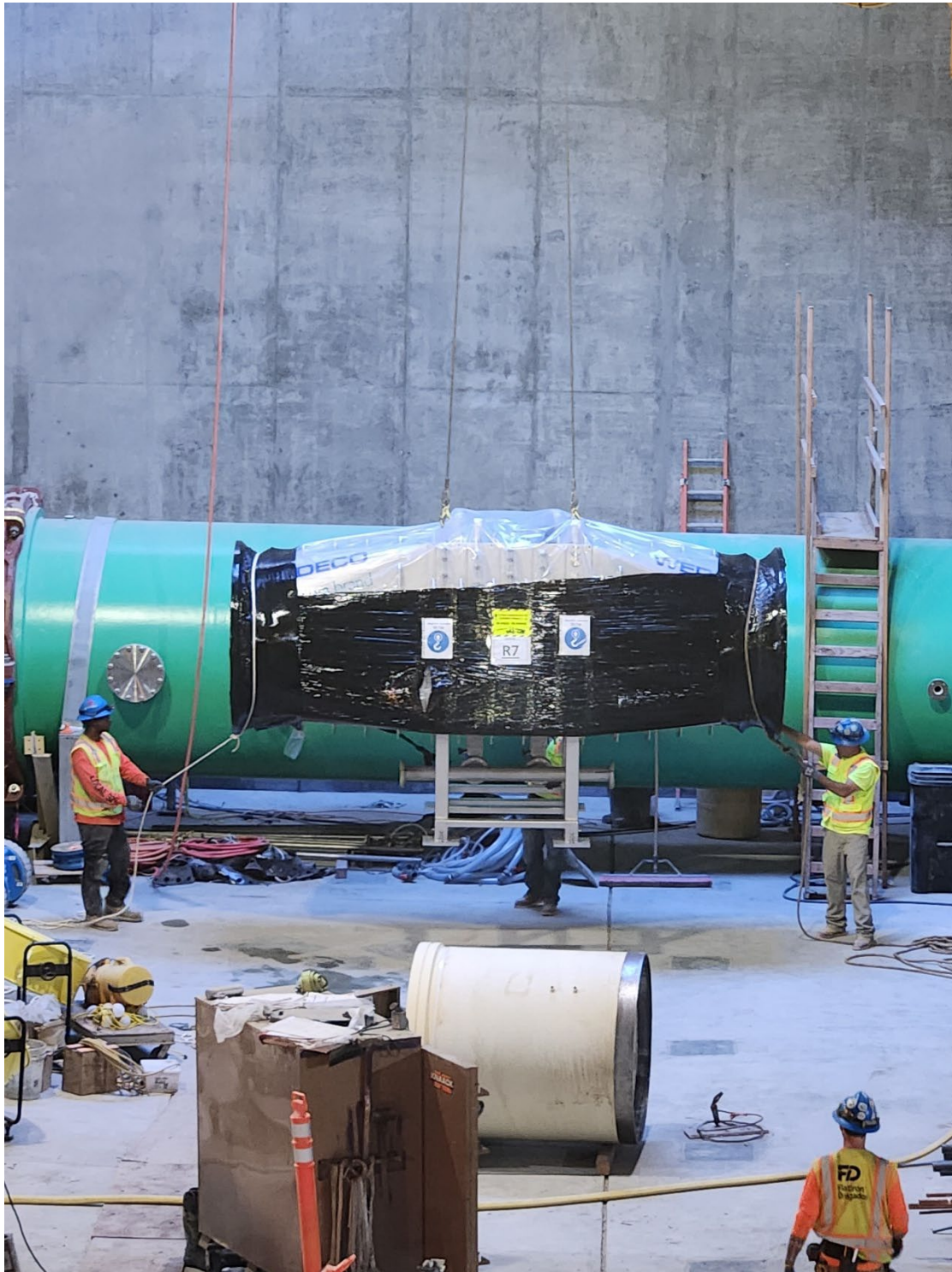
Figure 34 – Closeup view of crane lowering first UV disinfection vessel onto the floor of the UV Room. The access hatch in the first floor of the MAUVE Building is above the workers. The 84-inch green bypass piping can be seen in the background.
