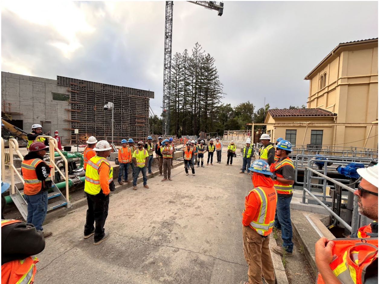
Figure 18 – Workers gather for the safety briefing each day before work begins in the MAUVE Building. At the peak of construction, up to 14 specialty subcontractors will be working on the finishes in this building.
