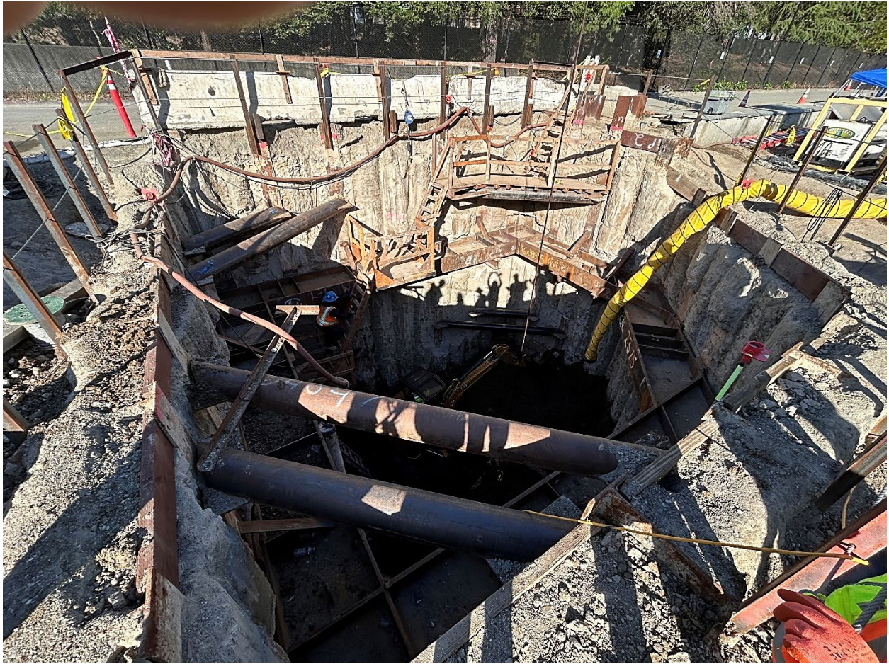
Figure 8 – View looking down into the Effluent 2 excavation with the multiple layers of bracing supporting the excavation walls and adjacent roadway.
