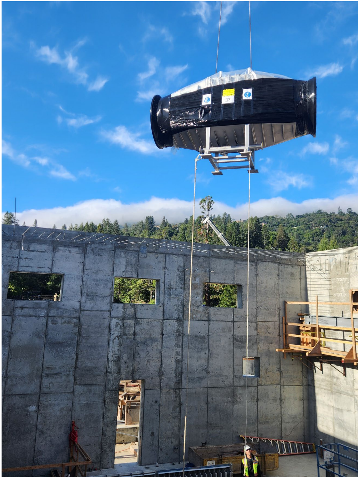
Figure 32 – View of crane lifting first ultraviolet disinfection vessels into the MAUVE Building.
