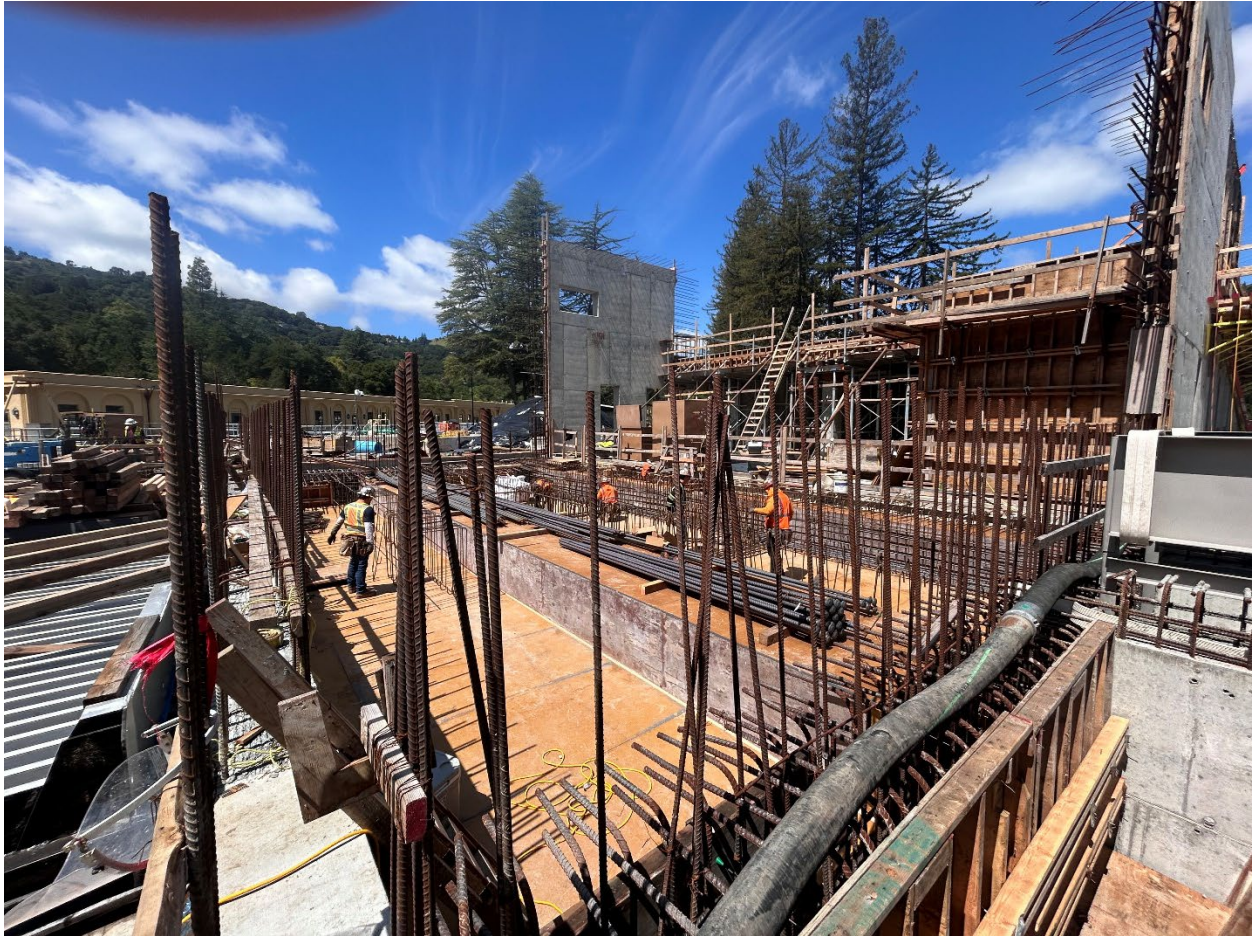
Figure 21 – Ironworkers installing rebar on wood decking for the MAUVE Building floor. This is the MAUVE Building south end.
