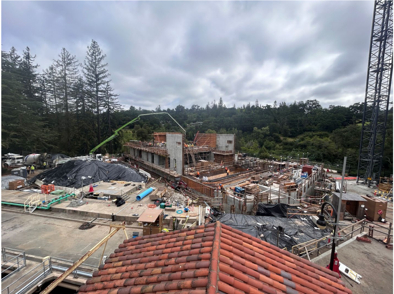
Figure 20 – View of the MAUVE Building under construction. The green articulating boom in the photo is pumping concrete from the concrete trucks to the wall forms for the second floor.
