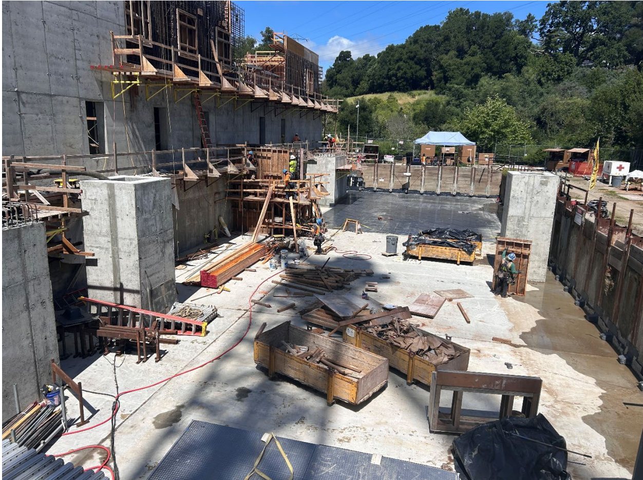
Figure 2 – View of workers installing black waterproofing material on the concrete roof of the Chlorine Contact Basin (CCB) which will be buried below the ground surface. The concrete ‘chimneys’ are the some of the accessways for the underground CCB.
