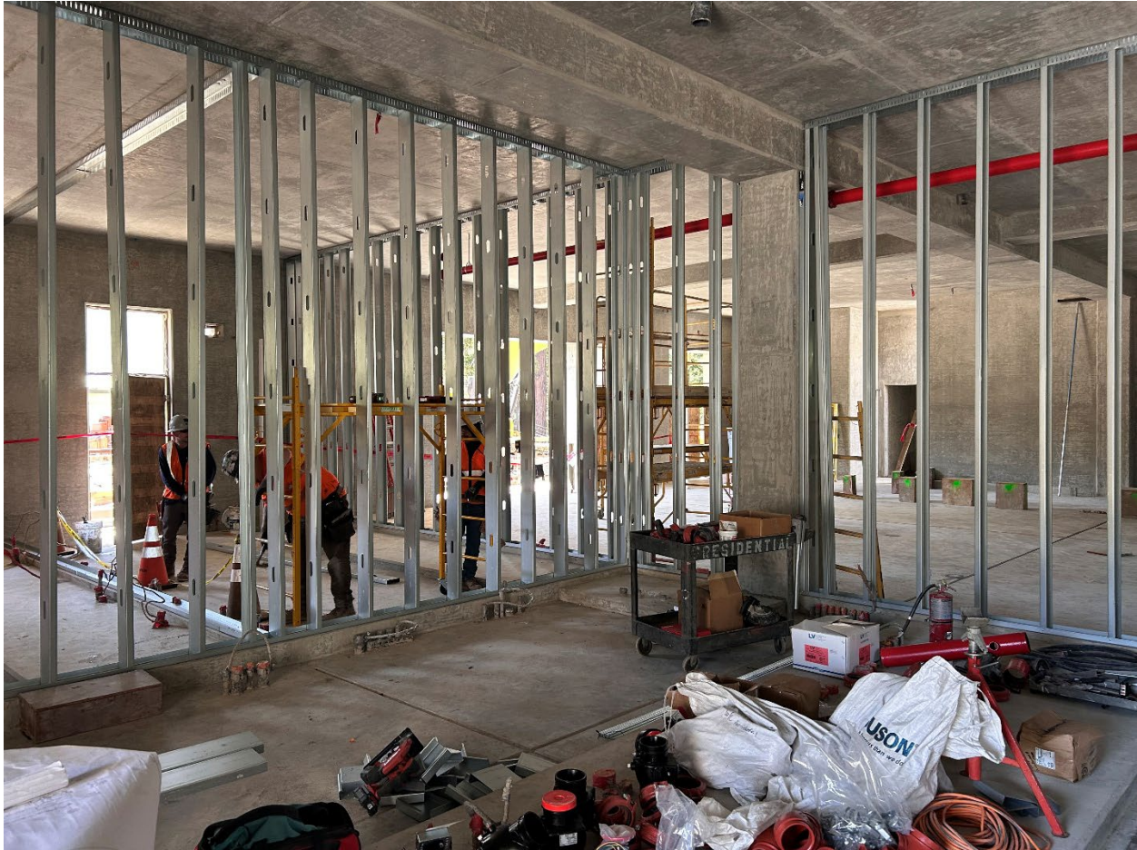
Figure 30 – View of carpenters installing metal stud interior walls on the first floor of the north end.
