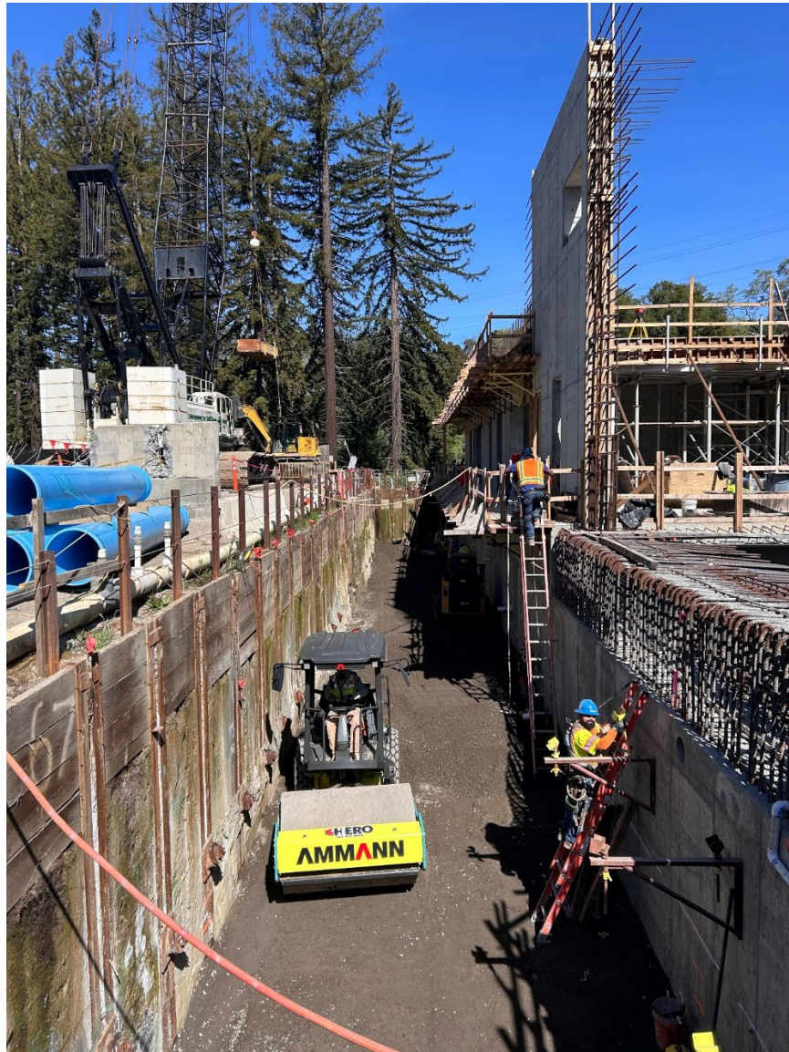
Figure 1 – View of workers placing and compacting engineered fill above the UV Inlet Channel in preparation for underground utilities for the MAUVE building.
