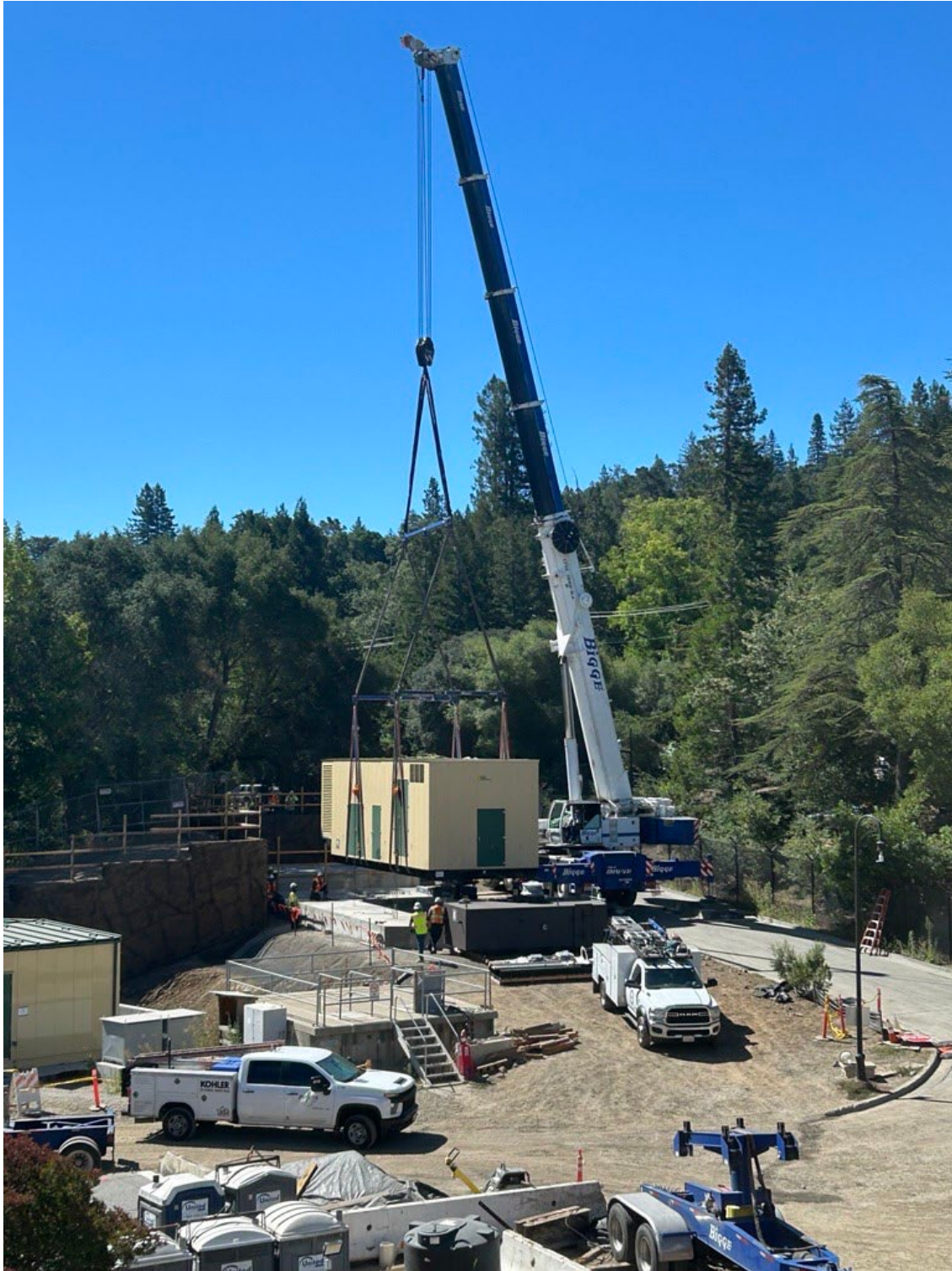
Figure 15 – View of crane lifting 2.5 megawatt emergency standby generator onto its concrete foundation pad.
