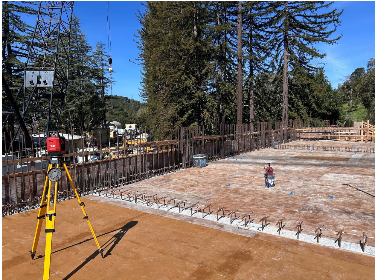
Figure 23 – View of the wood decking which will support the reinforced concrete for the MAUVE Building second floor.
