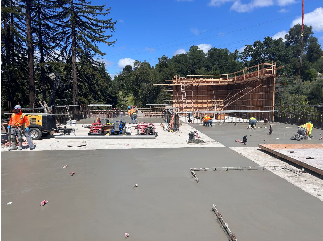
Figure 25 – Workers finishing concrete for the second floor of the MAUVE Building north end.
