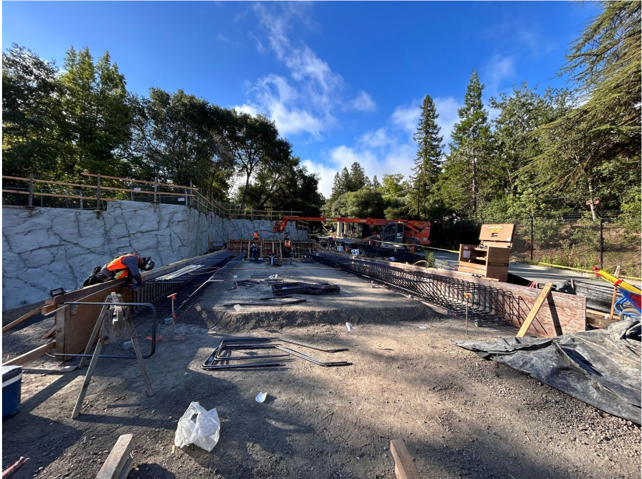
Figure 14 – View of ironworkers placing reinforcing steel for the concrete foundation which will support the future emergency generator. The decorative face of the retaining wall can be seen behind the workers.
