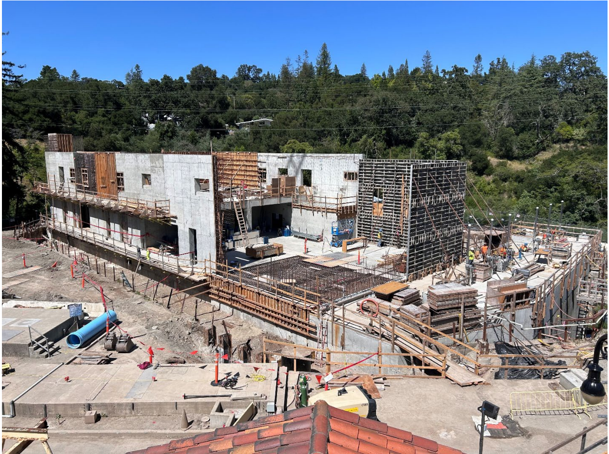
Figure 26 – View of the MAUVE Building south end walls under construction.
