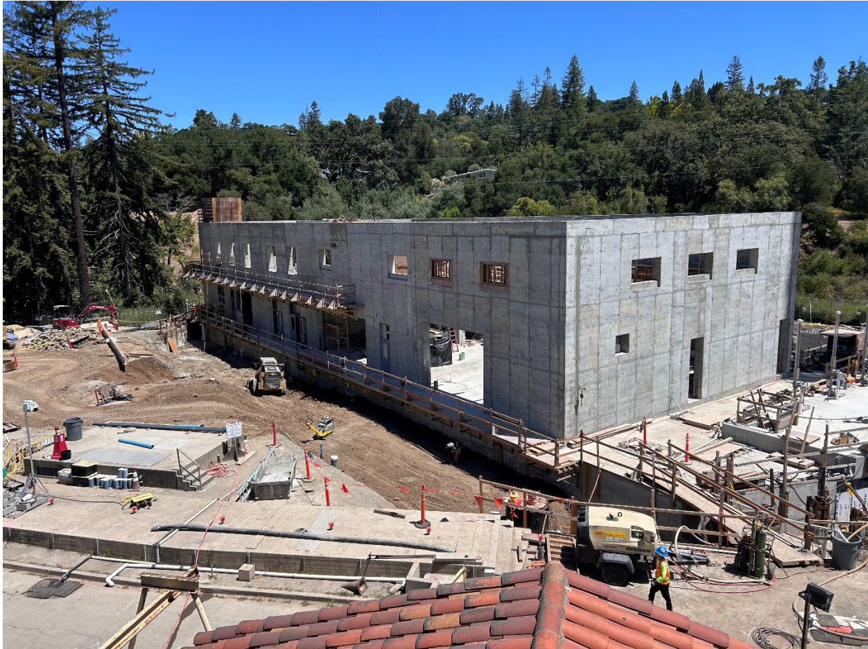
Figure 28 – View of MAUVE Building concrete shell completed. This includes both the south and north ends.
