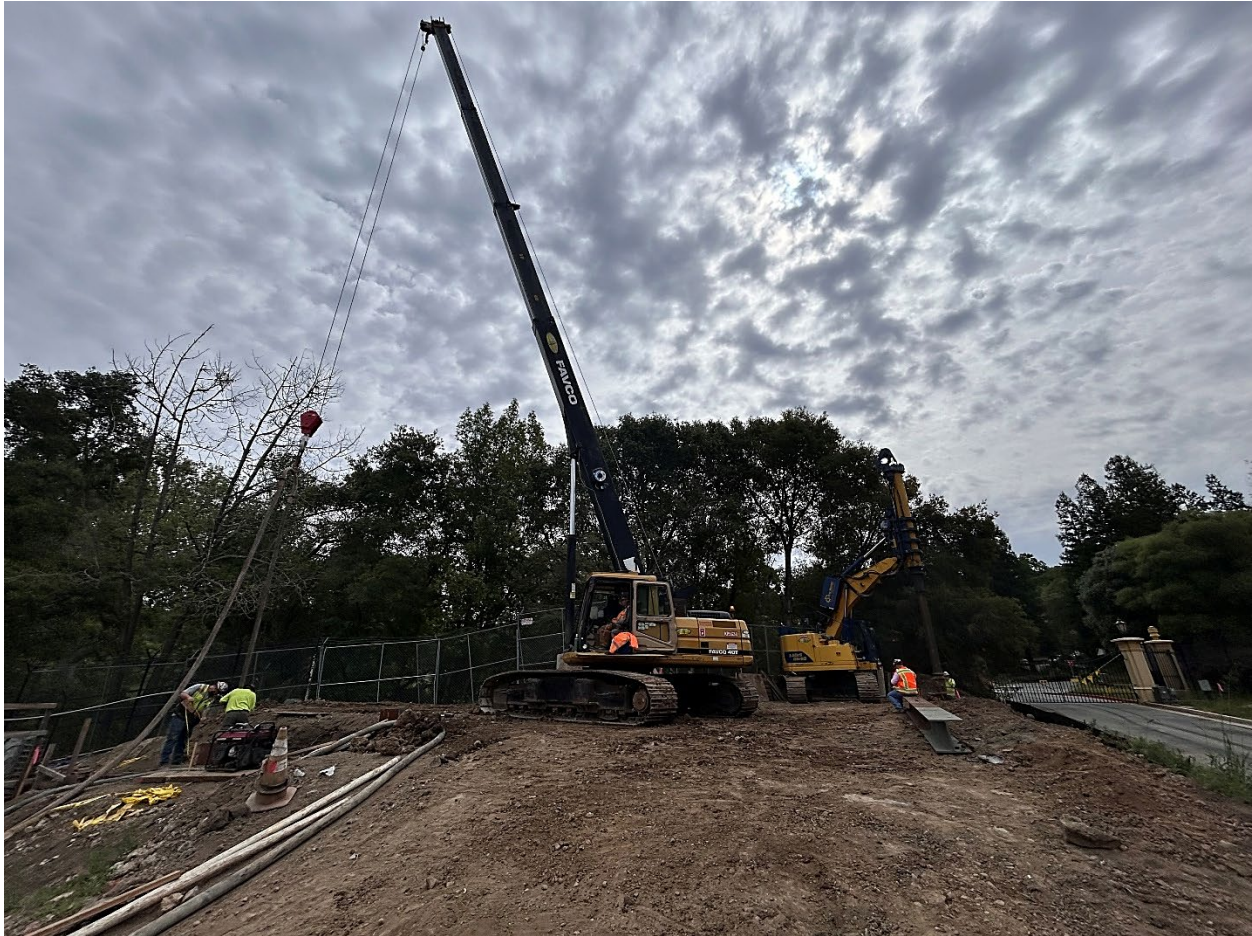
Figure 11 – View of carpenters drilling holes and installing underground beams in holes. The beams are part of the retaining wall system which allows the hillside to be supported while it is excavated down to a level surface.
