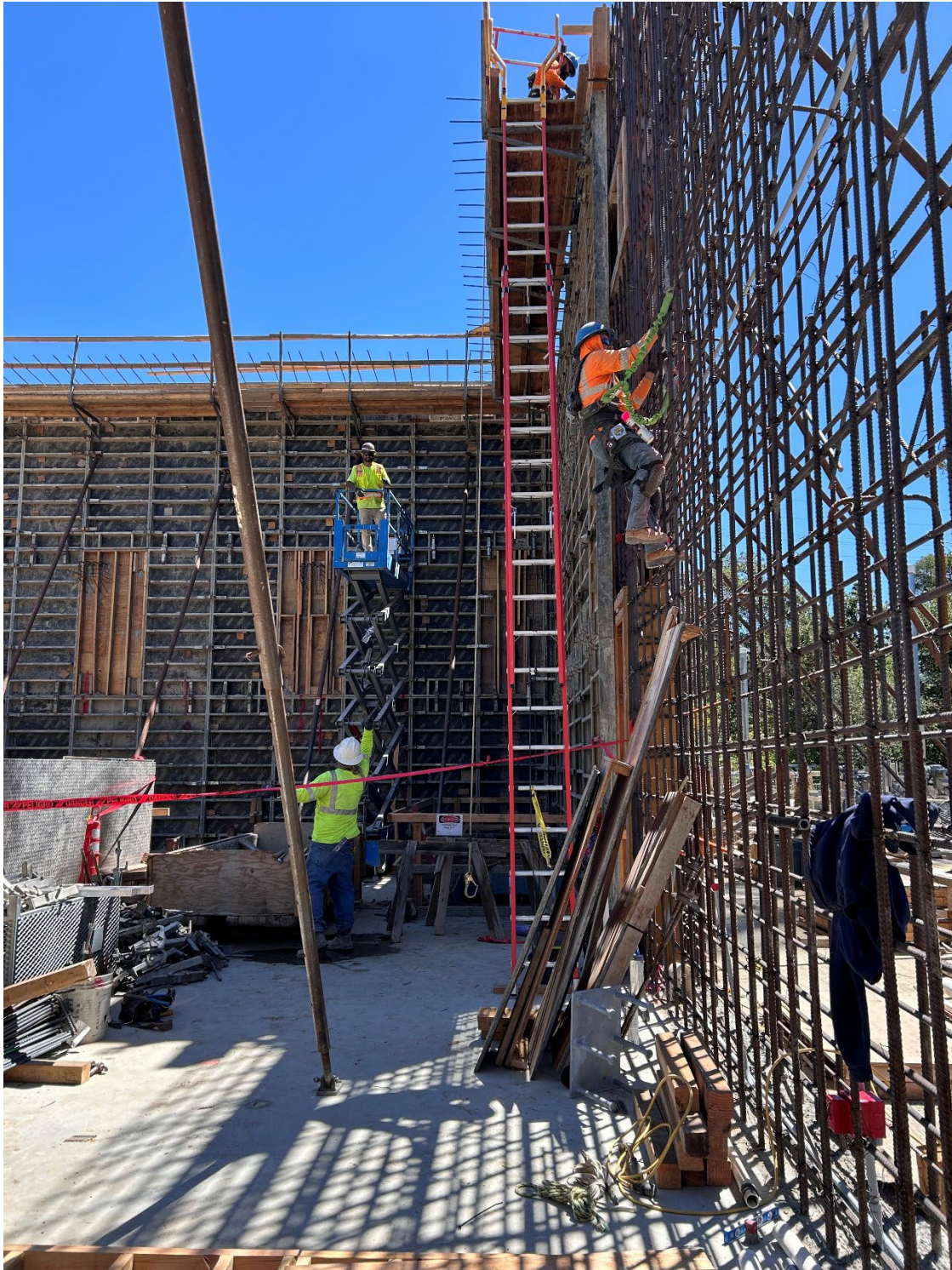
Figure 27 – Ironworker placing reinforcing steel wall curtain for MAUVE Building south end concrete walls.
