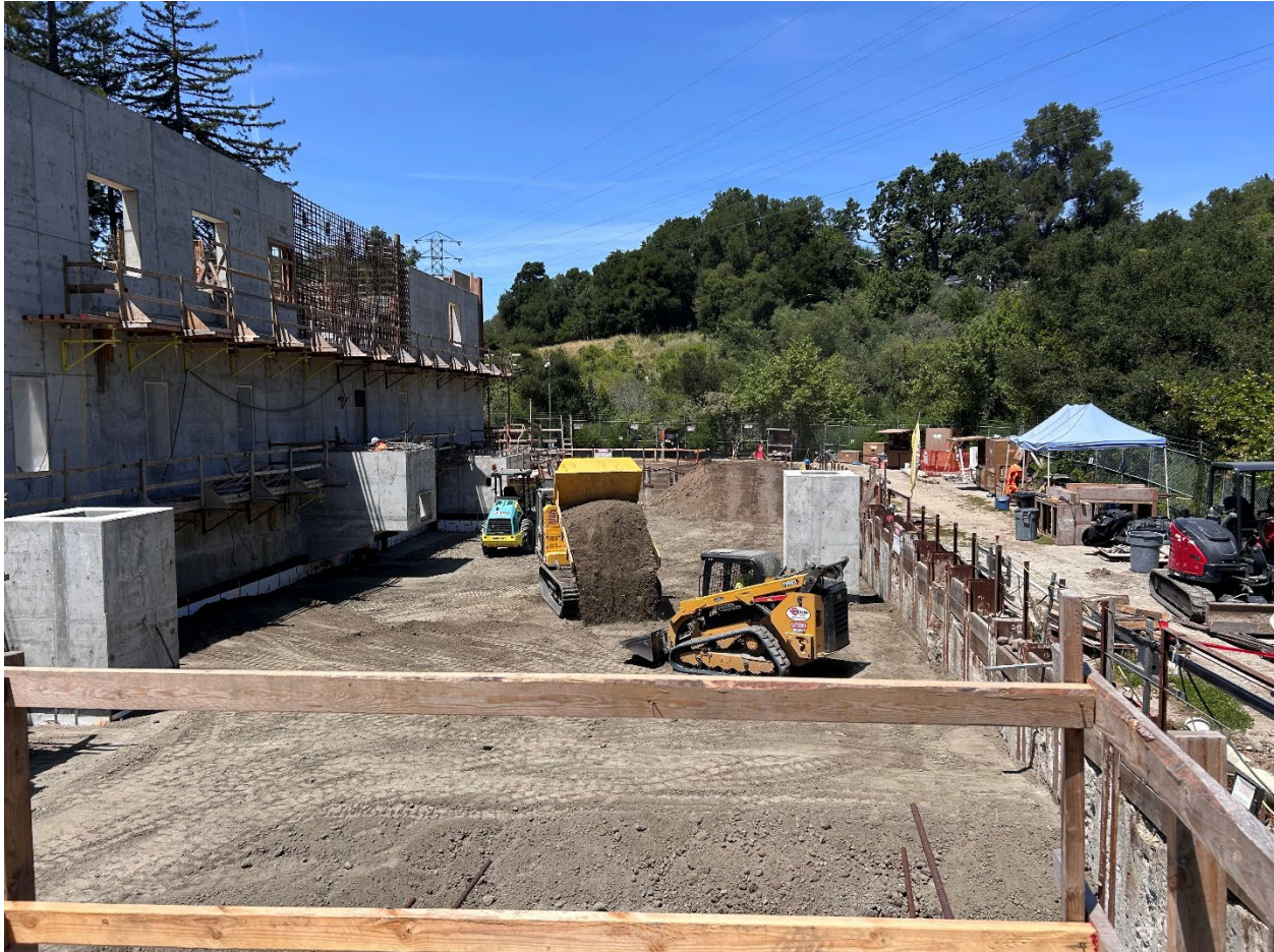
Figure 4 – View of workers burying the underground CCB. The photo shows a miniature dump truck emptying engineered-fill with other machinery redistributing and compacting the backfill in place.
