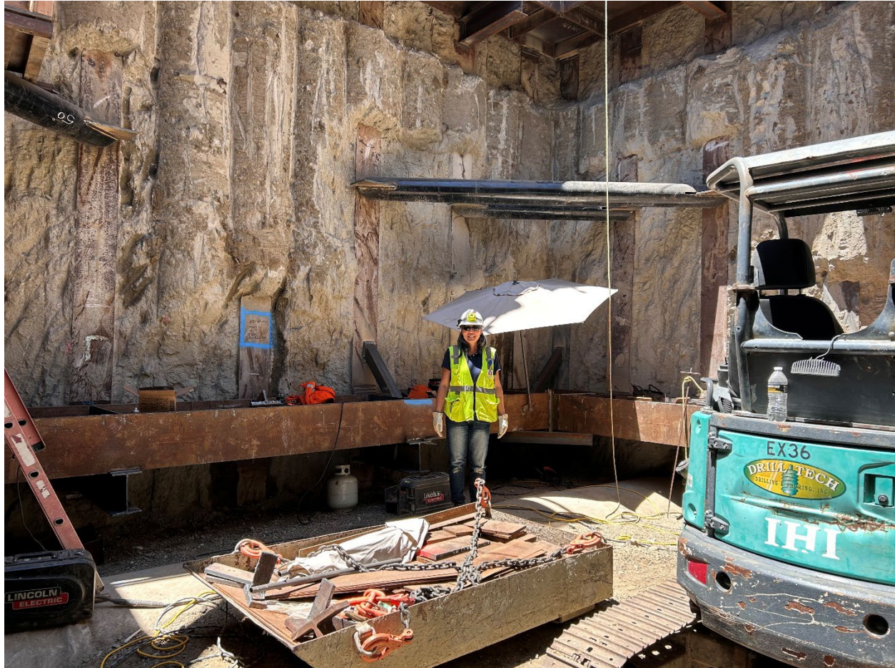
Figure 9— Engineer performing inspection at the interim bottom of the Effluent 2 excavation. The engineer is standing adjacent to the existing 78-inch Effluent 2 pipeline which must be evaluated and field measured accurately to complete the design and fabrication of the connecting pipeline. The excavation will continue another 15 feet below the feet of the engineer to fully expose the existing Effluent 2 pipeline and the new Effluent 2 connection tunnel.
