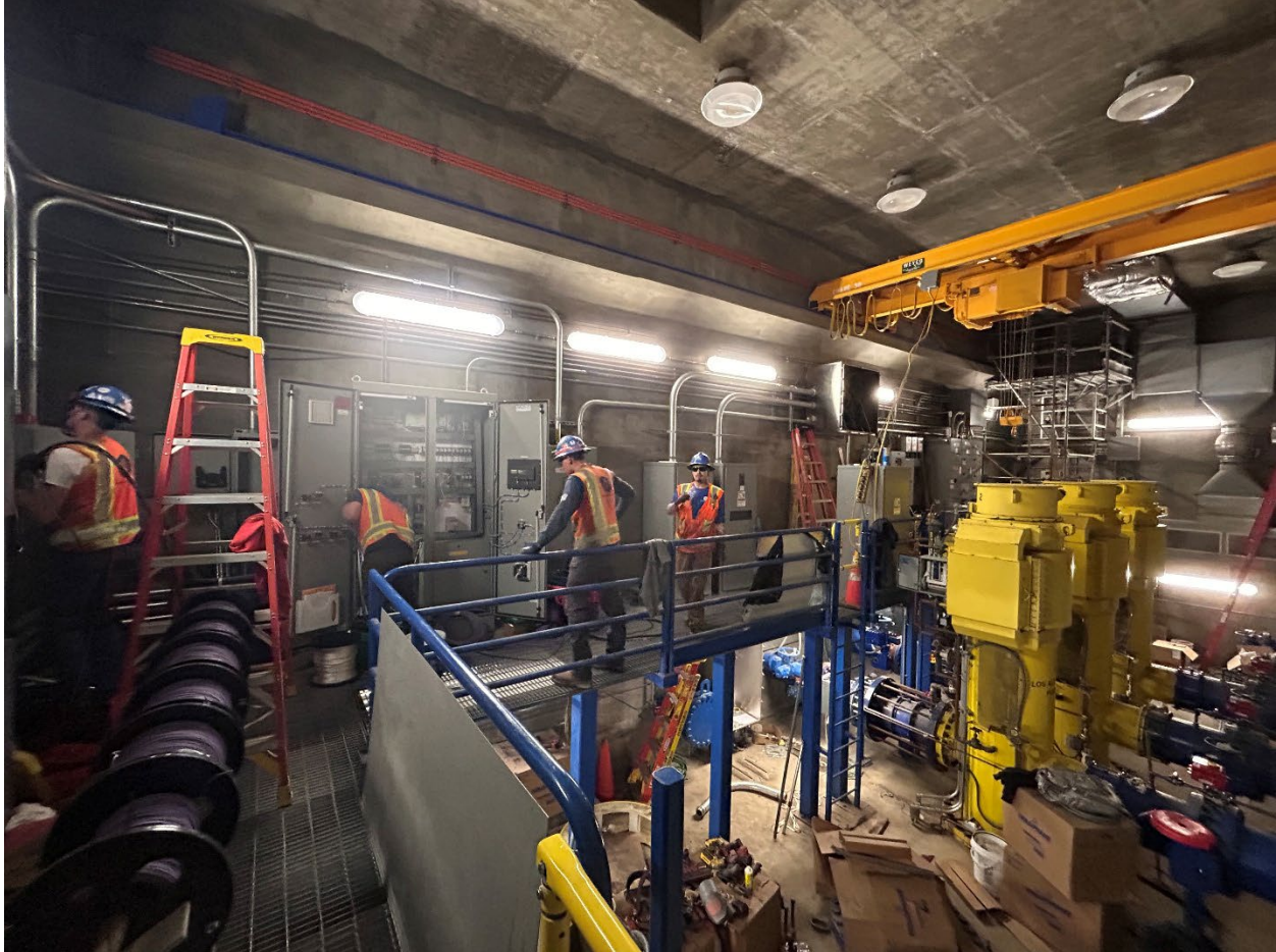
Figure 16 – Electricians installing medium voltage switching equipment in the underground Los Altos Pumping Plant No. 2. This pumping plant is located 40 feet below the ground surface at the Orinda WTP.
