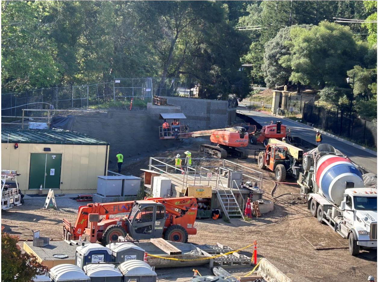
Figure 13 – View of retaining walls after excavation of the hillside. The workers on the manlift are applying shotcrete to the retaining walls to strengthen them. The level area created by the excavation is the location of foundation for the future emergency generator.
