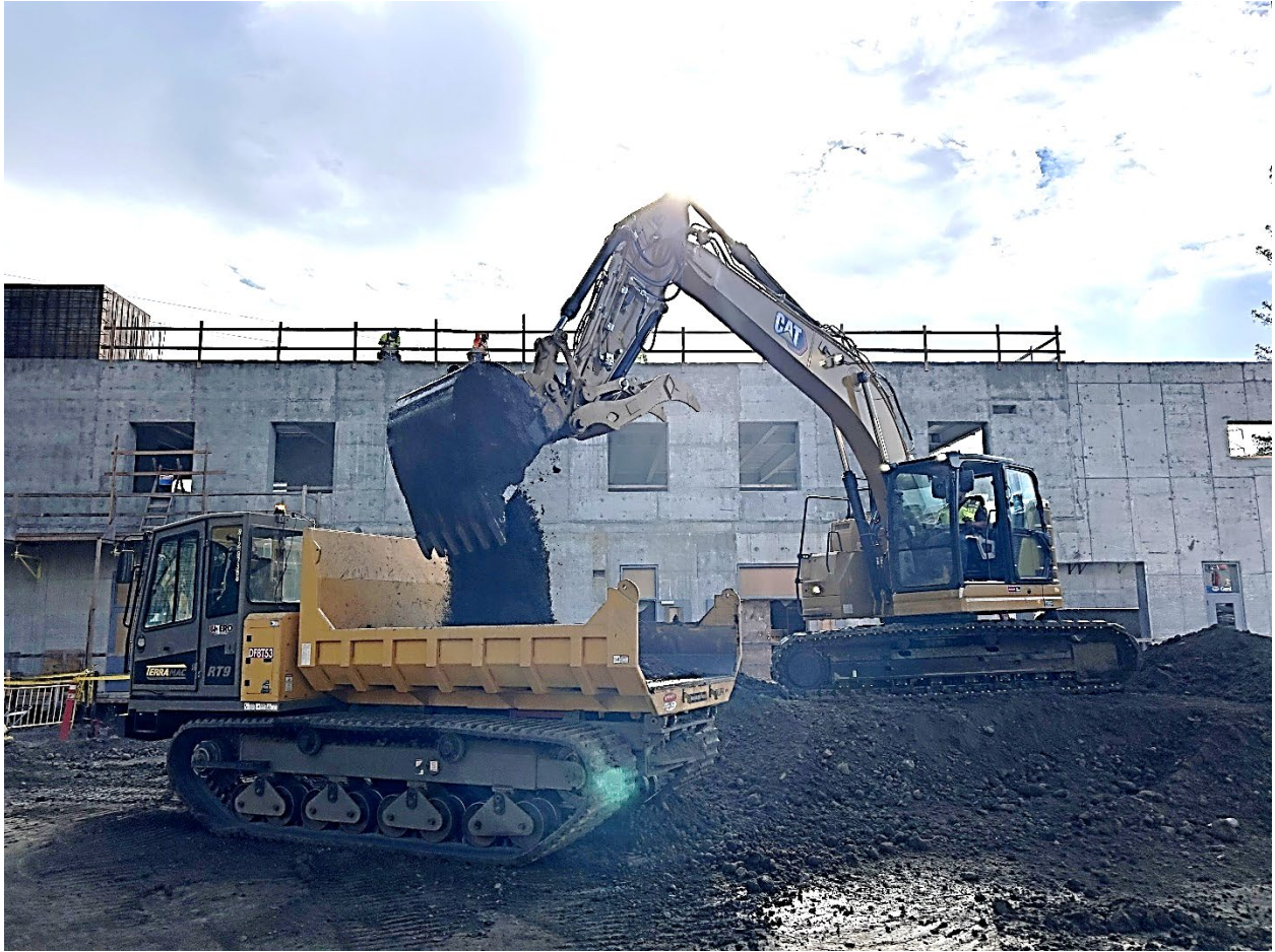
Figure 3 – View of an excavator filling a miniature dump truck with engineered fill which will cover the buried CCB.
