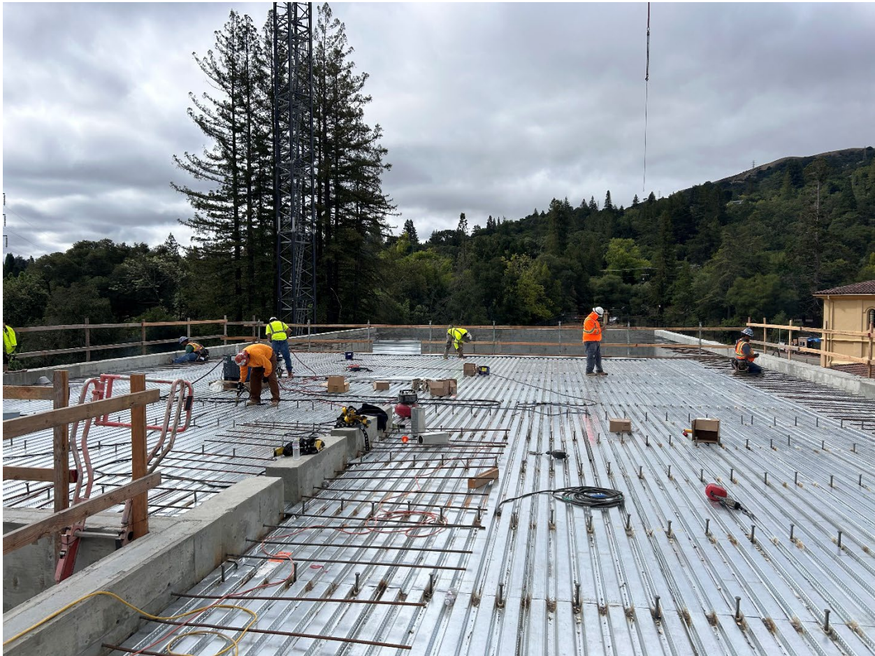
Figure 29 – View of ironworkers placing metal pan deck which will support the MAUVE Building north end roof.
