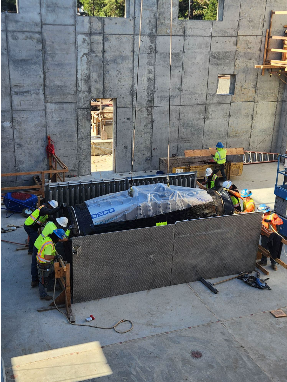
Figure 33 – Closeup view of crane lowering first UV disinfection vessel through the access hatch in the first floor of the MAUVE Building with the careful guiding hands of many workers.
