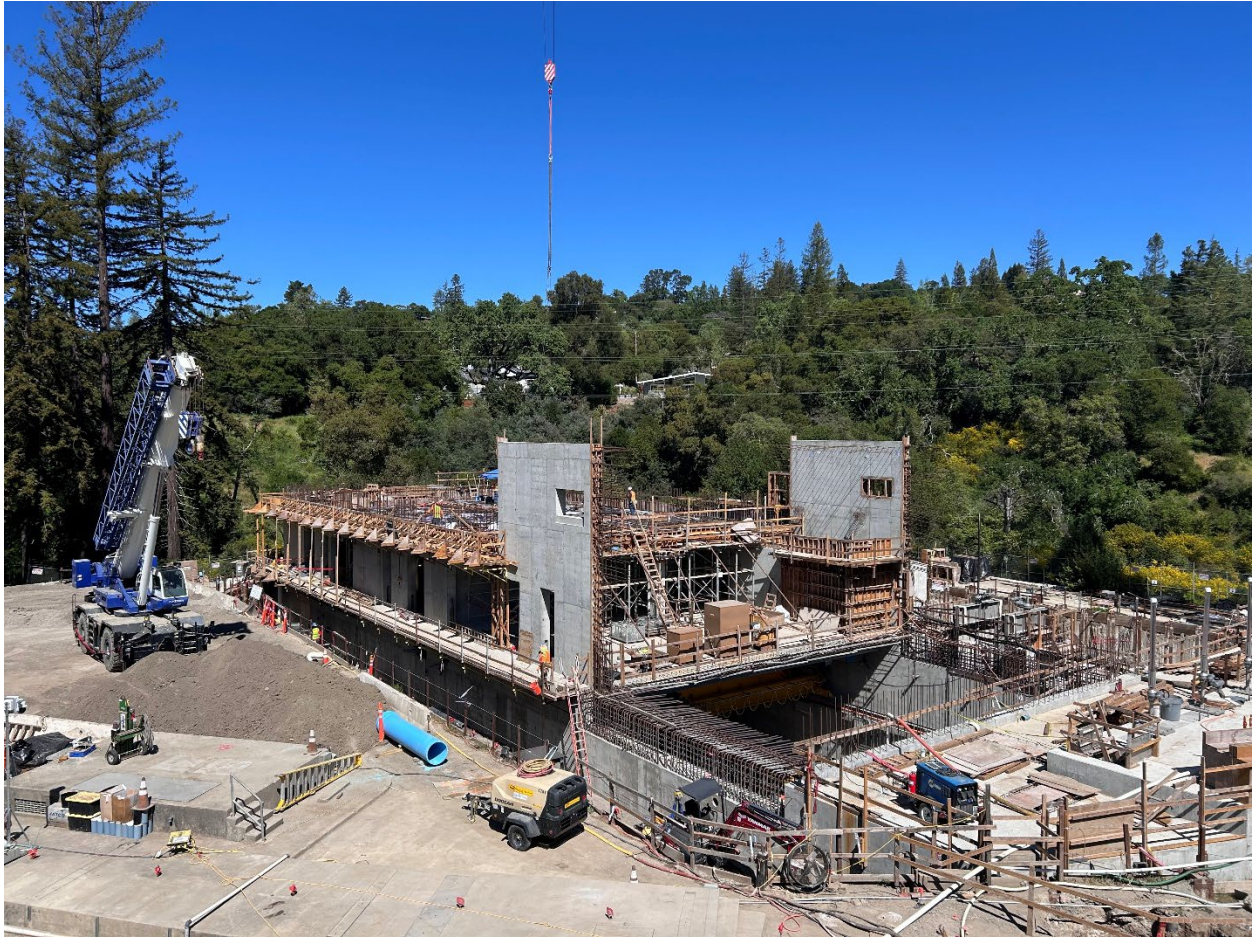
Figure 19 – View of the first floor of the MAUVE Building north end under construction. The building is constructed in two segments. The large opening in the MAUVE Building concrete floor in the foreground serves as easy access for very large piping into the UV Room located 30-feet below the floor.
