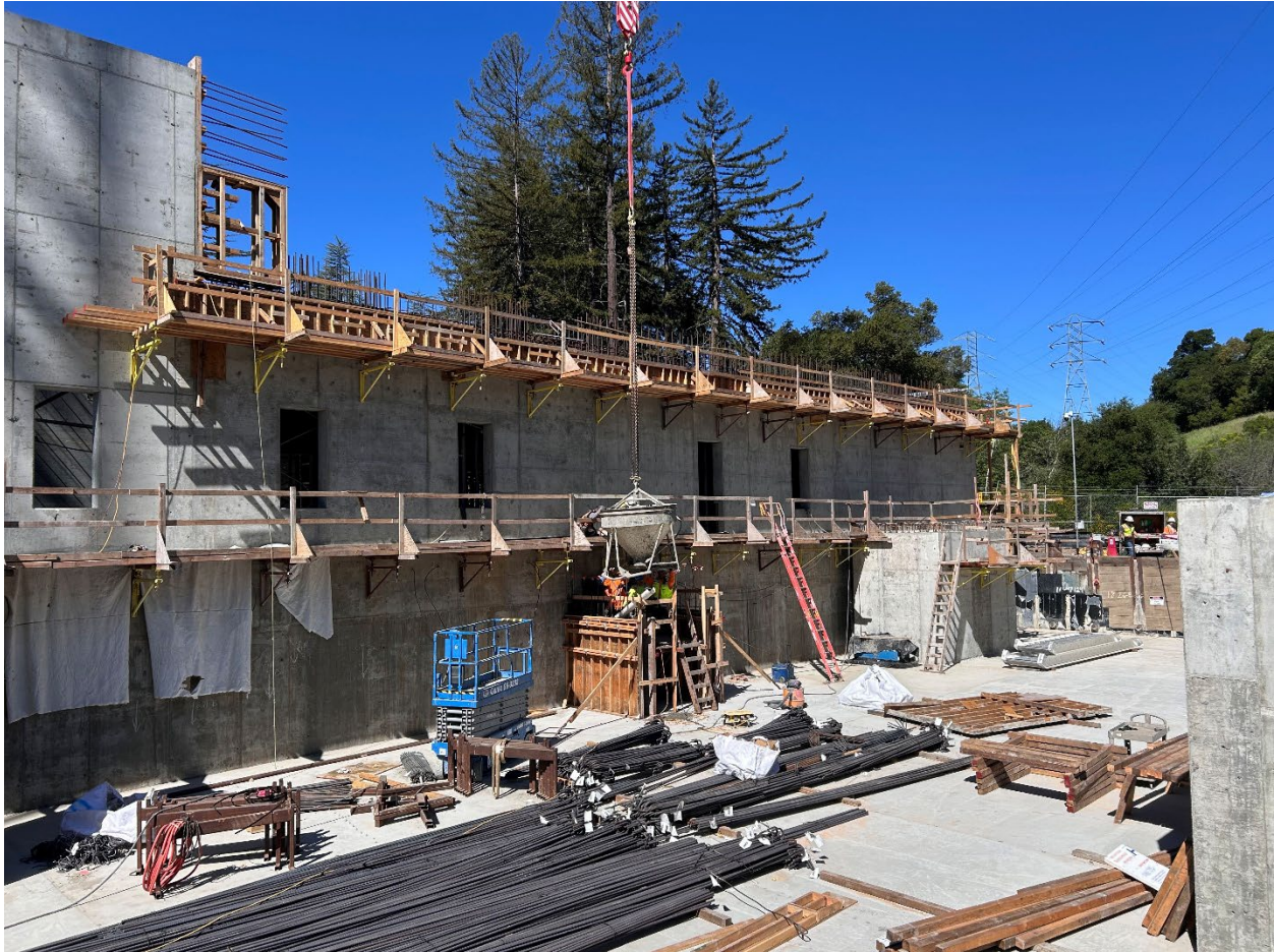
Figure 22 – Laborers using a large hopper to place concrete with the aid of the tower crane on the backside of the MAUVE Building. Hard-to-access areas such as this require special concrete placement techniques.
