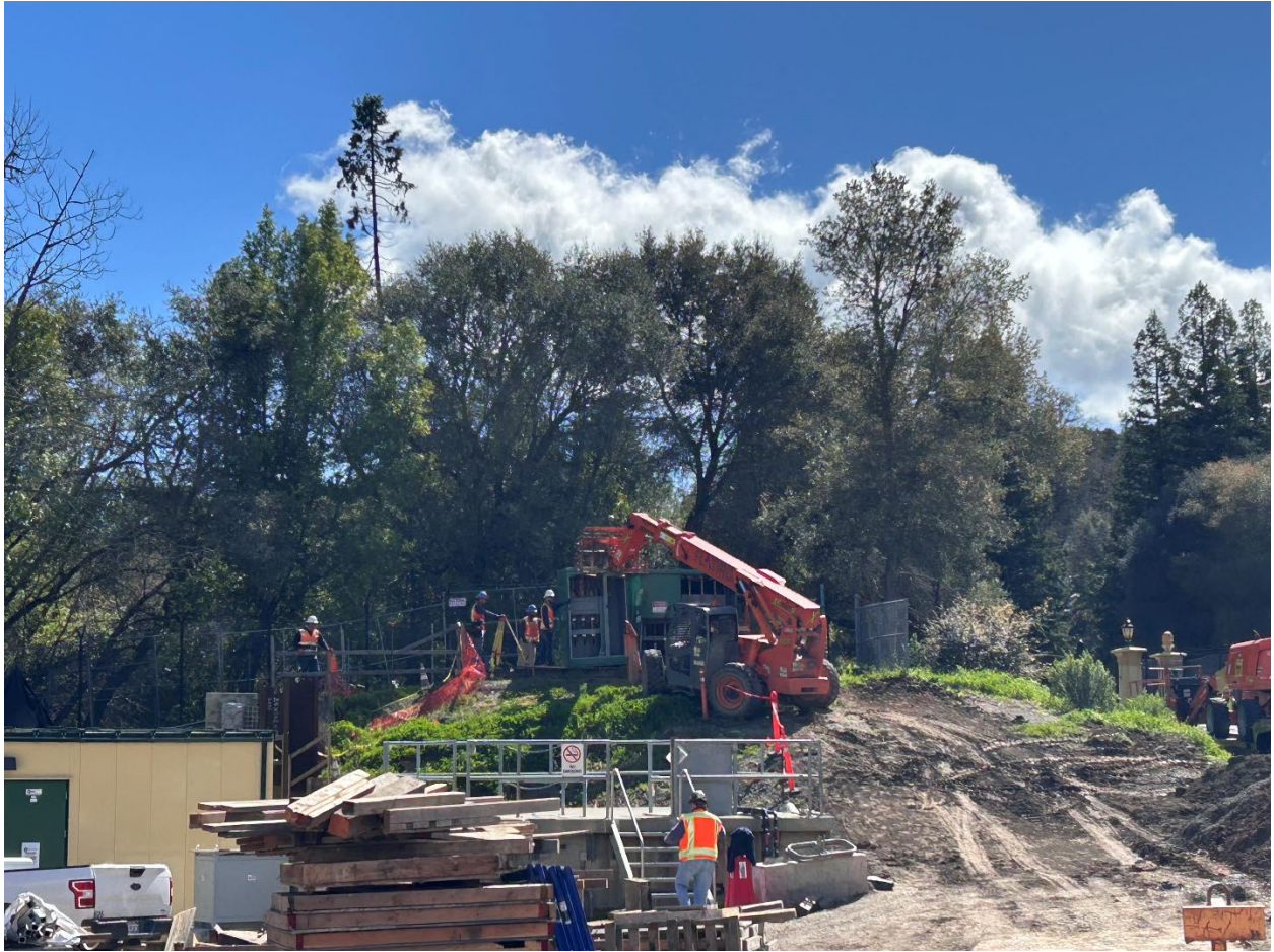
Figure 10 – View of electricians demolishing the transformer for Los Altos Pumping Plant No. 2 in preparation for constructing the foundation for the new emergency generator.
