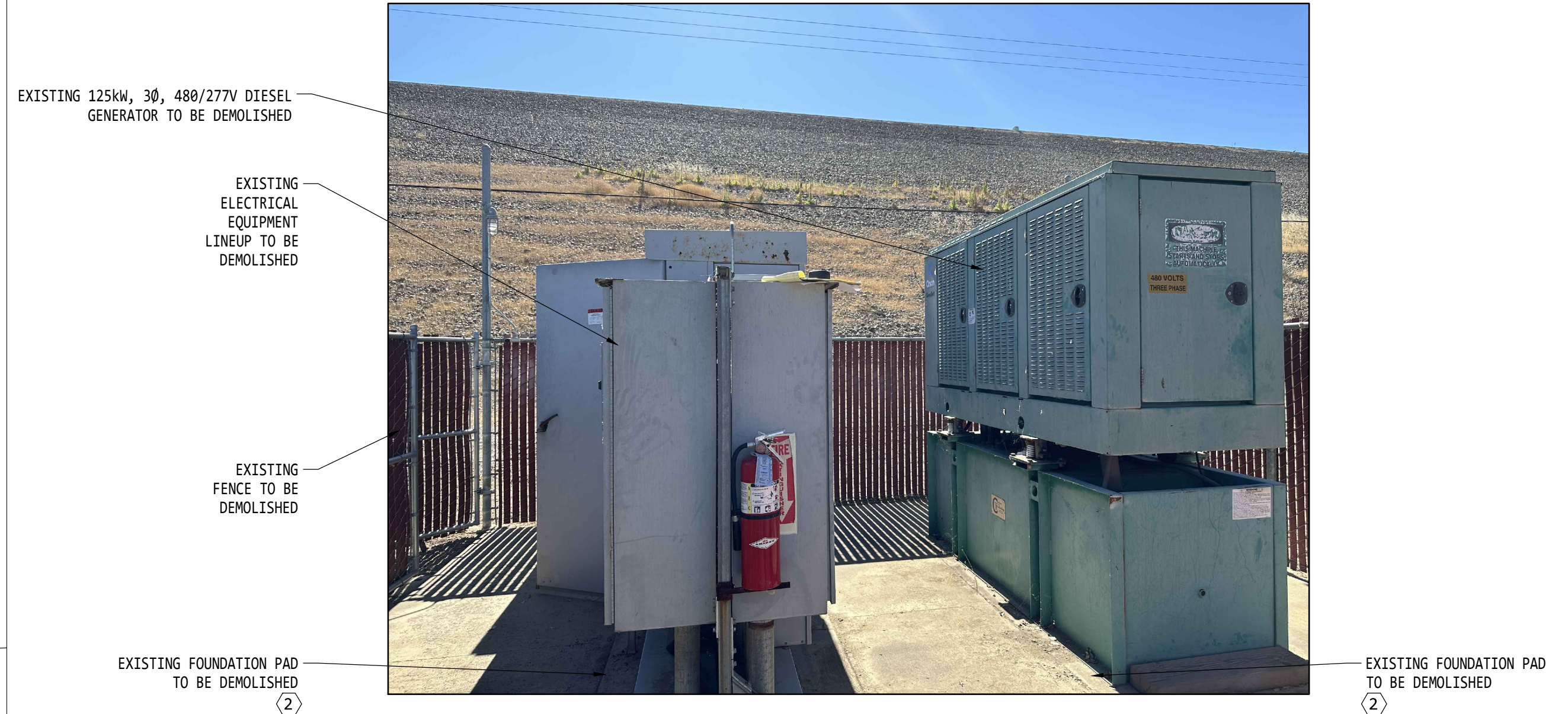
EXISTING SWITCHBOARD & GENERATOR NOT TO SCALE
