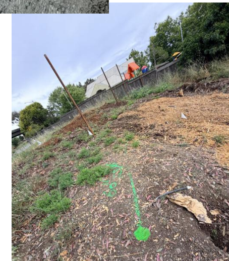
Utility marking (USA) prior to City excavation work
