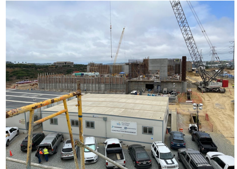
Pure Water San Diego construction site Photo courtesy of F. Wedington
