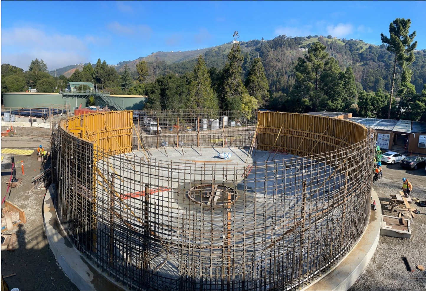
Figure 11 – Gravity Thickener: construction of perimeter wall underway
