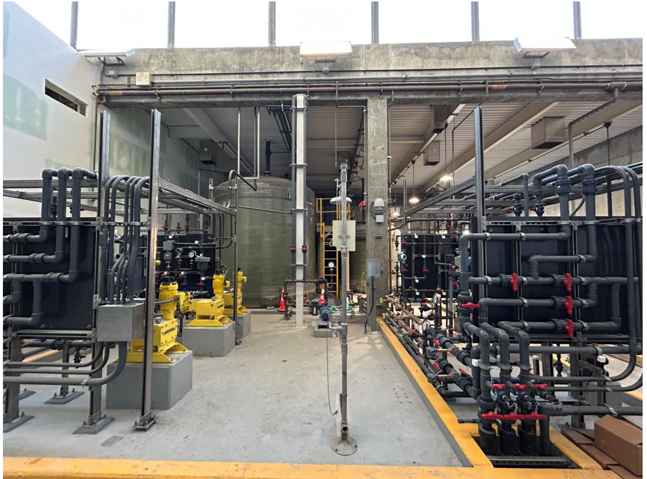
Figure 14 – Sobrante WTP: chemical area ongoing work for permanent chemicals
