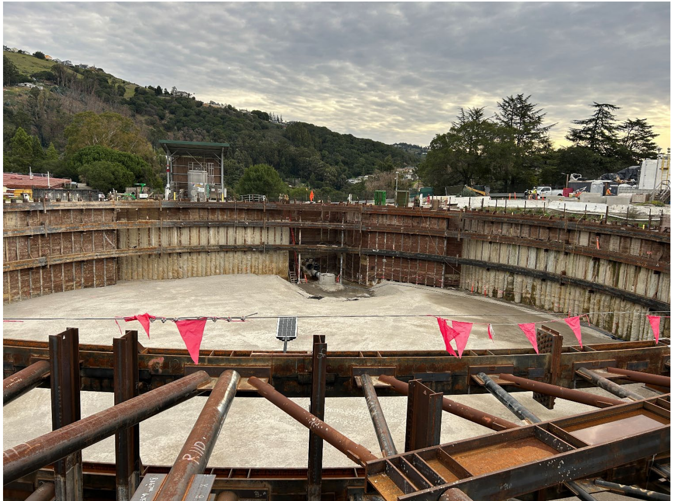
Figure 5 –Chlorine Contact Basin: excavation with completed subgrade preparation
