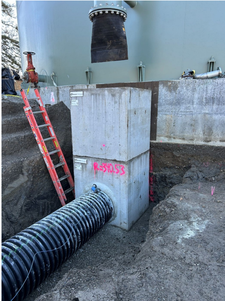
Figure 1 – Spent Wash Water Basin 3: completed the emergency overflow vault and piping
