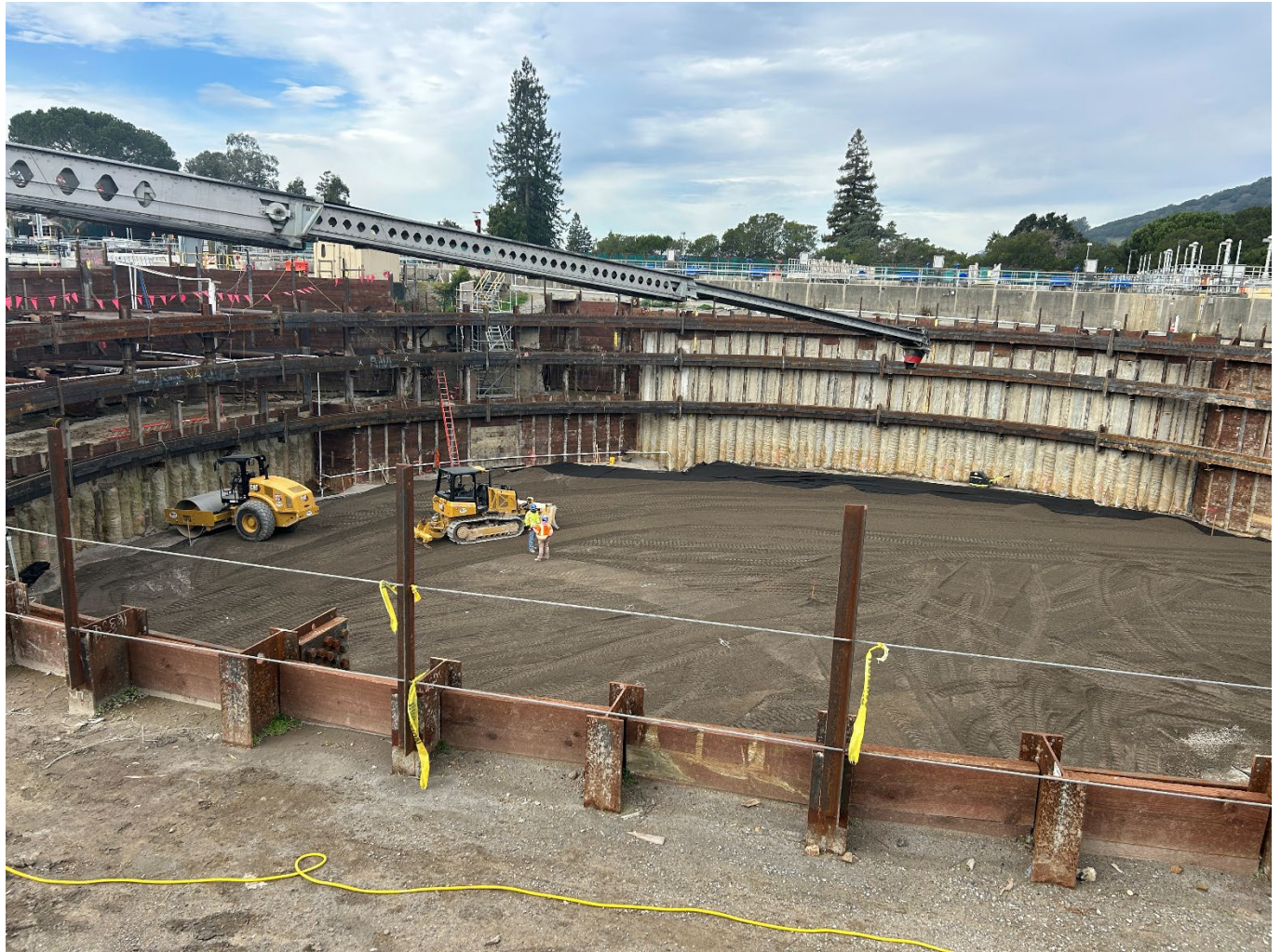
Figure 4 – Chlorine Contact Basin: excavation subgrade preparation
