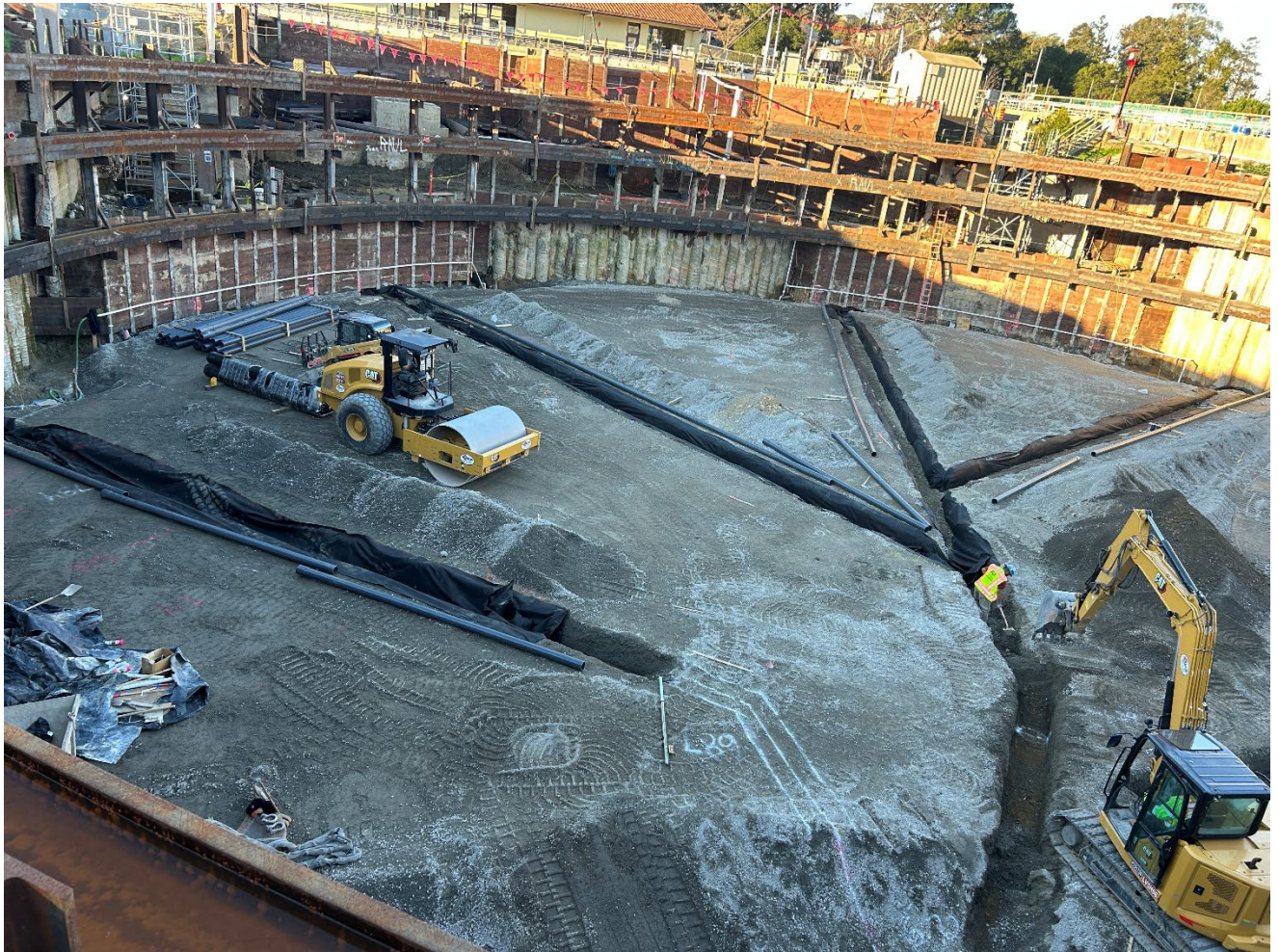
Figure 3 – Chlorine Contact Basin: underdrain installation
