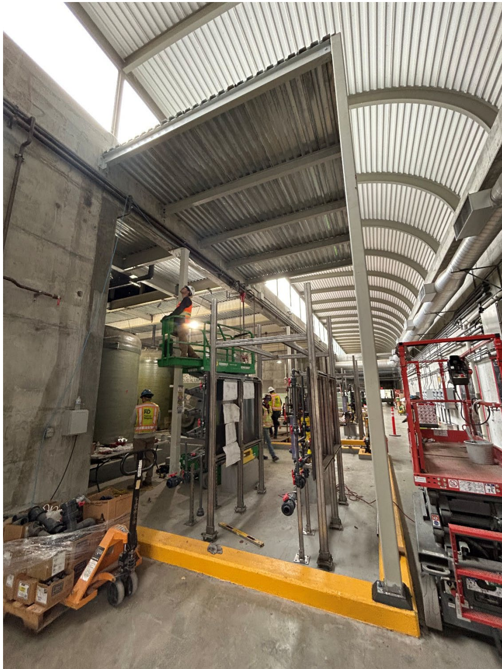
Figure 12 – Sobrante Chemical Building: Phase 1.2 electrical and chemical work ongoing
