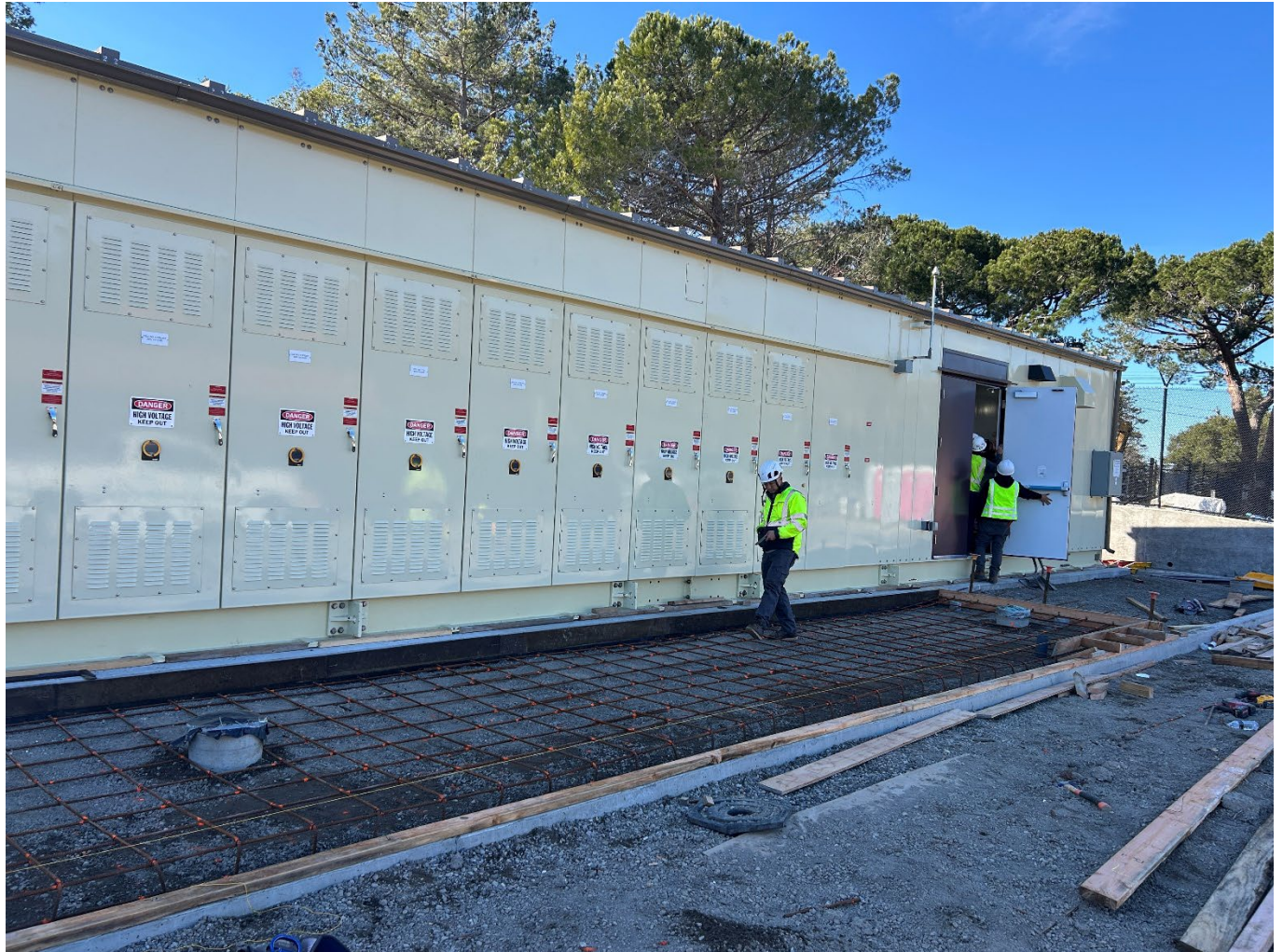
Figure 2 – USL Power Building: wiring work continues in preparation for energization
