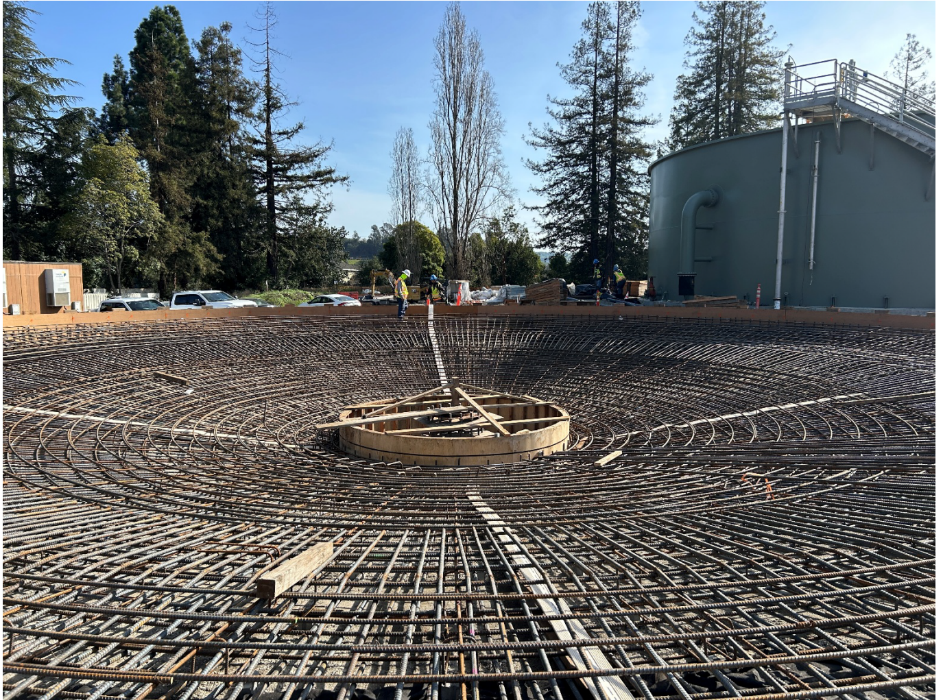
Figure 9 – Gravity Thickener: rebar mat for upcoming foundation pours
