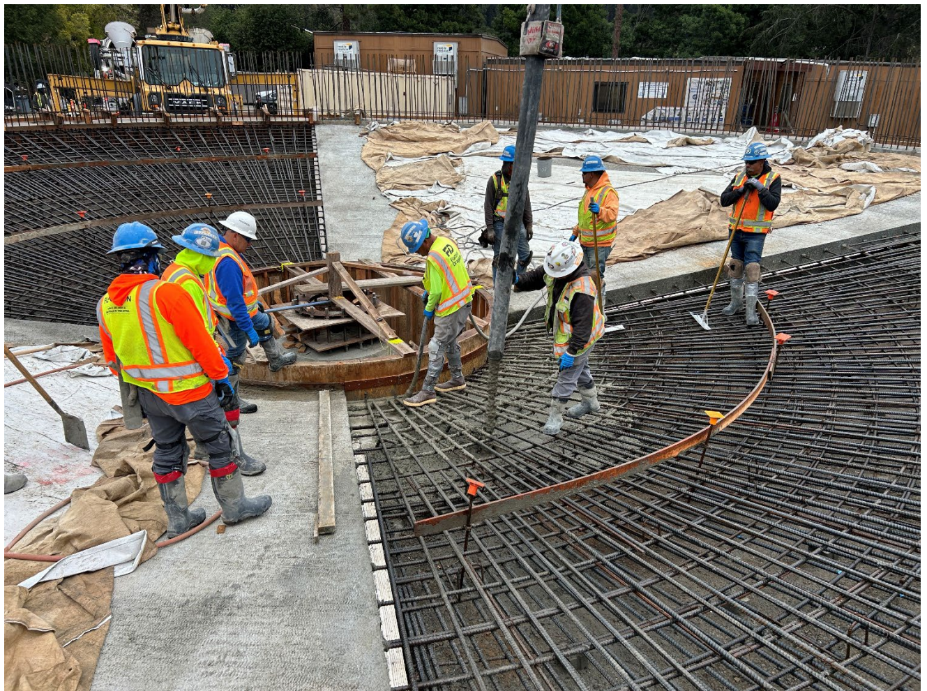
Figure 10 – Gravity Thickener: foundation concrete placement underway
