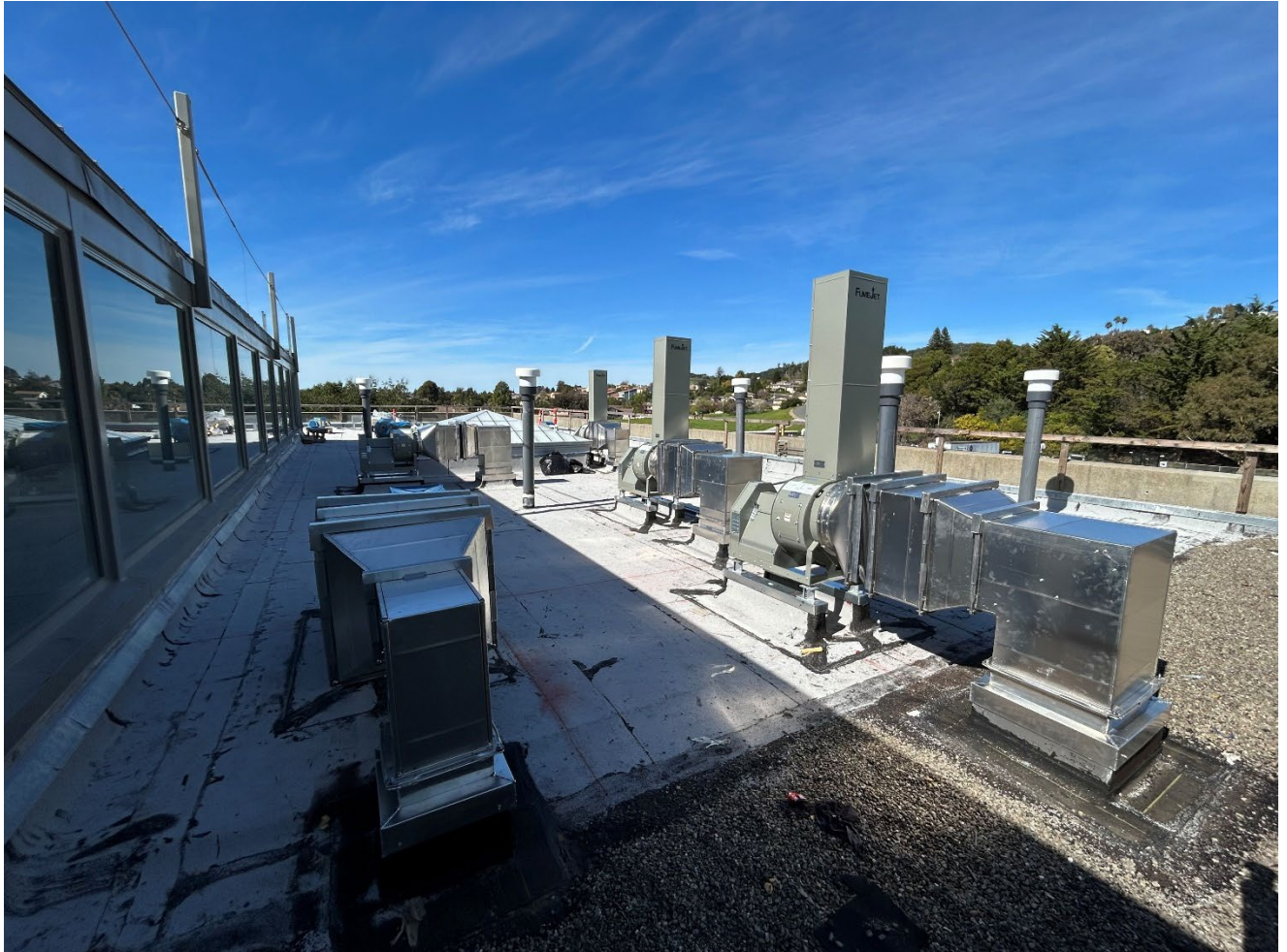
Figure 17 – Sobrante WTP Chemical Building Roof: completed HVAC equipment
