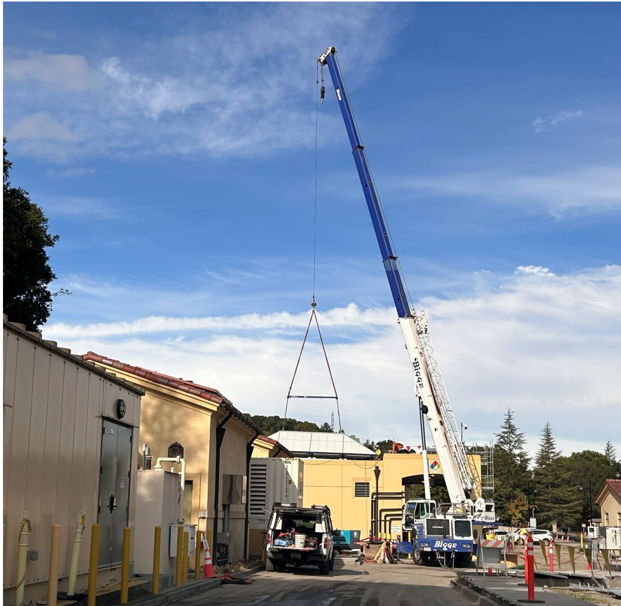
Figure 40 – Crane lowering skylight to close Chemical Building roof opening.
