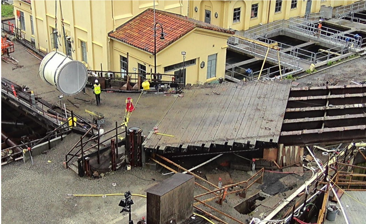
Figure 45 – UV-CCB Facility temporary bridge in partially demolished state.
