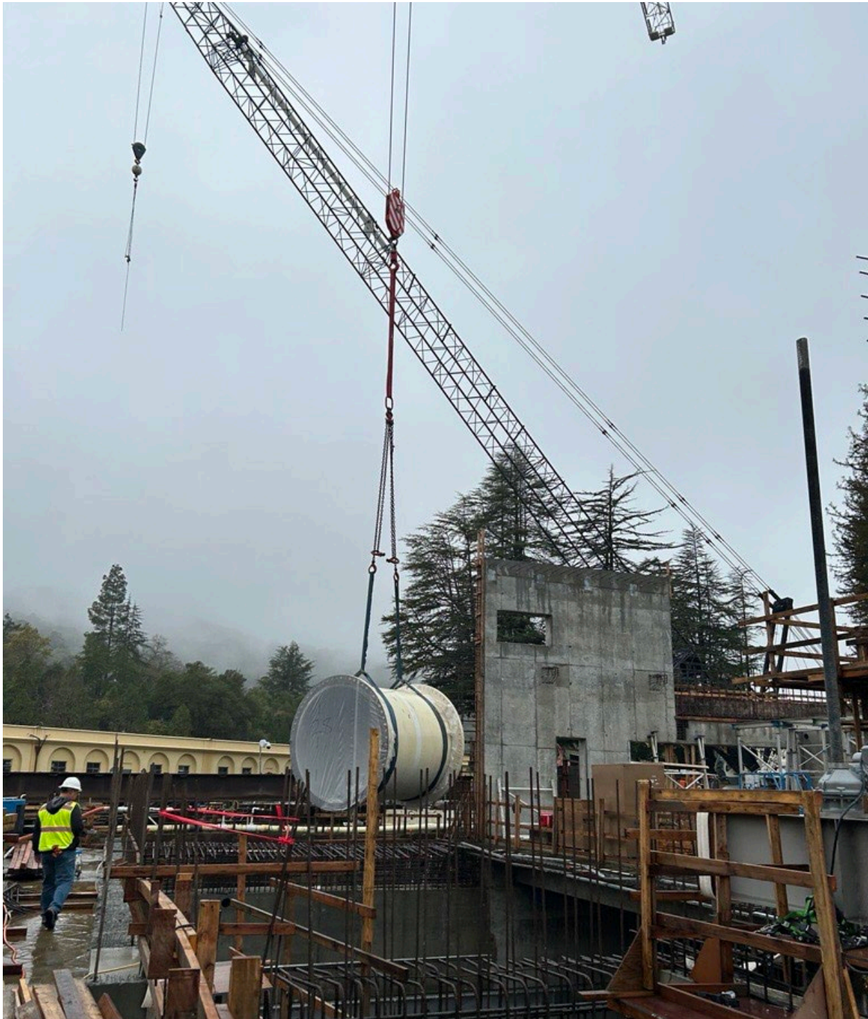
Figure 27 – Crane lowering 84-inch steel bypass piping into the UV Room below.
