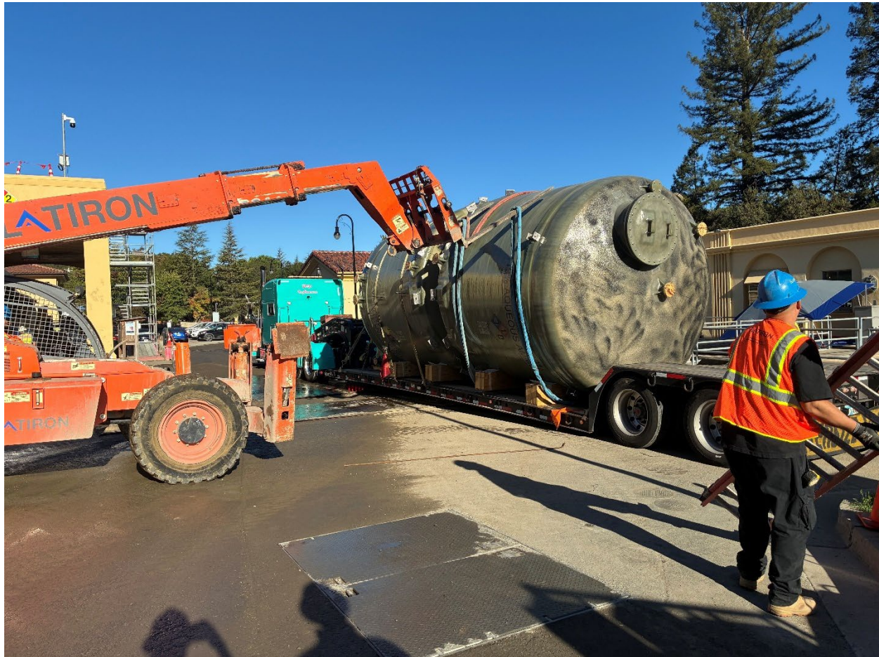
Figure 38 – Workers unloading fiberglass reinforced plastic chemical tanks from a delivery truck.
