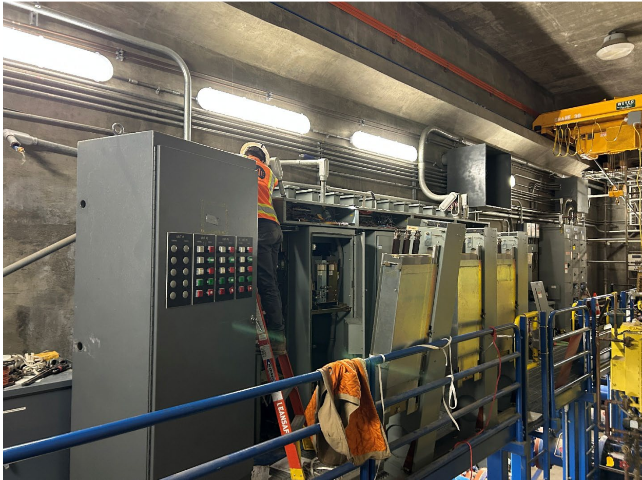
Figure 43 – Worker demolishing old electrical gear in LAPP2.
