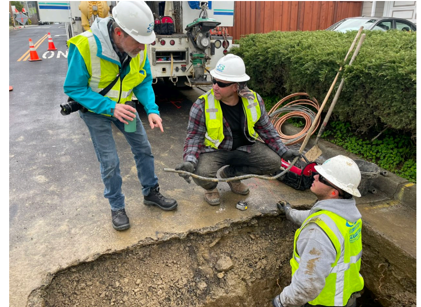
District employees extracting service line
