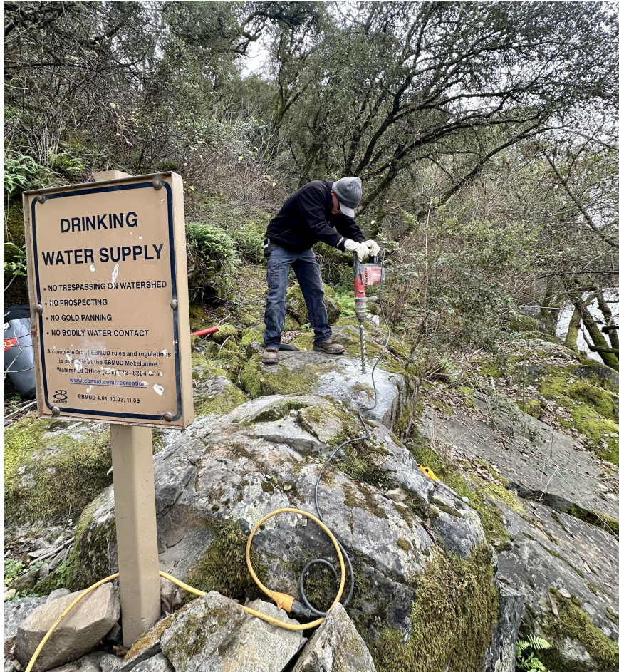
Ranger installing fence near Mokelumne River
