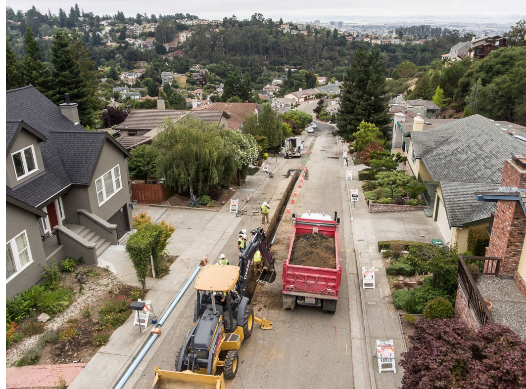
Pipeline Construction Project using Contracted Dump Truck Service
