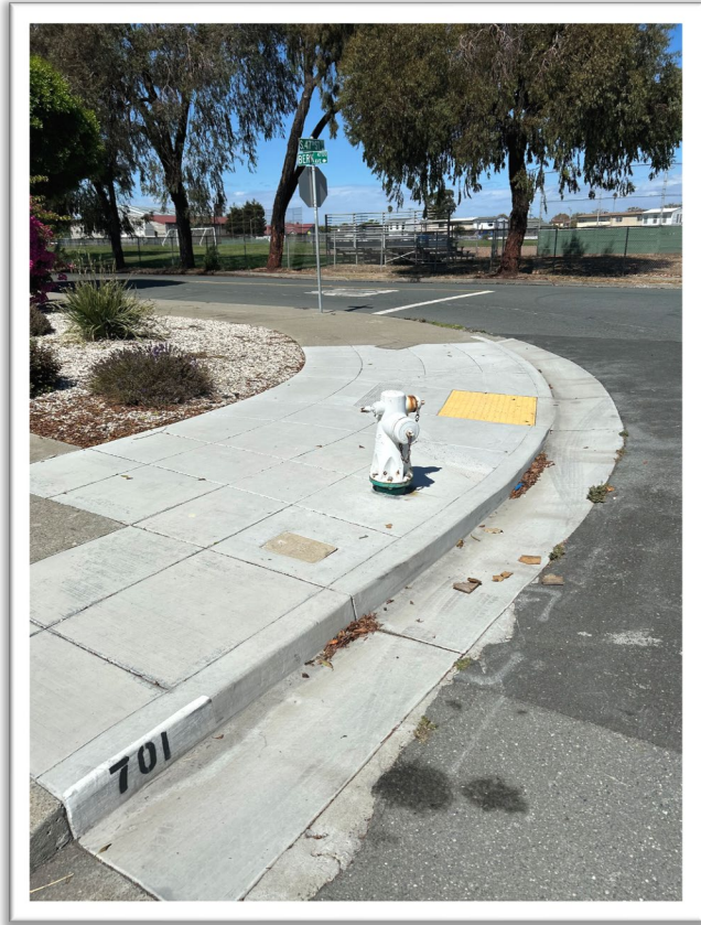
S. 47th Street, Richmond ADA Sidewalk Restoration Specialized Service
