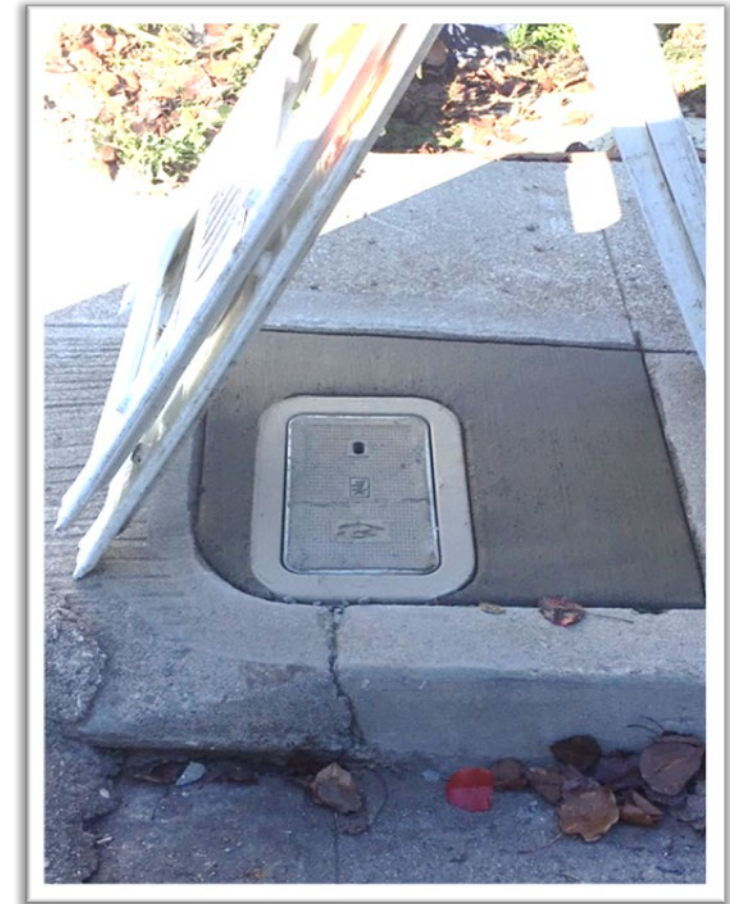
Meter Box Concrete Repair
