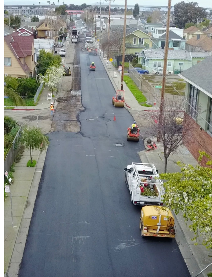
Extension paving by Contractors
