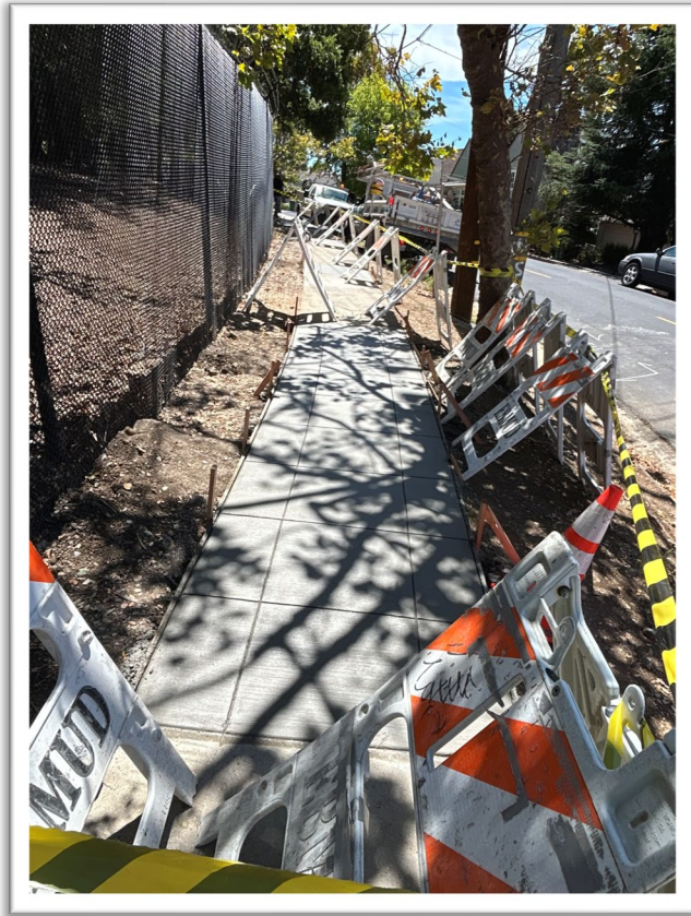
Berkeley Park Sidewalk Repair Per City Ordinance • Utilized 4 Finishers
