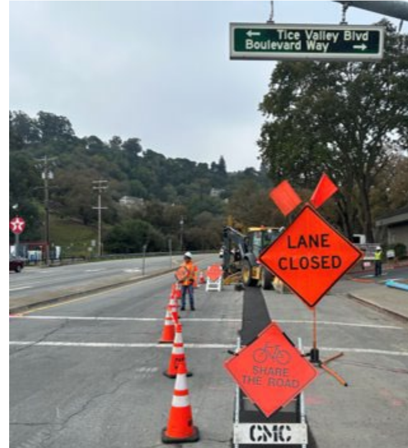
Contract Flaggers alongside District Forces Replacing Pipe in a Trench
