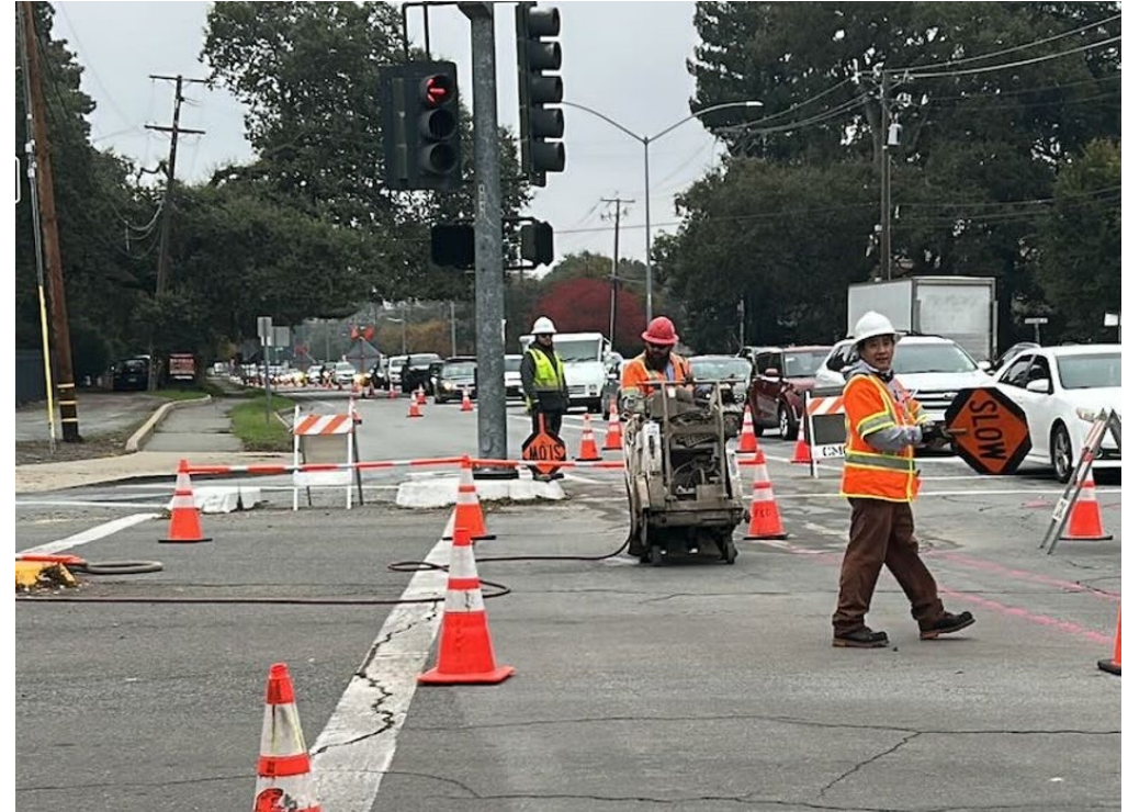
Contractor Performing Asphalt Saw-Cutting for District Pipeline Project
