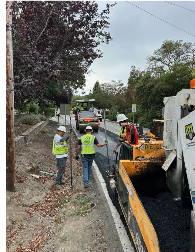
Extension paving in Oakland
