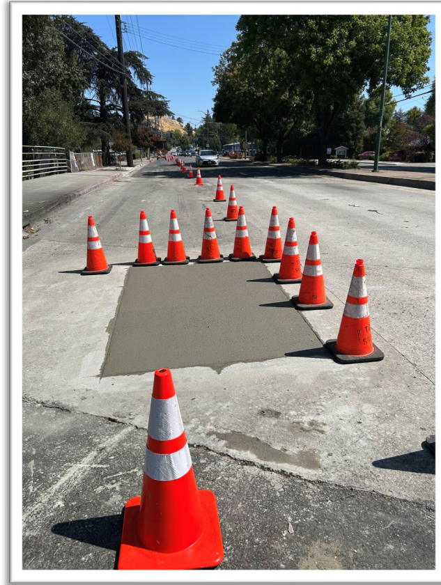
Ygnacio Valley Rd. Main Break • Utilized 4 Finishers
