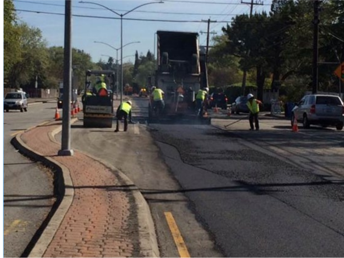
Extension Paving by District Forces
