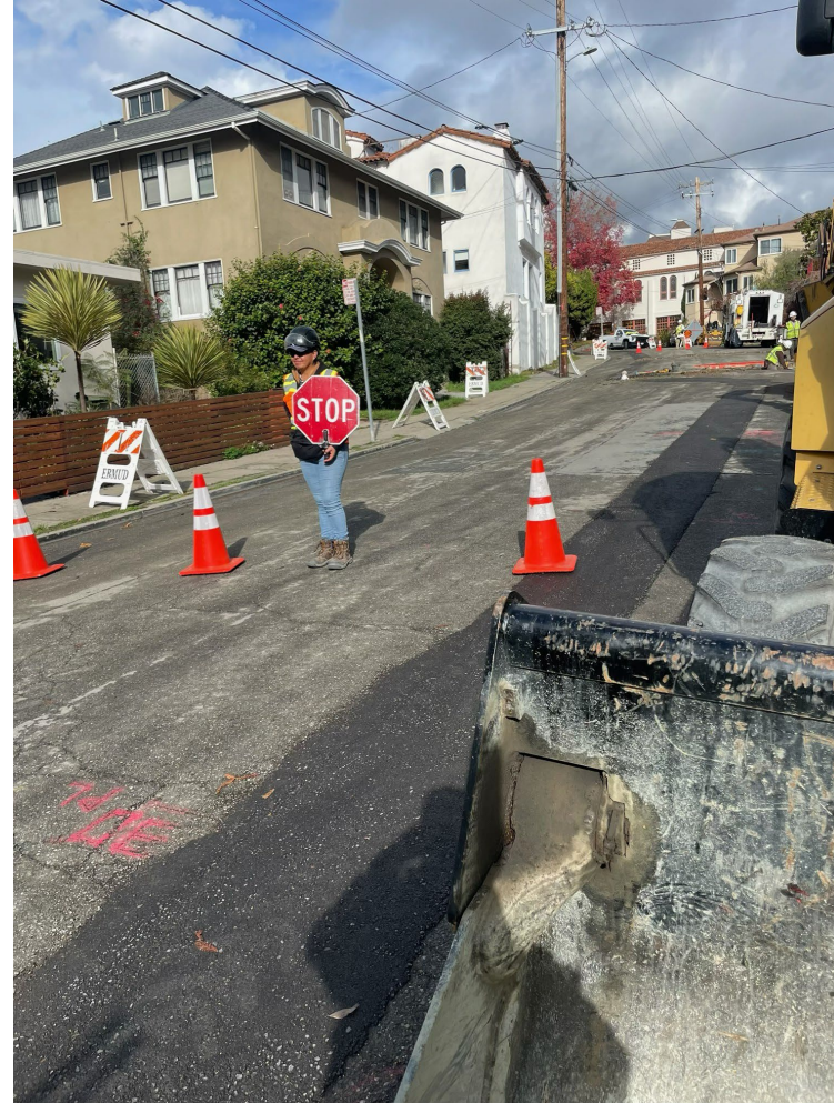
Contract Flagger at Work
