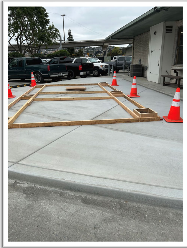
South Yard Rest Area Restoration • Utilized 5 Finishers
