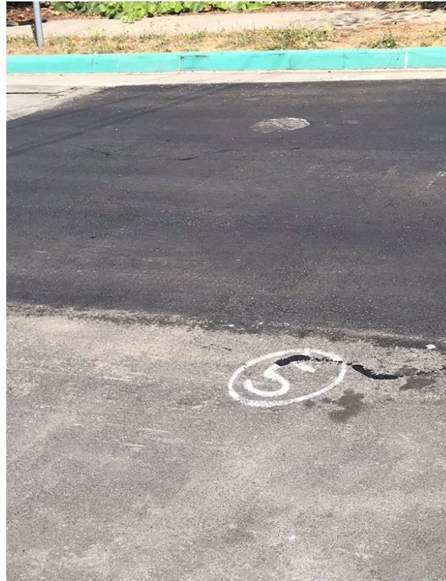
Patch paving in El Cerrito
