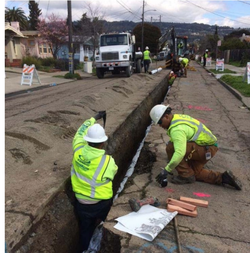
District Staff Working on a Pipeline Replacement Project
