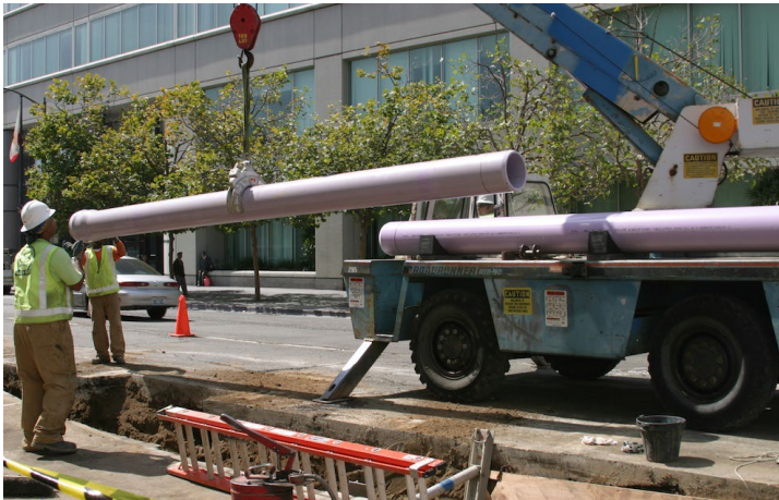
Recycled Water Pipeline
