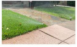
**2) After** photos showing all sprinkler nozzles within the irrigation zone have been converted to high-efficiency nozzles.
