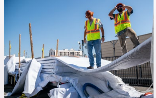
Flexible liners strengthen aging wastewater pipelines.
