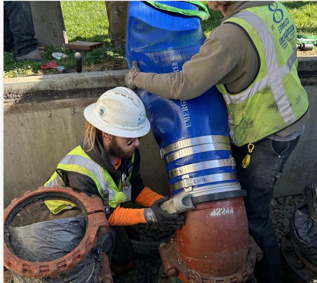
Crews practice installing a temporary bypass during an EOT exercise.
