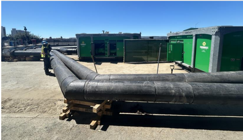
Bypass Pumping in Emeryville During Construction
