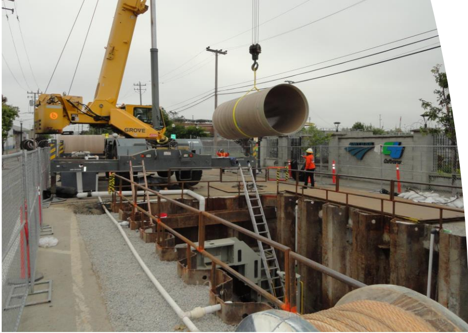
South Interceptor Rehab 3rd St.
