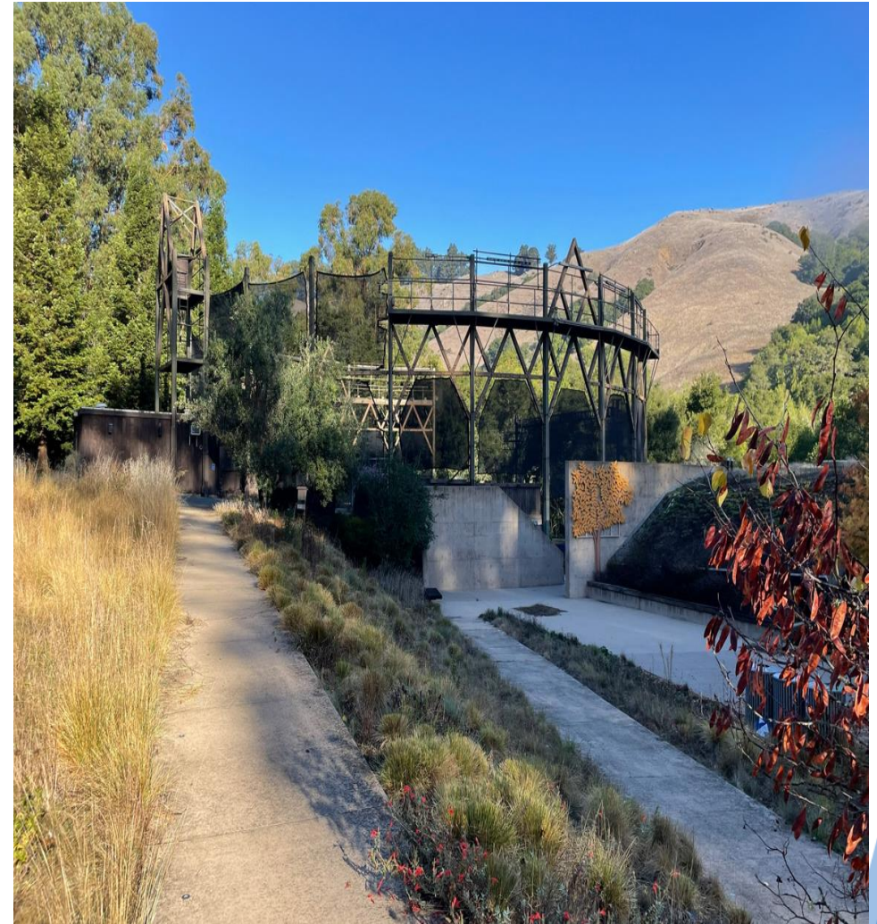
Photo of Theatre Structure
