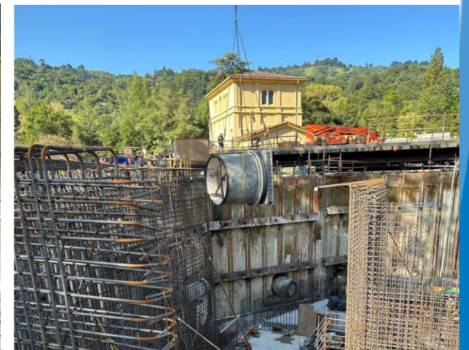
UV and CCB Structure Rebar and Piping
