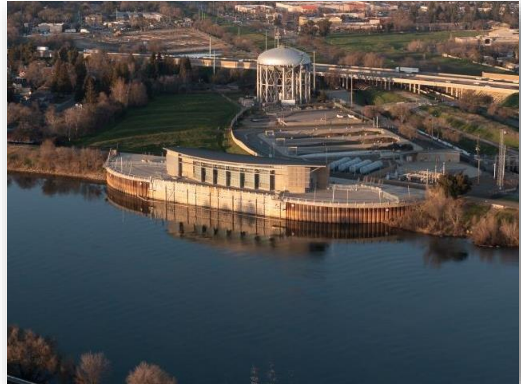
Freeport Regional Water Project Intake, Sacramento River Photo Credit: Freeport Regional Water Authority
