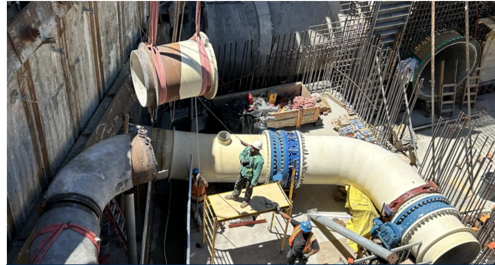
Contractor setting a section of 36-inch pipe in the UV/CCB
