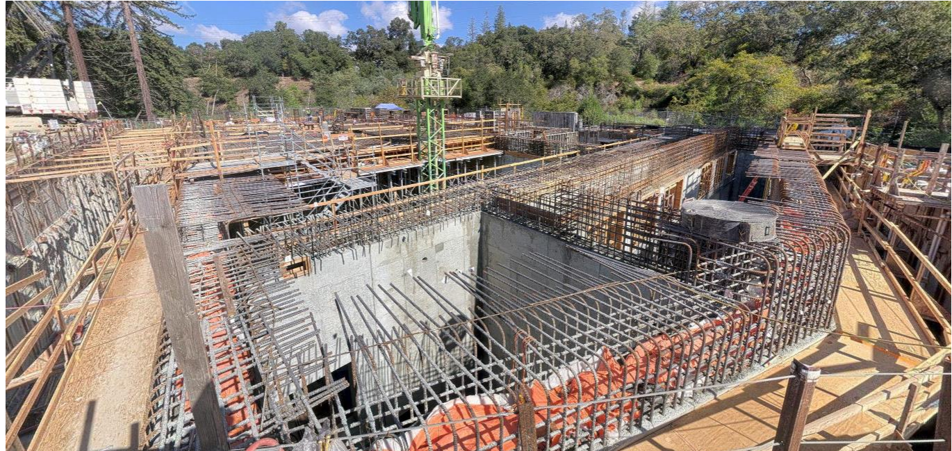
UV/CCB Construction at Ground Level (structure continues 65-feet below ground)
