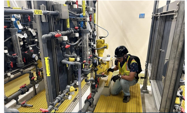
Stantec Project Engineer checks equipment for a submittal review
