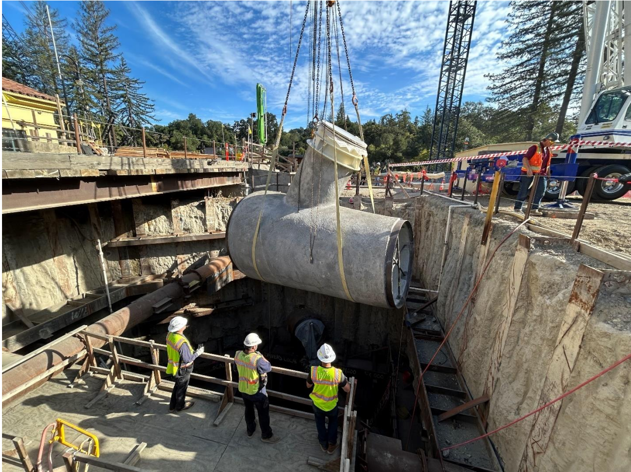
Figure 33 - Lowering the 9-foot diameter steel piping connector piece (wye) which connects the 9-foot diameter UV Influent piping to the 4-foot diameter Effluent 1 and 6-1/2-foot diameter Effluent 2 tunnels.
