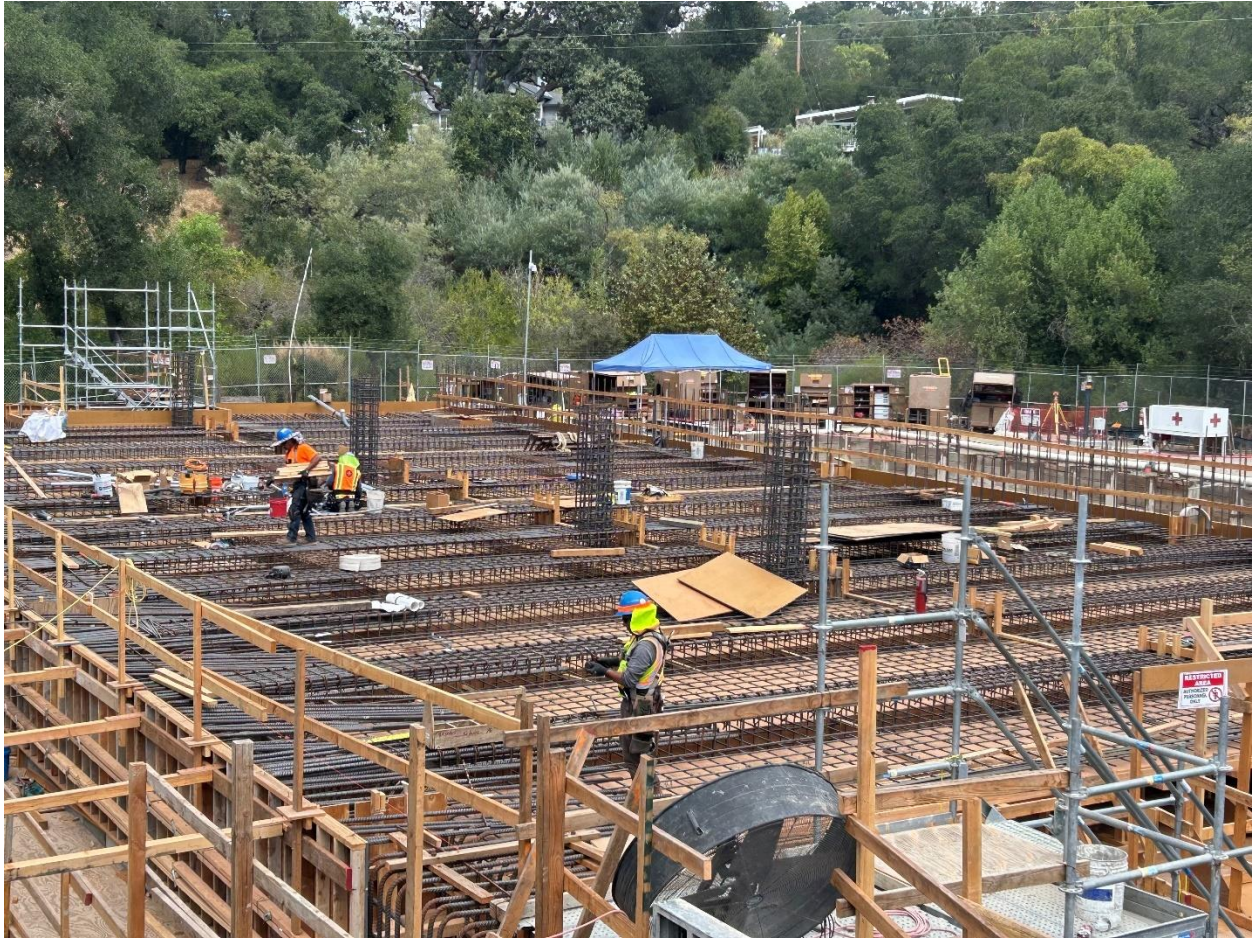
Figure 15 - Installation of formwork and reinforcing steel for the CCB Room roof deck. This deck will serve as the ground of the future ground floor for the MAUVE building.
