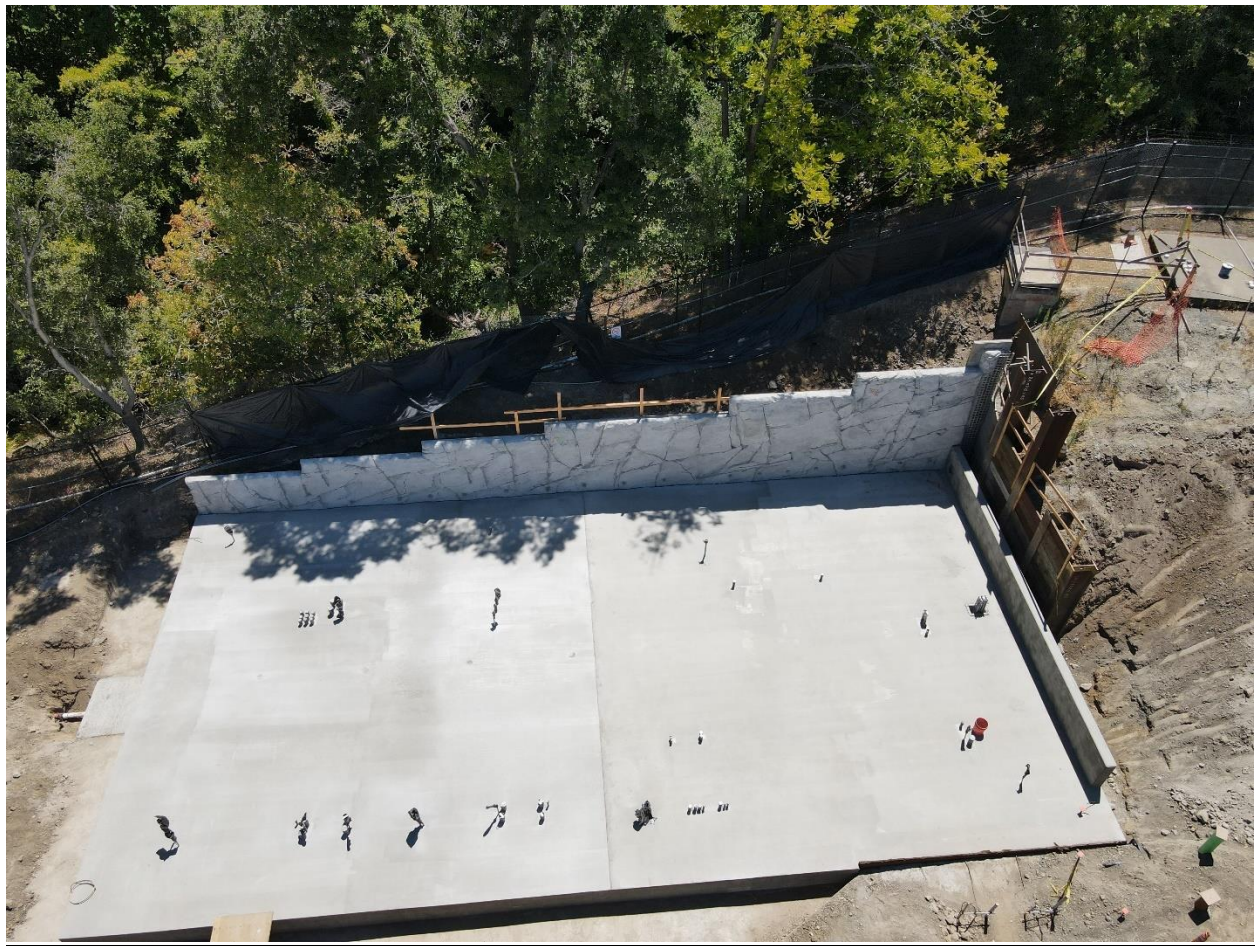
Figure 27 - Aerial view of the completed South Electrical Building (SEB) foundation.
