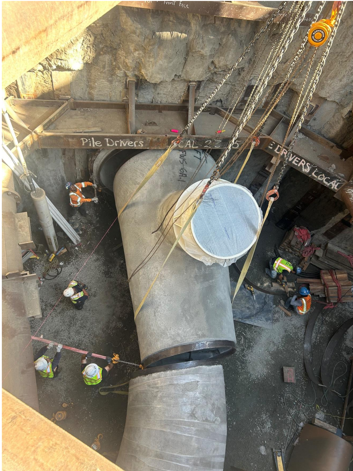
Figure 34 - Pipefitters using complex crane slings and mechanical devices to position the massive wye into alignment with the tunnels in the Effluent 1 excavation.
