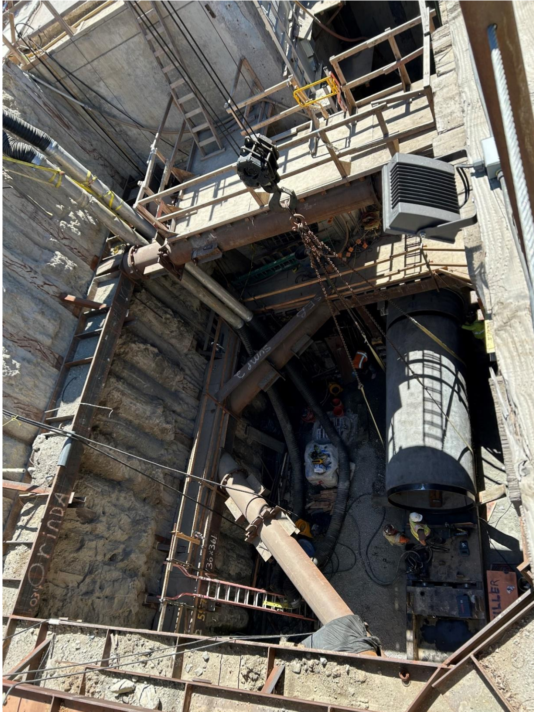
Figure 32 - View looking down into the 45-feet deep Effluent 1 shored excavation. Pipefitters using a crane to lower a 6-1/2-foot diameter steel pipeline segment the pit.
