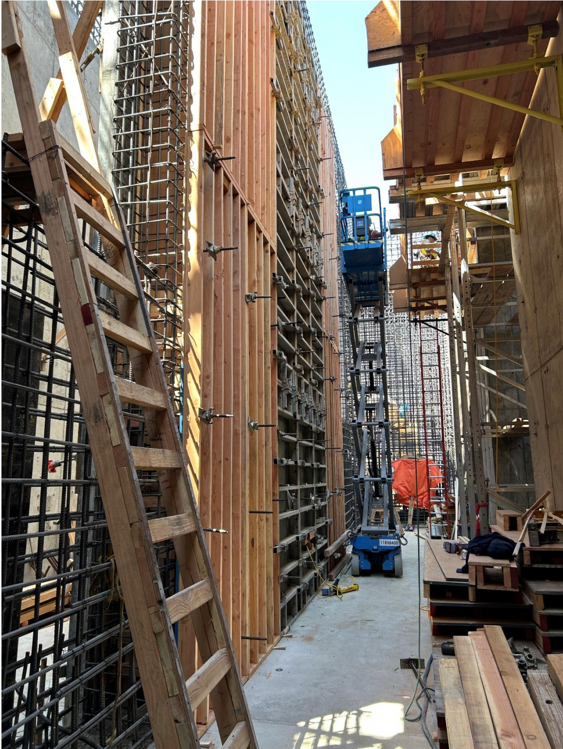
Figure 20 - Workers on blue scissor lift installing concrete wall forms for the Effluent Weir Structure.
