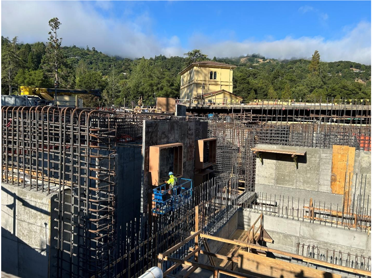
Figure 19 - Workers installing wall block-outs in the Effluent Weir Structure for the weir gates which will control the hydraulics of the water treatment plant.
