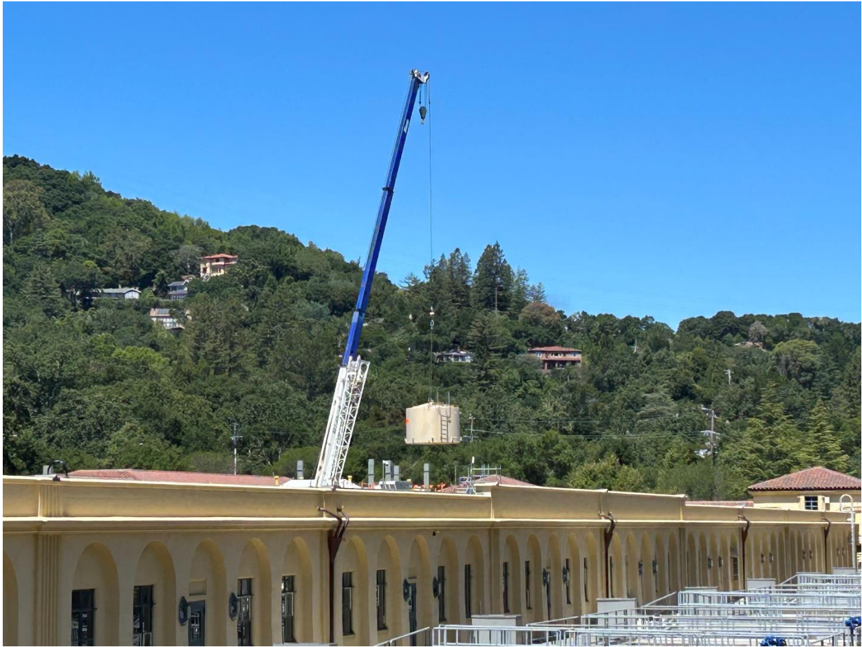
Figure 37 -- Crane lowering new fiberglass reinforced plastic chemical tank into the Chemical Building through the new roof opening.
