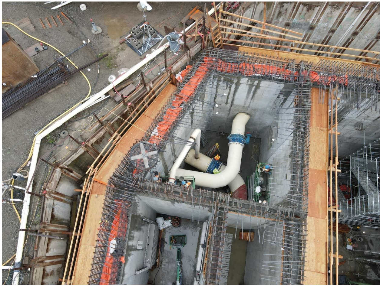
Figure 24 - Aerial view looking down into the nearly complete Valve Vault.
