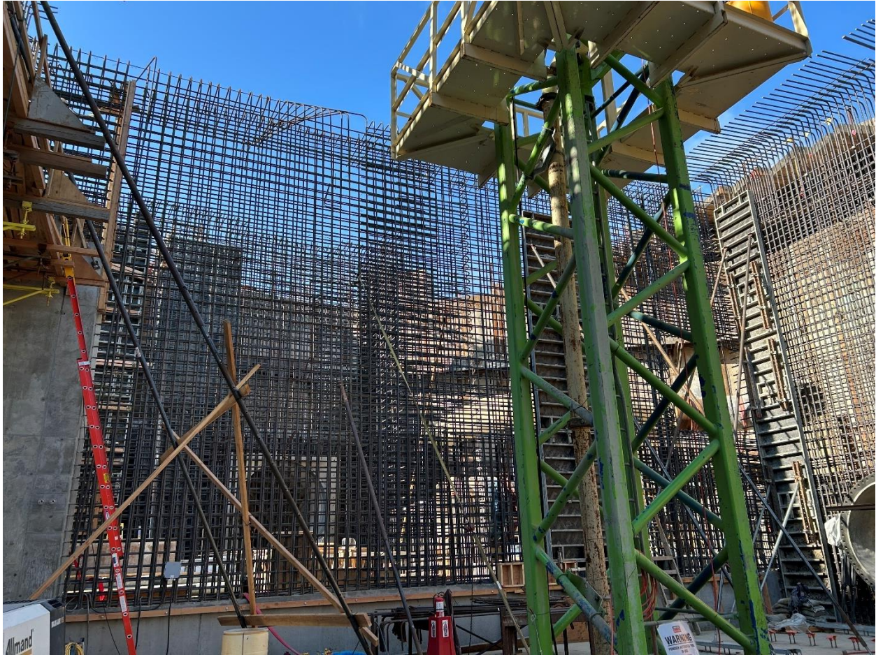
Figure 11 - Reinforcing steel for the divider wall between the UV Room and Effluent Weir Structure prior to installation of formwork.
