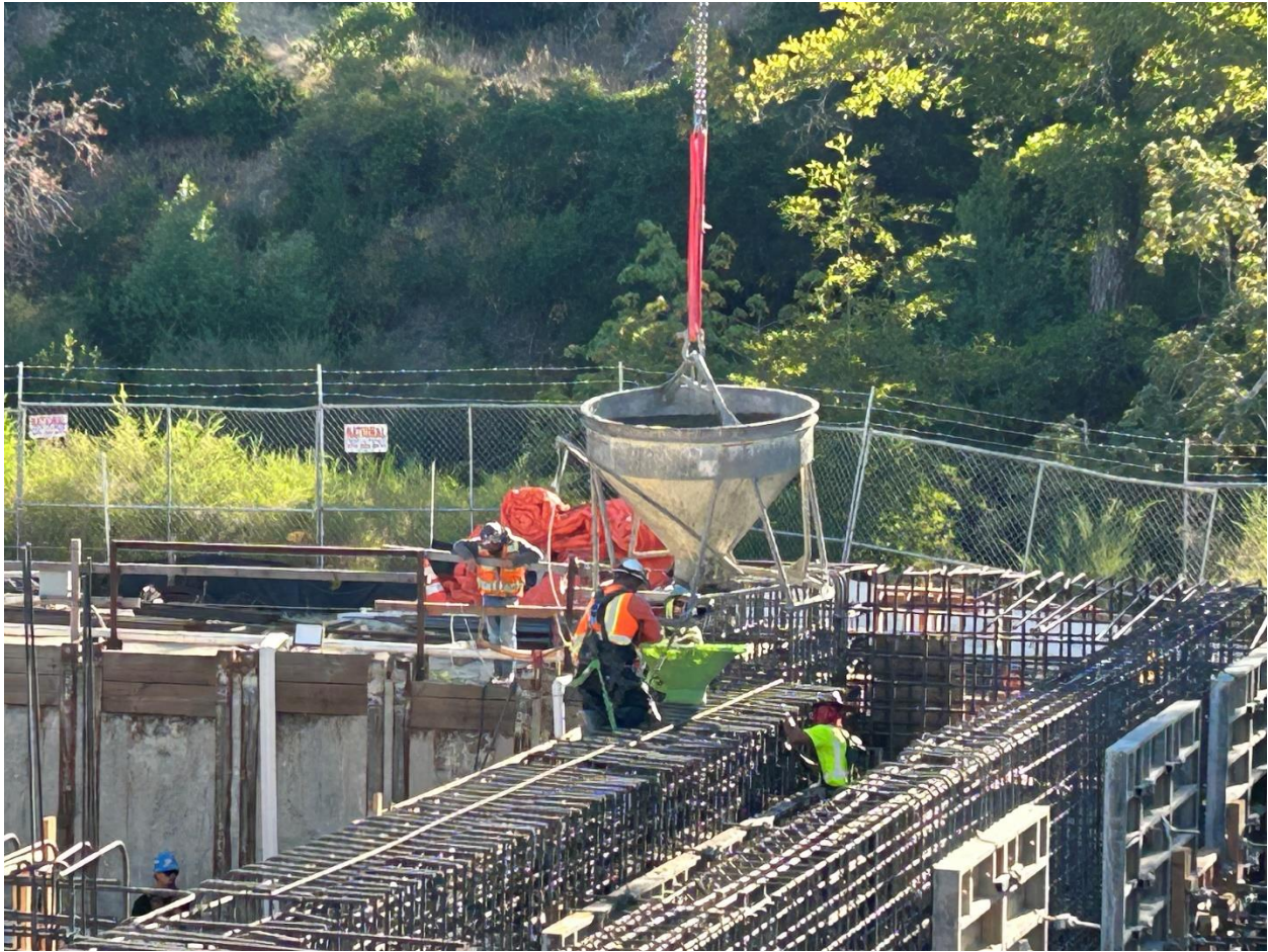
Figure 21 – Placement of concrete using a concrete bucket suspended by the 210-foot tall tower crane. The contractor uses the bucket for pouring "smaller" amounts of concrete.
