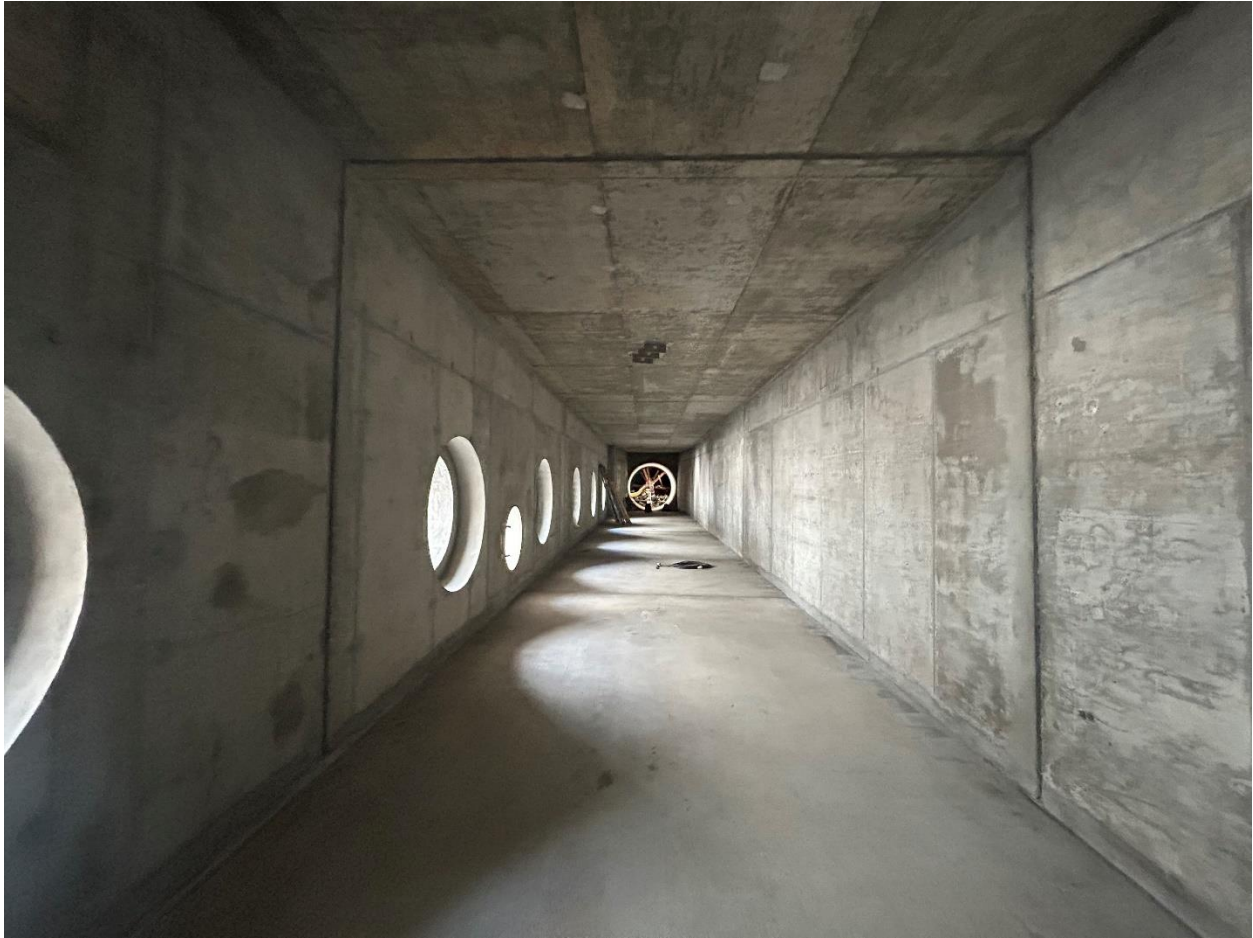
Figure 25 - View looking down the inside length of the Influent Weir Structure. This structure is undergoing leak testing for watertightness prior to being backfilled
