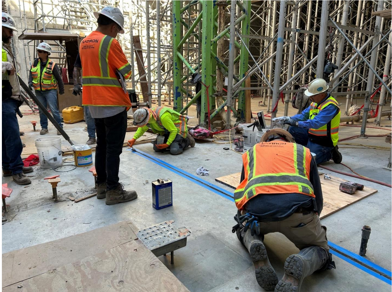
Figure 14 - Workers starting the installation of the joint sealant between concrete floor slabs in the UV Room.
