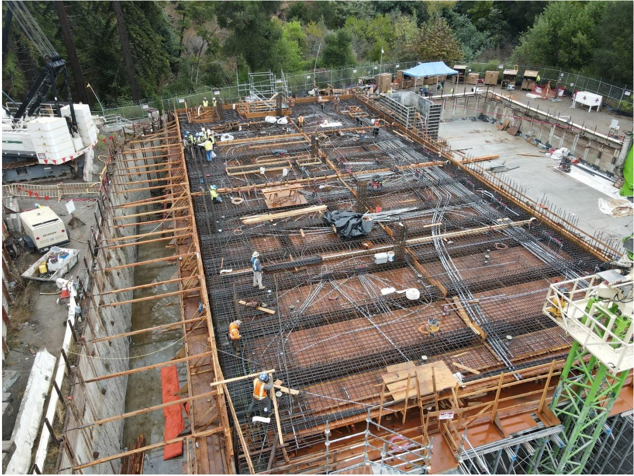
Figure 16 - Installation of embedded conduits, plumbing, and equipment anchors for the MAUVE floor.
