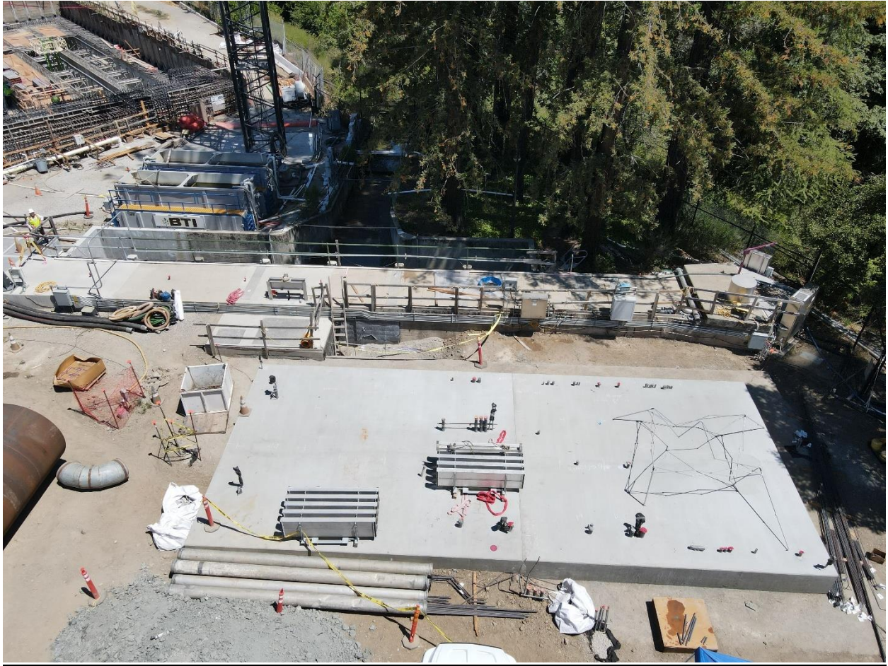
Figure 26 - Aerial view of the completed foundation for the Los Altos Power Building (LAPB).
