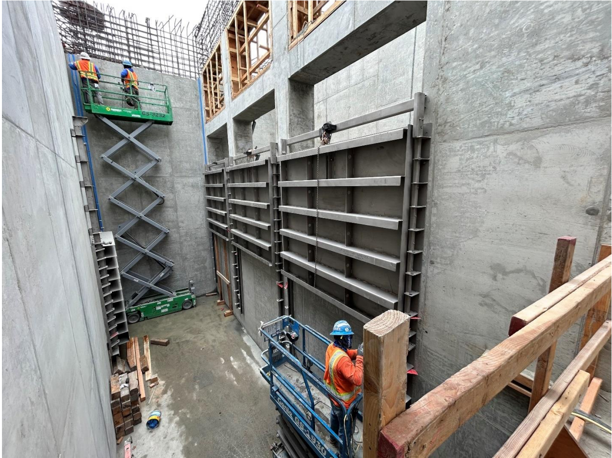
Figure 22 - Workers on scissor lifts installing the weir gates in the partially completed Effluent Weir Structure.
