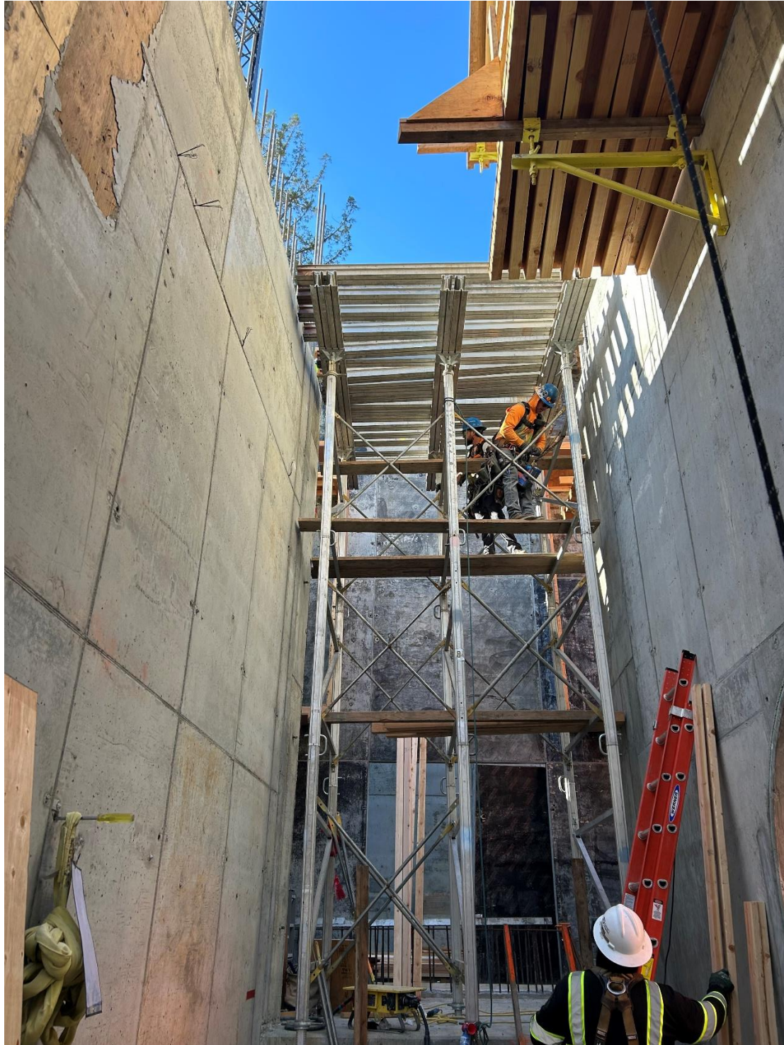
Figure 2 -- Installation of the scaffolding towers for the CCB roof. These towers support the concrete formwork as concrete is placed and cured.
