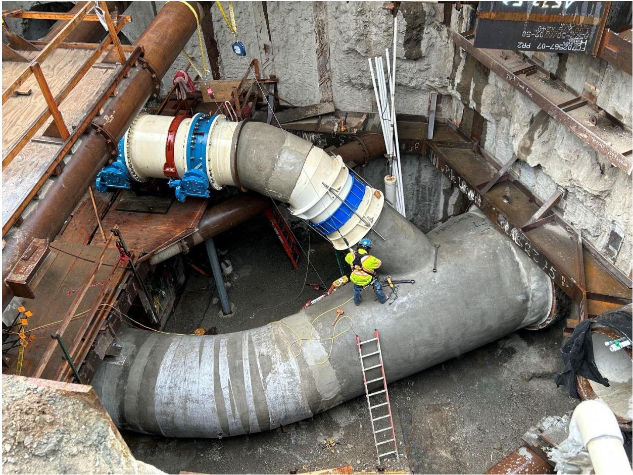
Figure 35 – The photo shows a pipefitter standing on the 9-foot diameter wye connector piping from Effluent 2 to Effluent 1. The pipefitter is making final mechanical connections on the wye after completion of all welded joints and mortar corrosion protection on the steel piping.
