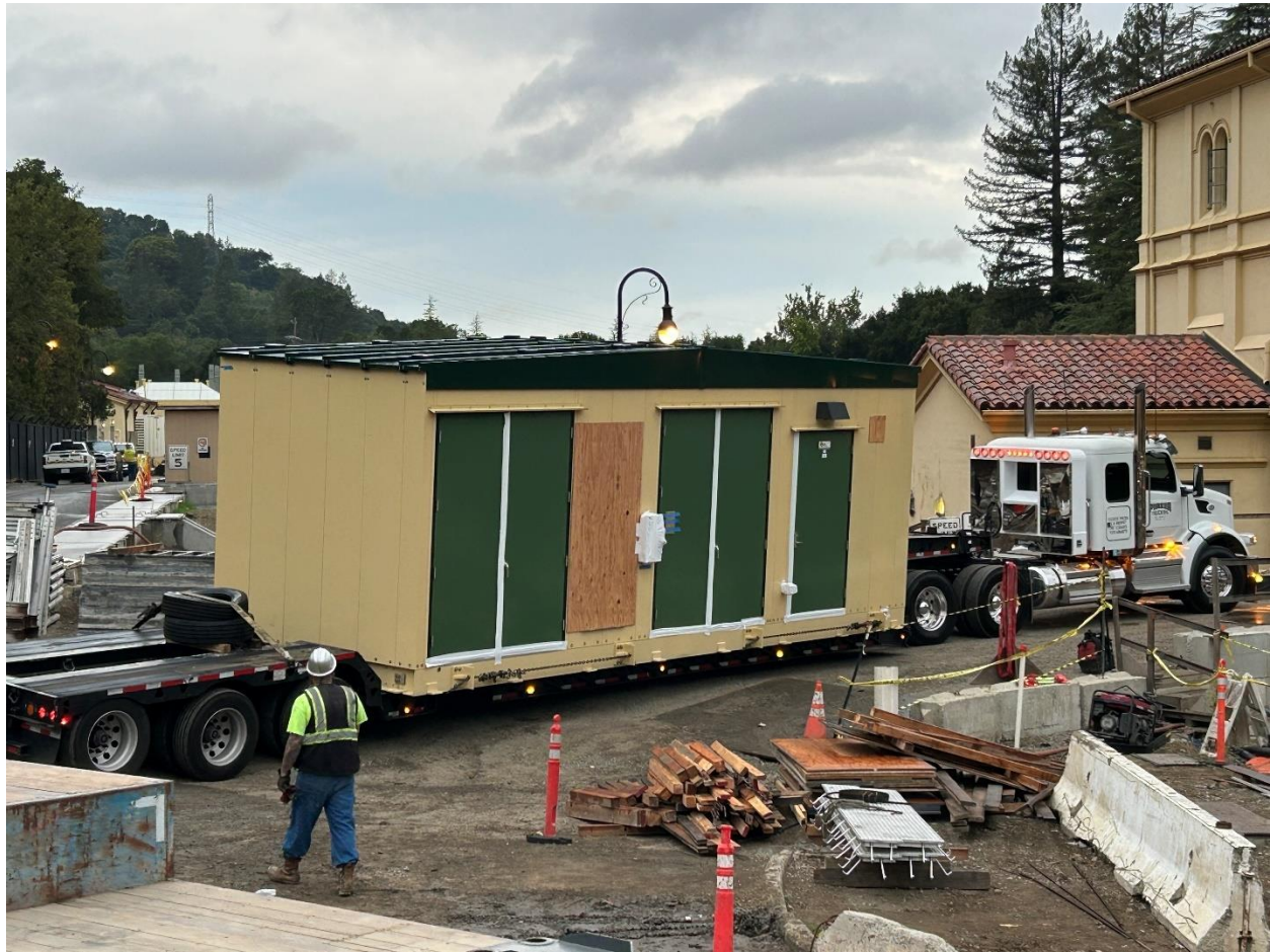
Figure 29 – Worker assisting truck as it backs one of seven SEB building segments into place for the crane to lift it into place.
