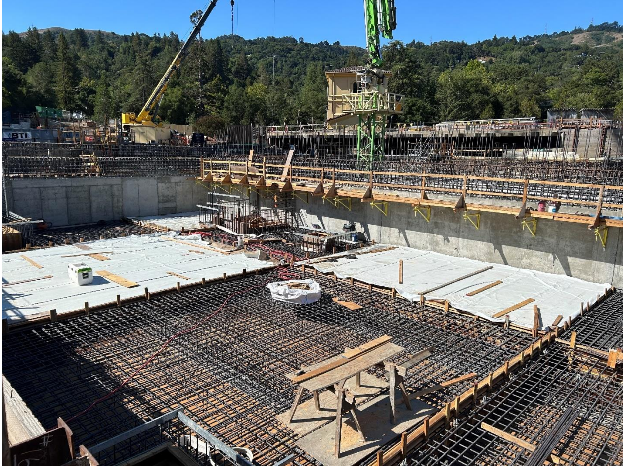
Figure 6 – Partially completed CCB roof. The photo shows rebar supported on wooden formwork and completed concrete slabs. The concrete is cured under the white blankets which control the environmental conditions.
