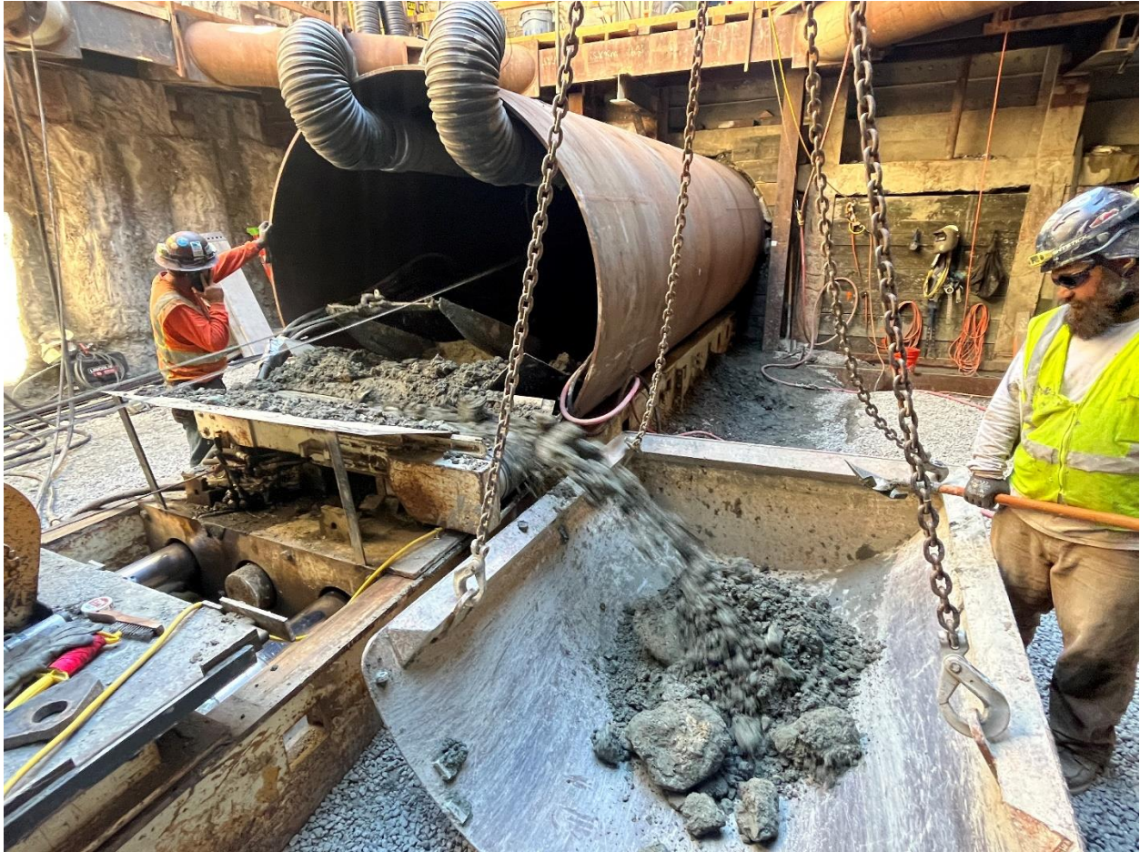
Figure 31 - Tunneling through the ground 45-feet below the ground surface of the water treatment plant. Mine tailings being ejected out of the end of the 90-inch steel tunnel casing for installation of the steel pipeline from the filter Effluent pipelines.
