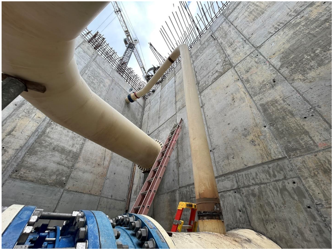
Figure 23 - View looking up from the floor in the Valve Room.
