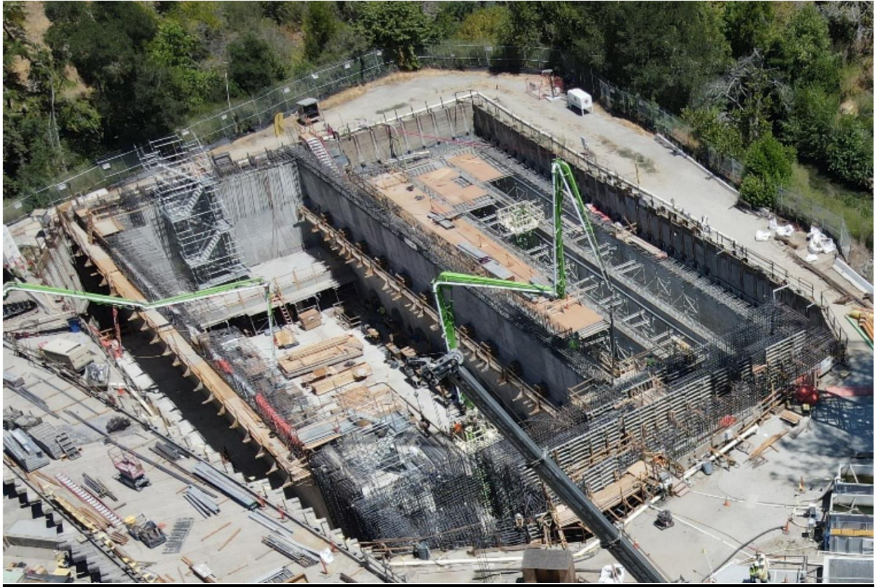
Figure 4 –Concrete placement via concrete pump truck for the last 25-foot tall walls for the CCB.
