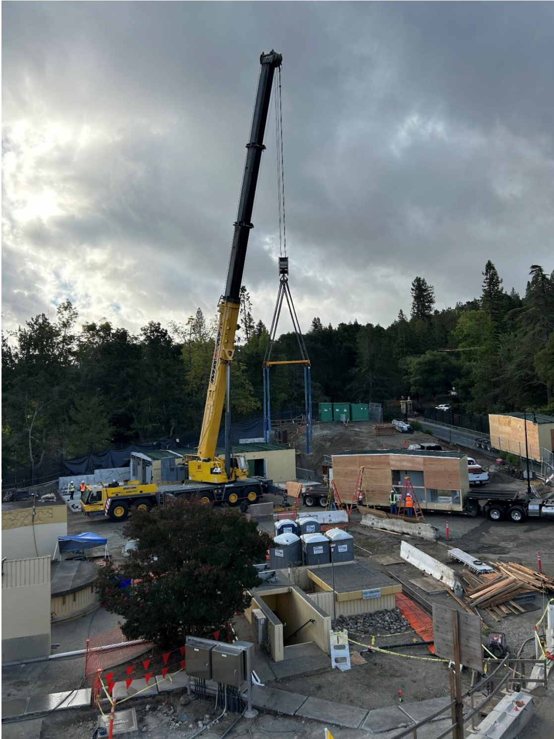
Figure 28 – Installation of pre-fabricated SEB section on the right side of the photo.
