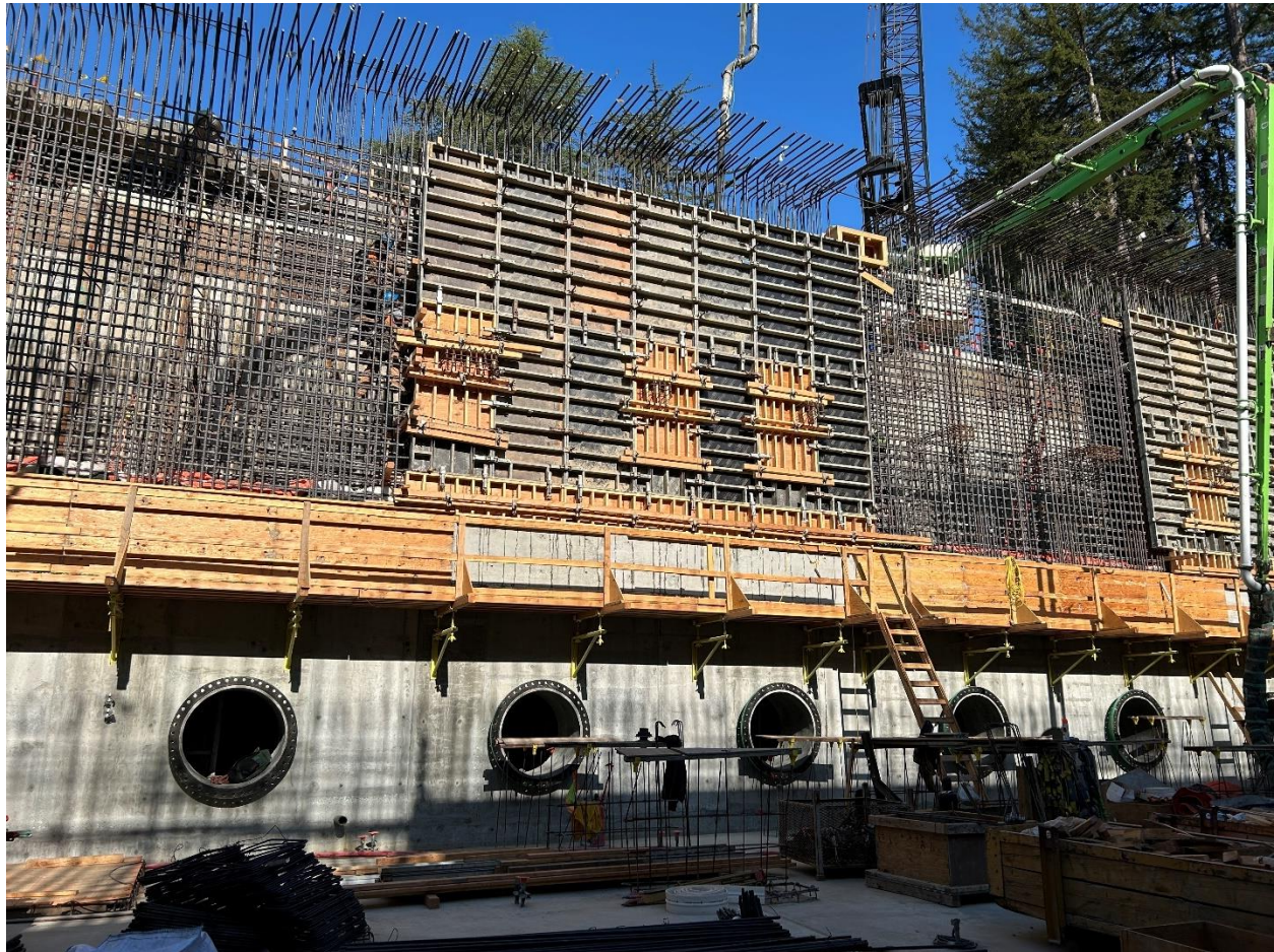
Figure 9 - Partially completed wall in the UV Room.
