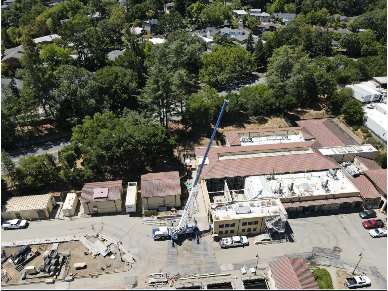
Figure 36 - Crane lifting structural steel beams into openings in Chemical Building roof.
