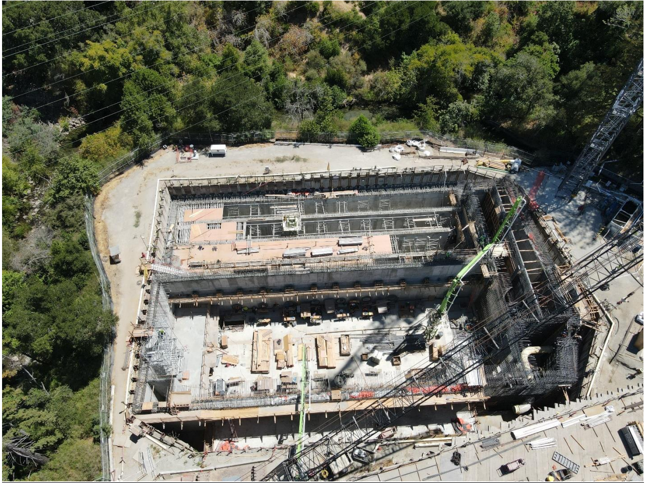
Figure 1 -- Aerial View of underground UV-CCB Structure with Influent Channel in the foreground, UV Room in the midground, CCB in the background, Effluent Weir Structure in the upper right, and Valve Room in the lower right.
