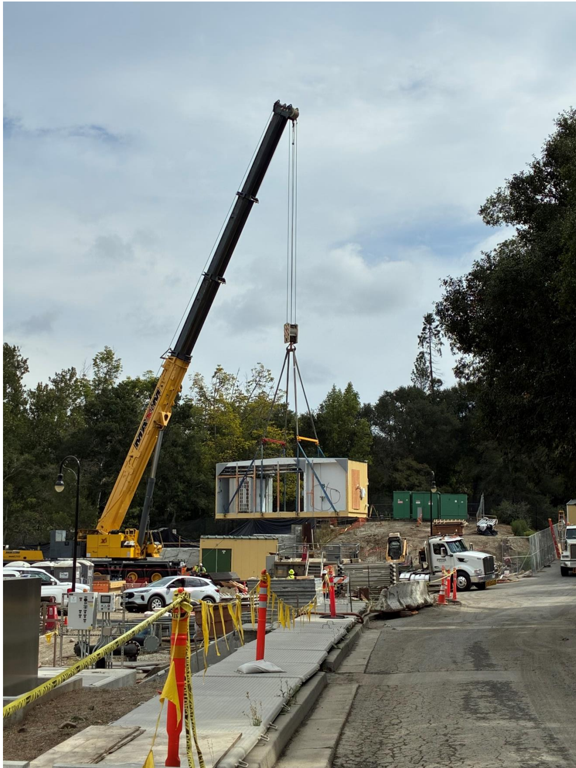
Figure 30 - Crane lifting a SEB segment off the delivery truck onto its new foundation using complex sling support system.
