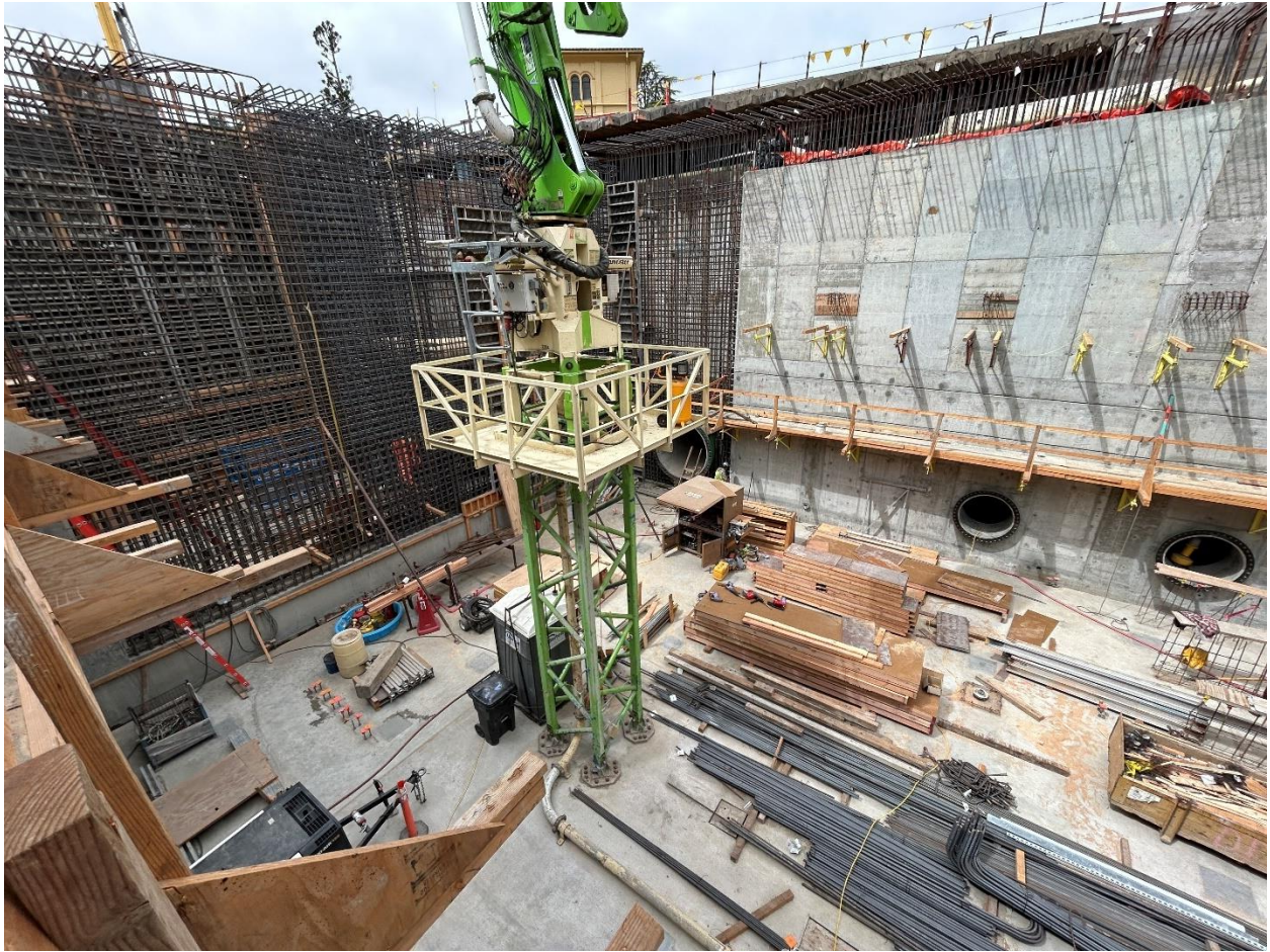
Figure 10 - The concrete wall from Figure 9 is shown as completed in this photo.
