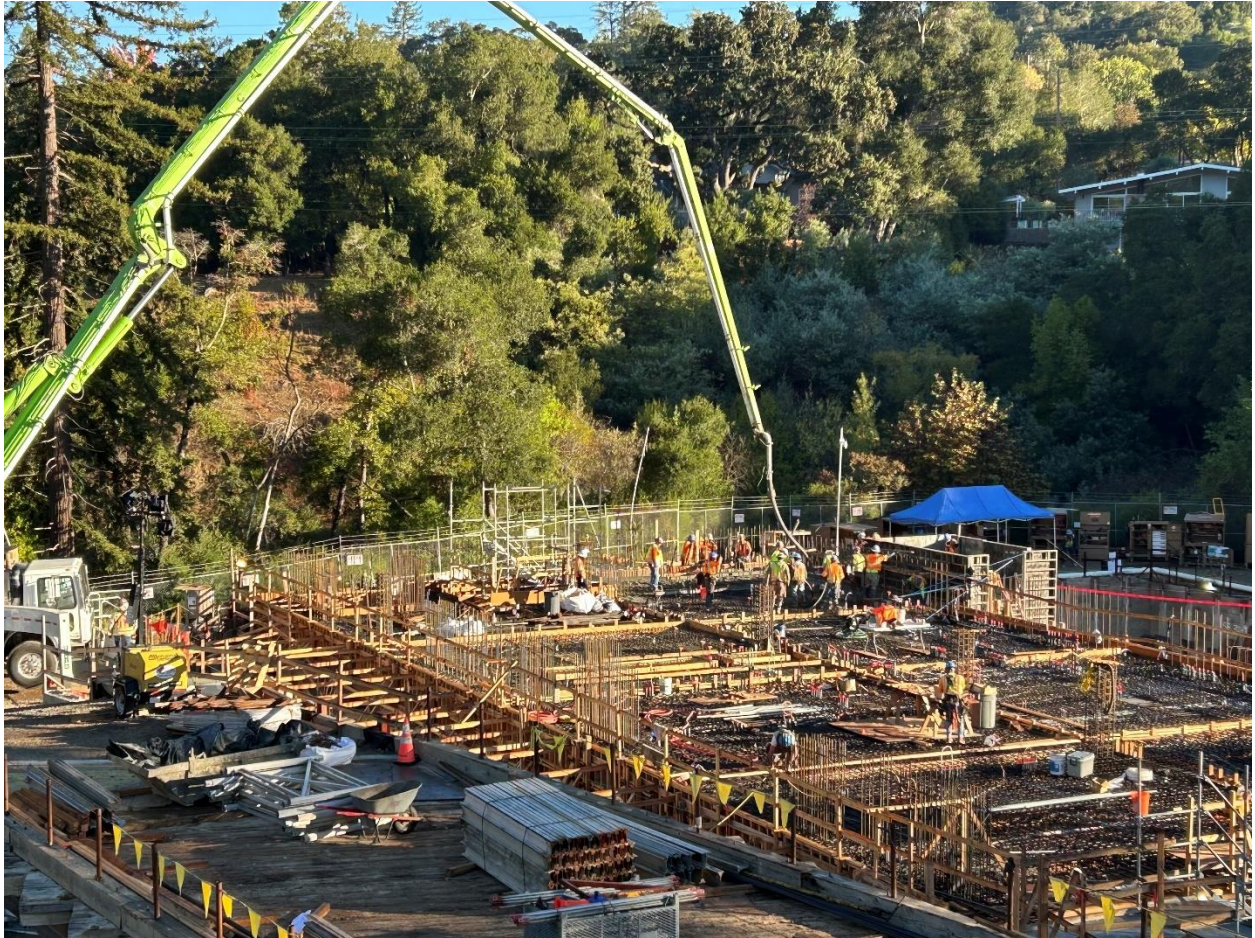
Figure 18 – Installation of the first concrete for the MAUVE floor with the aid of the articulating boom and concrete pumper truck.
