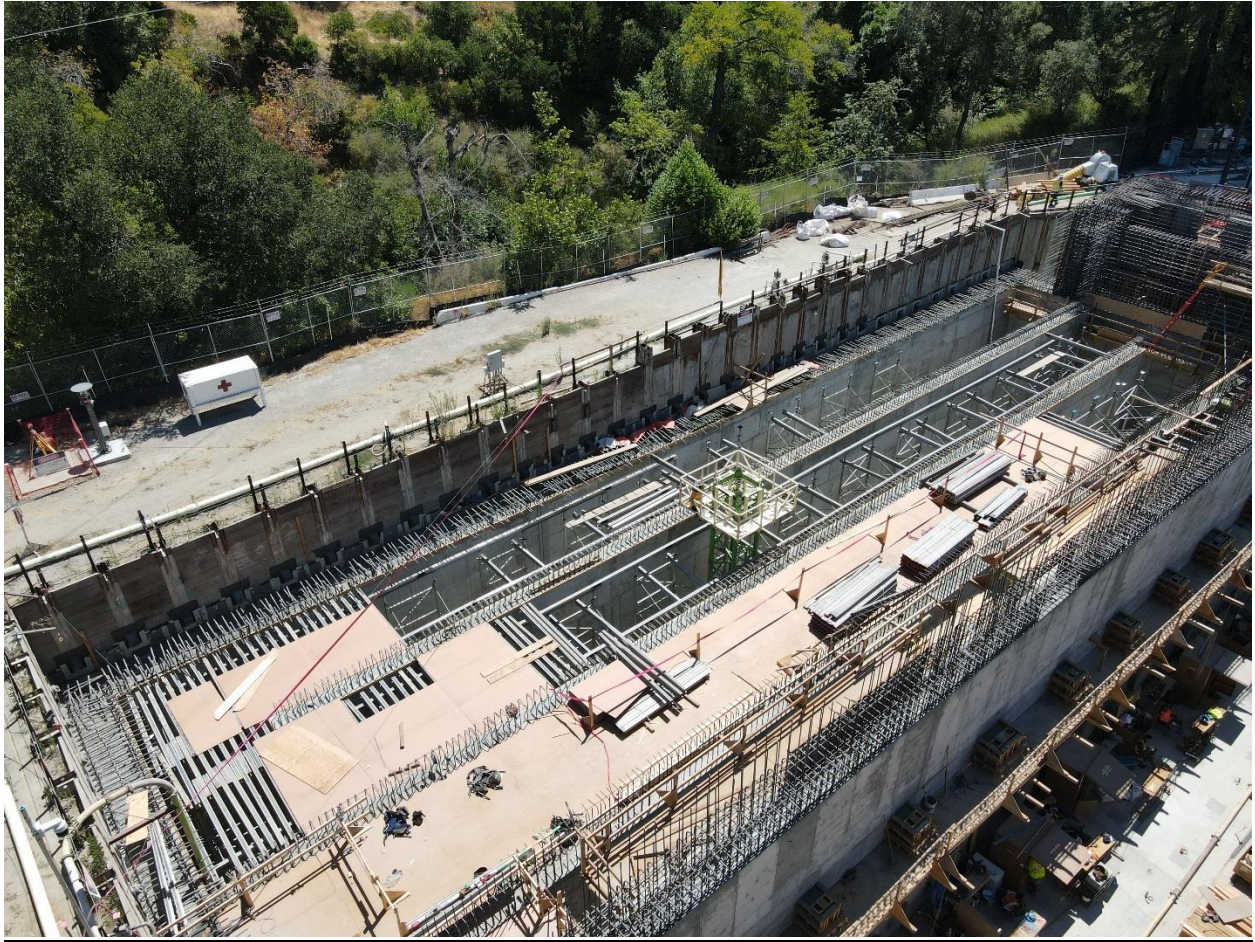
Figure 3 -- Aerial view of the CCB with shoring towers and formwork for the partially completed CCB roof.
