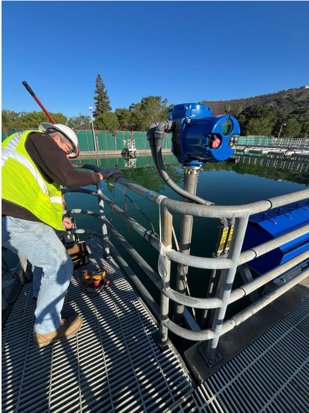
Figure 2 – North Sedimentation Basin –sedimentation basin testing for return to service
