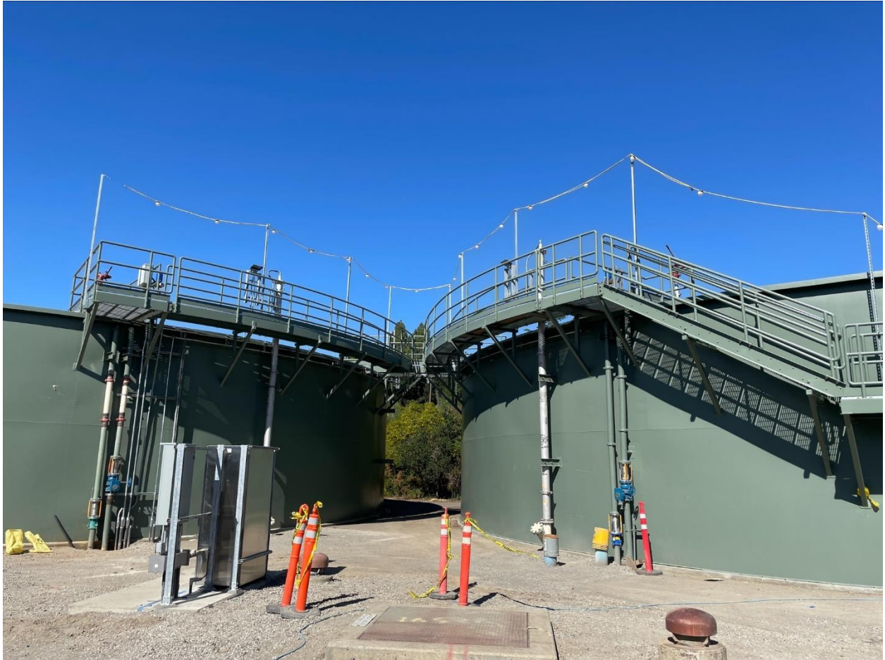
Figure 9 – Newly recoated Detention Basin No. 1 and 2 exterior
