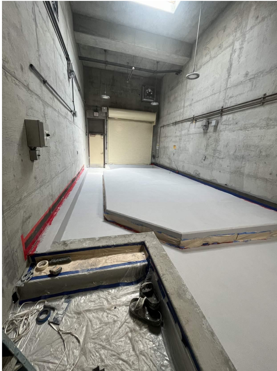
Figure 14 – USL WTP chemical system coagulant storage room tank pad completed
