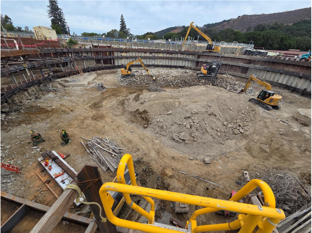
Figure 5 – Old Chlorine Contact Basin structure complete demolition
