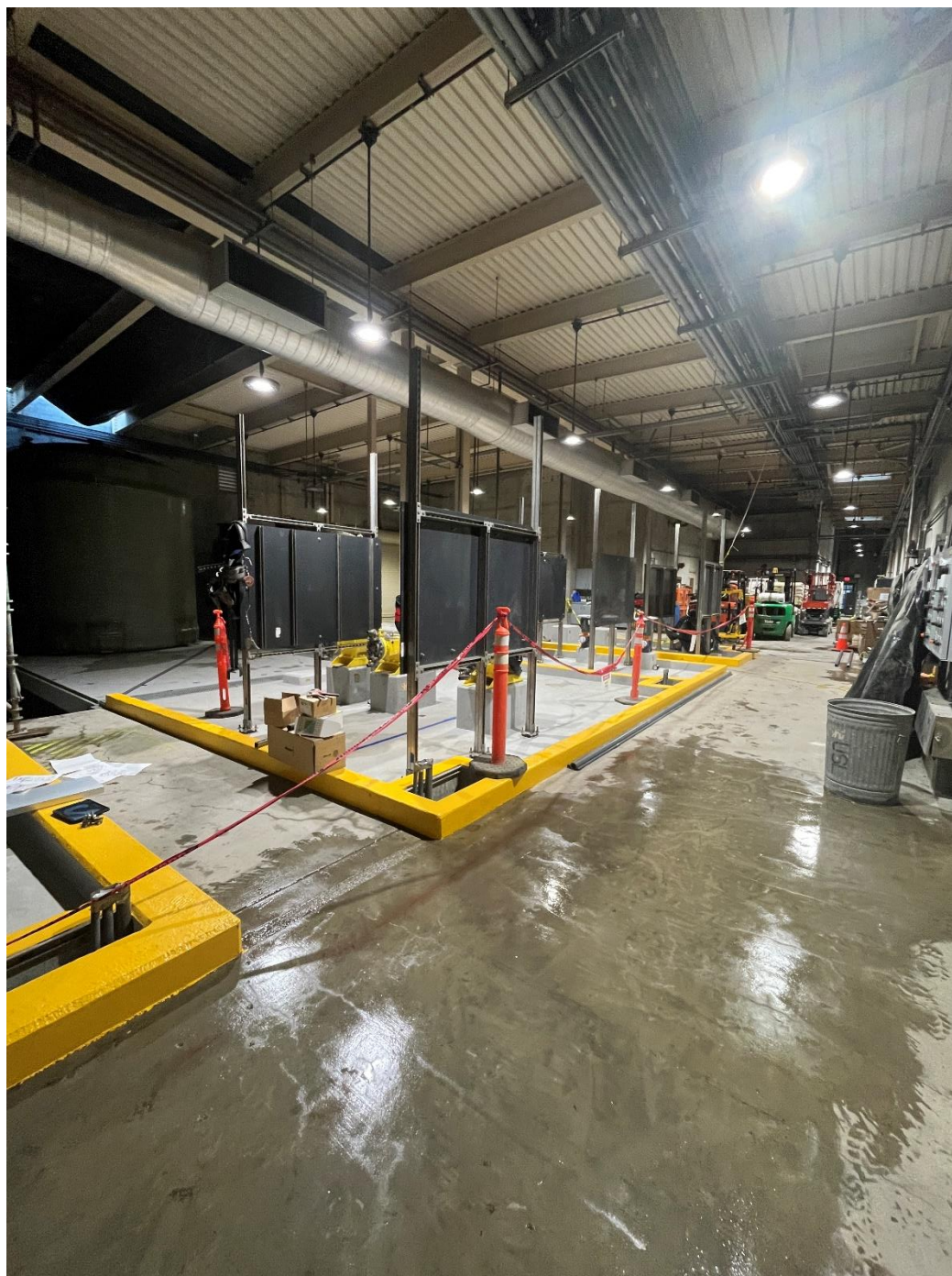
Figure 12 – USL WTP chemical area preparing for permanent chemicals
