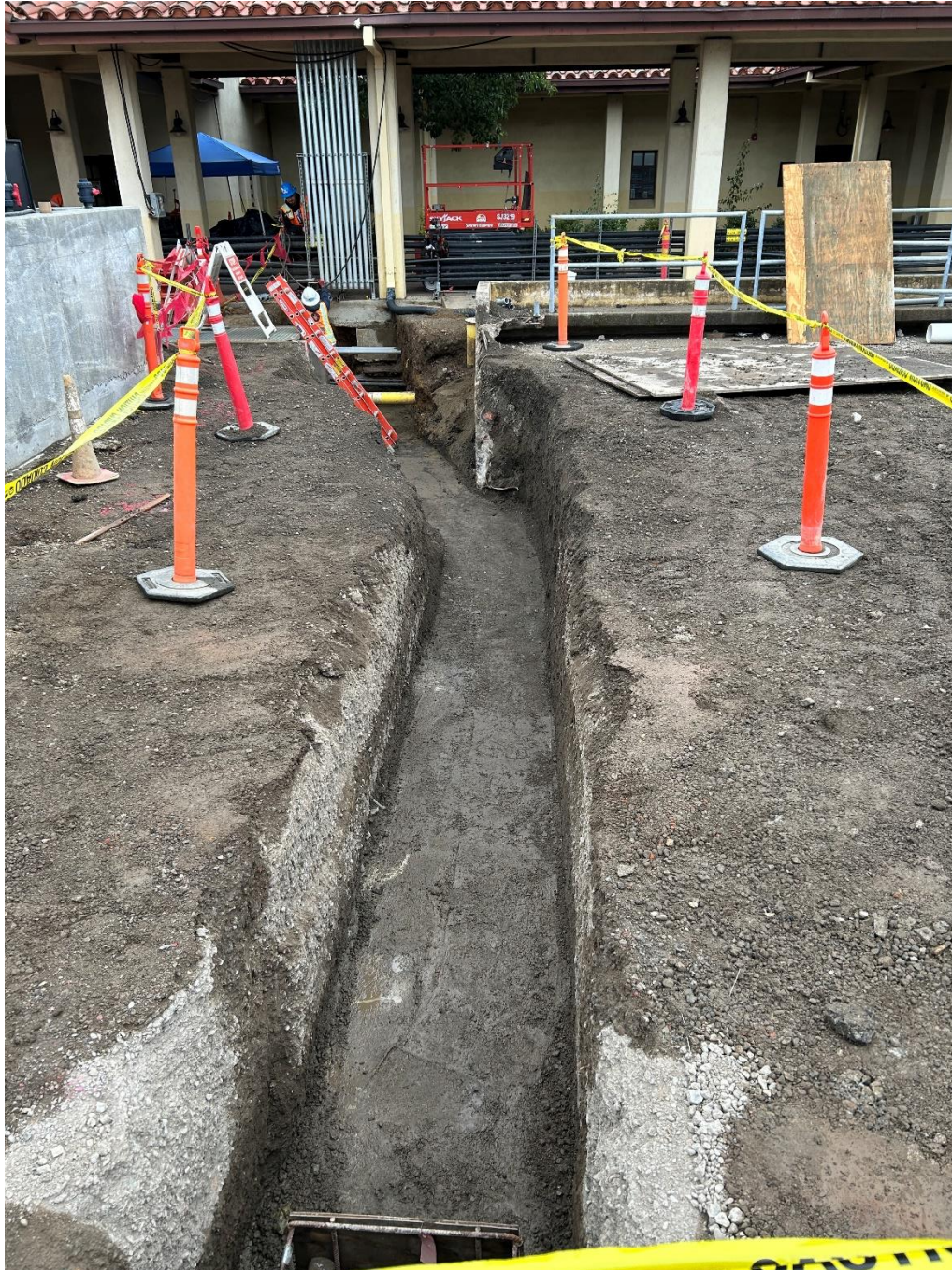
Figure 6 – Electrical duct bank installation preparation
