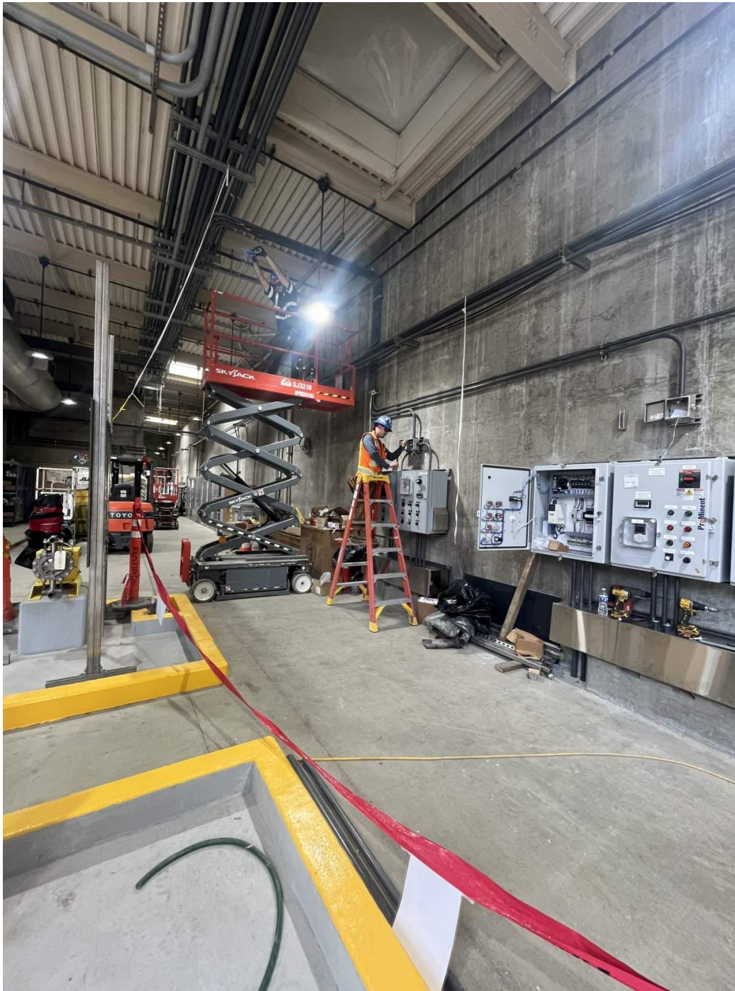
Figure 13 – USL WTP chemical area electrical sub pulling wire for new electrical controls
