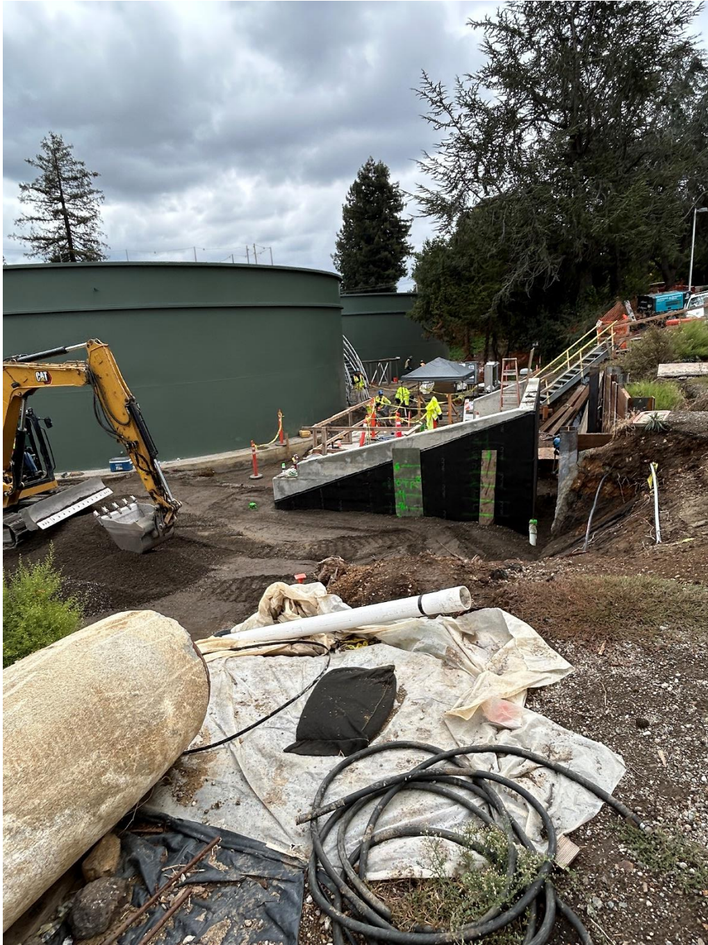
Figure 7 – Reclaim area vault construction completion and backfill
