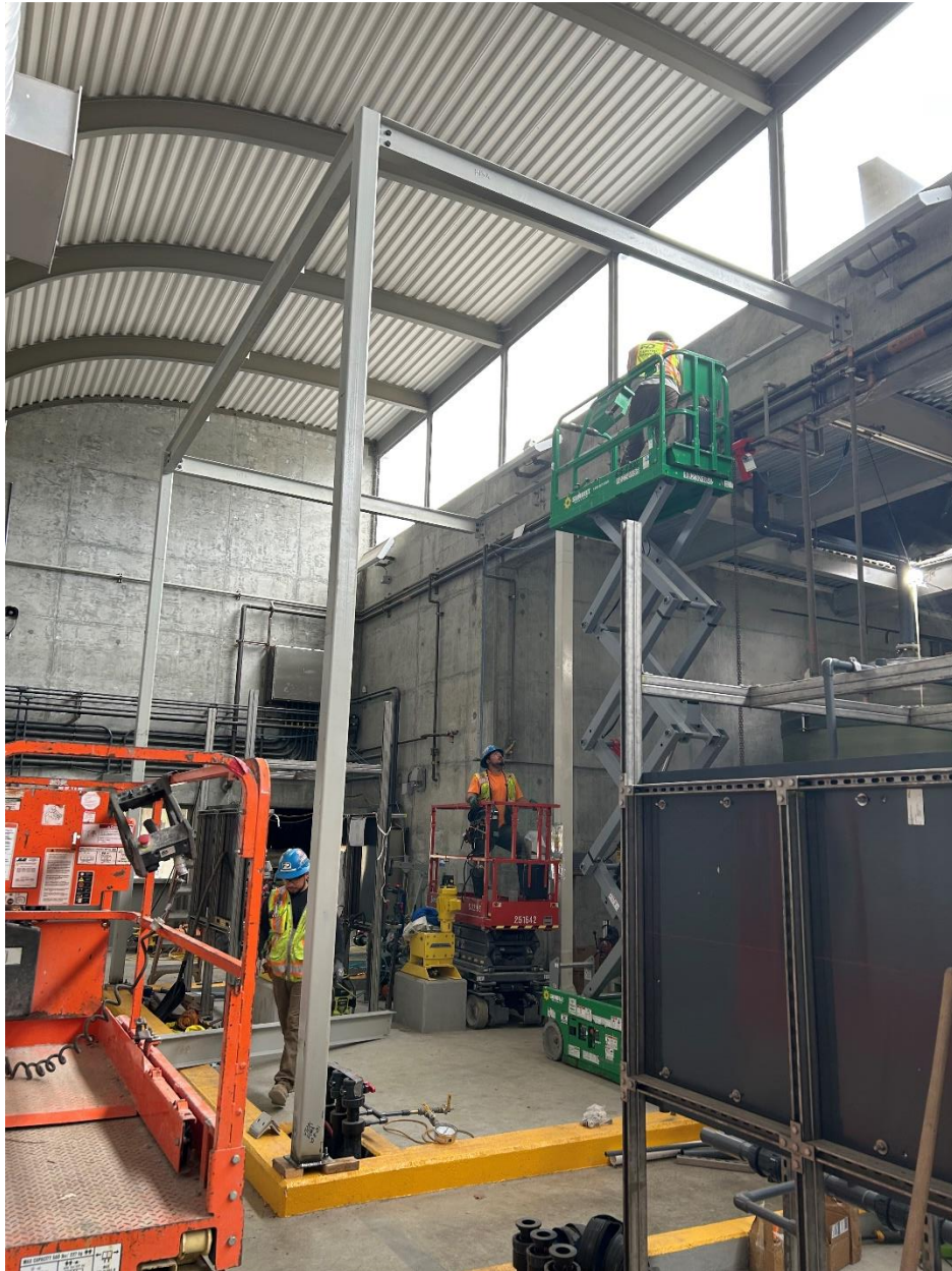
Figure 17 – Sobrante WTP Installation of new conduits
