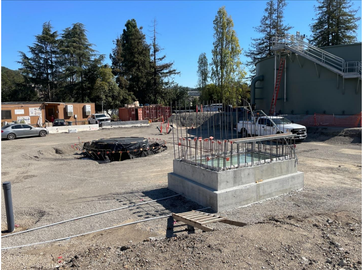
Figure 10 – Installation of Gravity Thickener Center Ring, Foundation, and Subgrade Preparation
