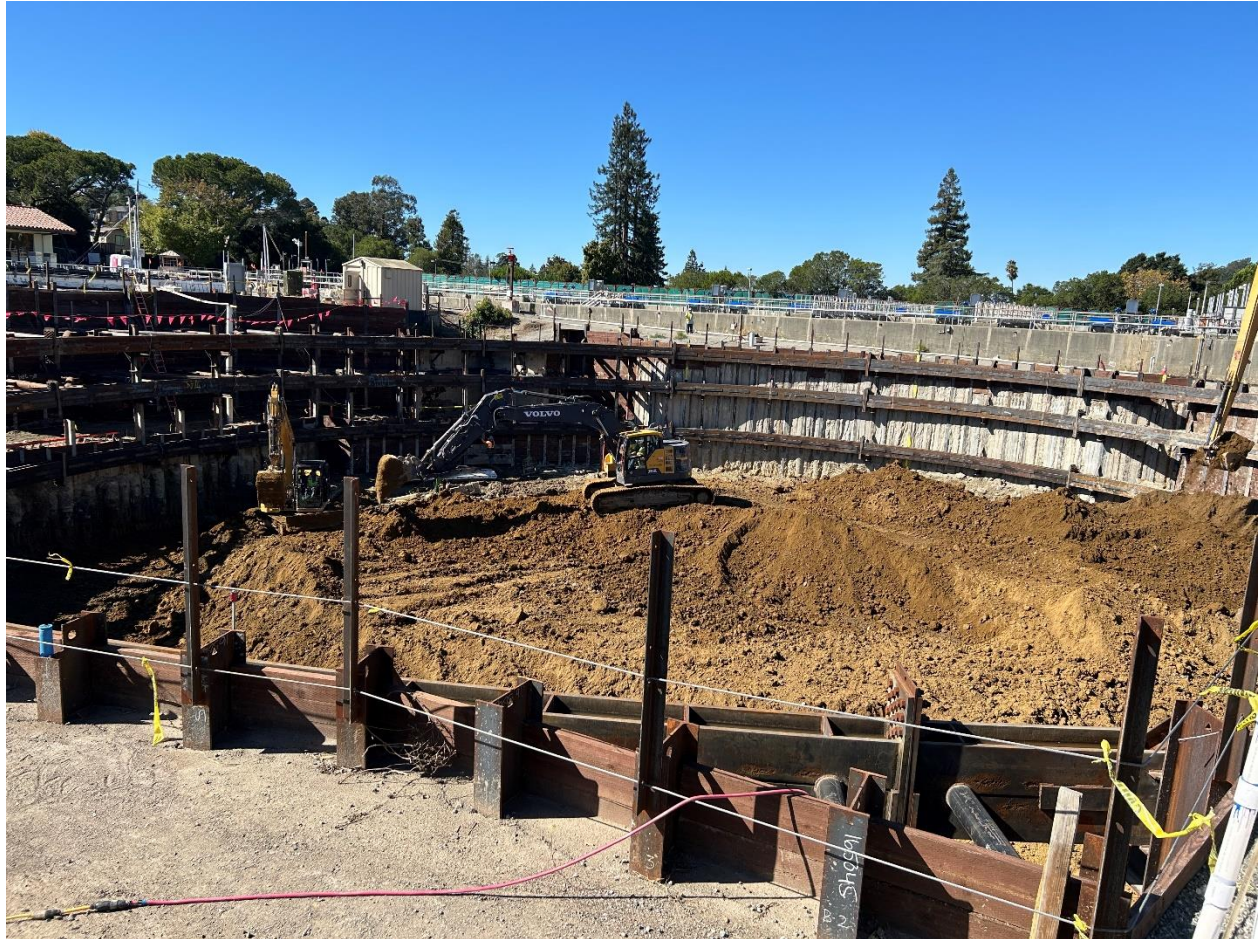
Figure 3 – Chlorine Contact Basin excavation shoring installation
