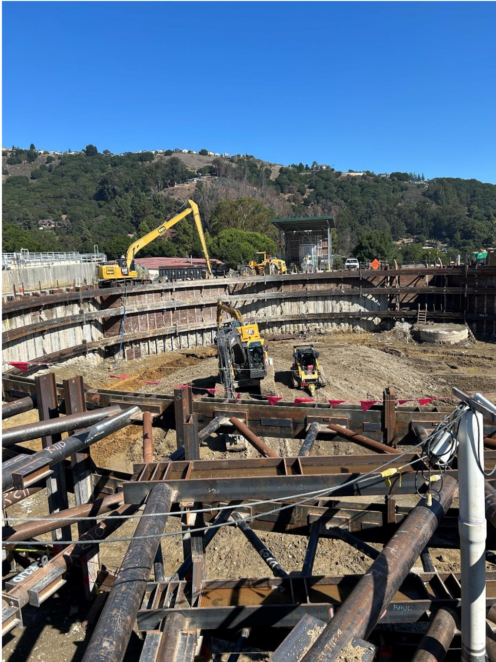
Figure 4 – Chlorine Contact Basin west side excavation bracing
