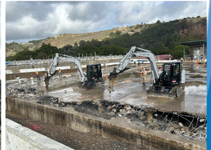
Demolish 95-year-old CCB
