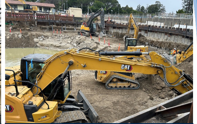
Excavation for New CCB
