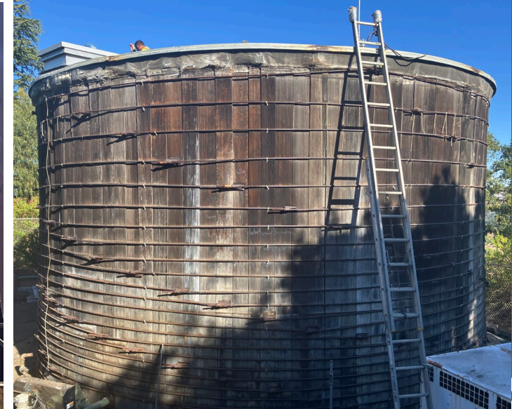
Crest Rehabilitation to be Demolished
