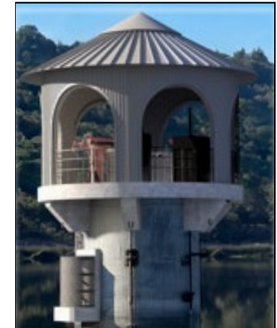
Metal Operating House
