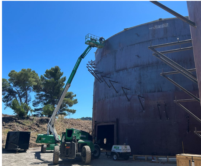
Grizzly Reservoir Rehabilitation (Welding)
