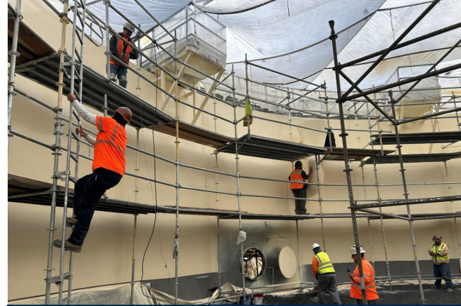
Workers Recoating Interior Tanks
