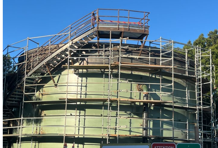
Carter Reservoir Rehabilitation (Recoating)
