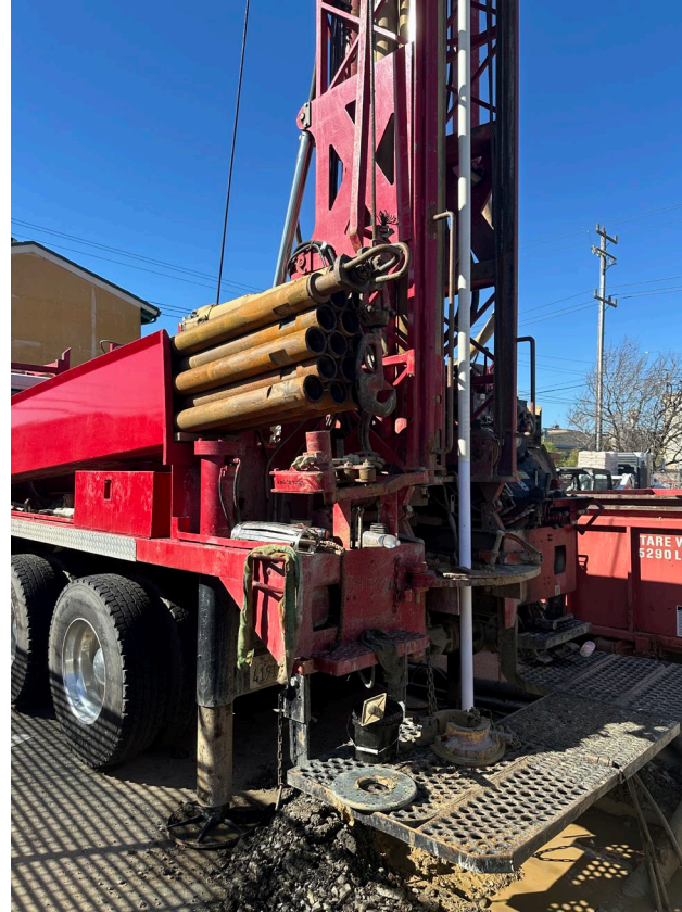
Groundwater Monitoring Well Installation
