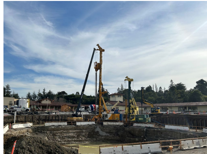
Installation of Drilled Shoring System
