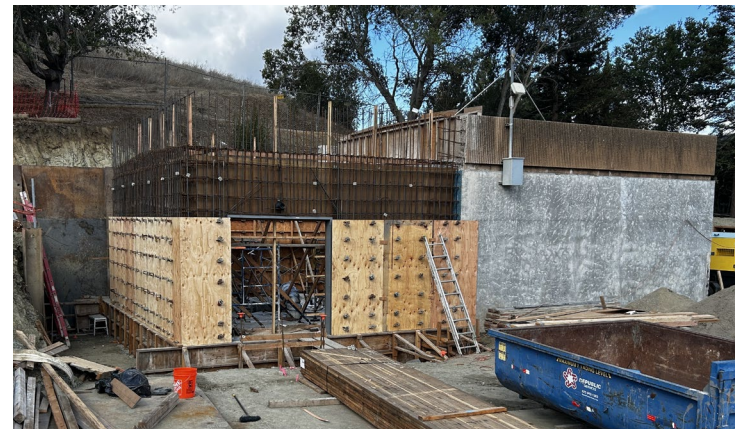
New Fay Hill PP Building Construction
