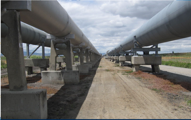
Mokelumne Aqueducts Nos. 1, 2, & 3 in the Delta
