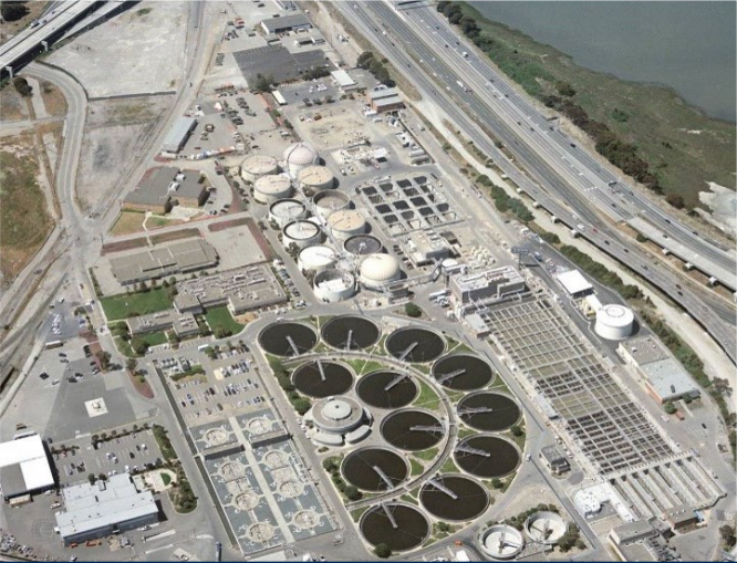
MWWTP Originally Constructed in 1951
