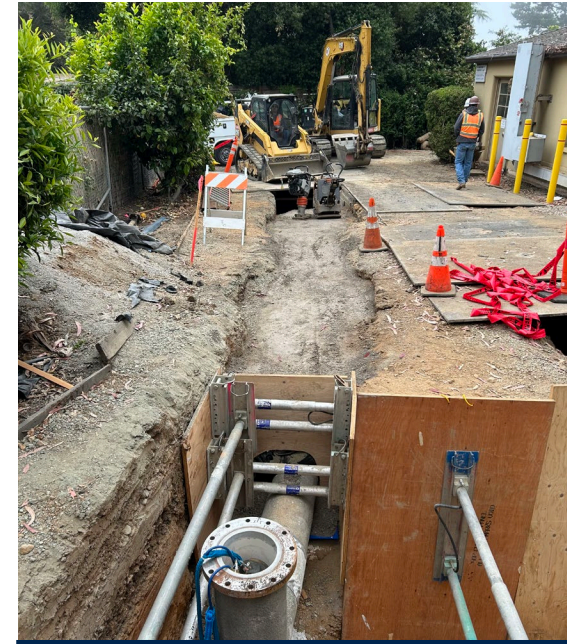
Rehabilitation of Yard Piping Palo Seco PP
