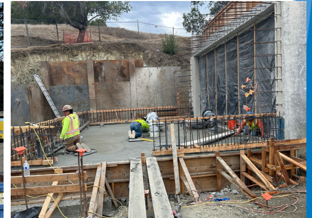
Fay Hill PP Floor Slab
