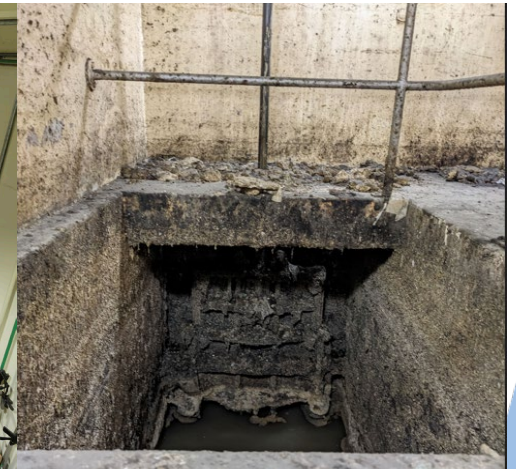
Rehabilitate Corroded Concrete
