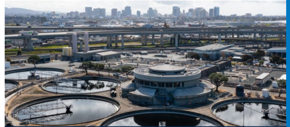
Secondary Treatment System Installed in the 1970s
