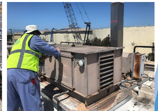
Failing HVAC Equipment
