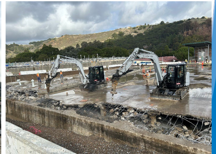
Demolish 95-year-old CCB
