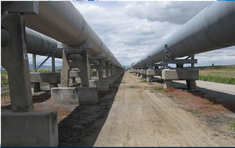
Mokelumne Aqueducts Nos. 1, 2, & 3 in the Delta
