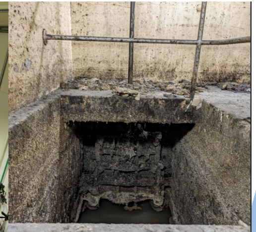
Rehabilitate Corroded Concrete
