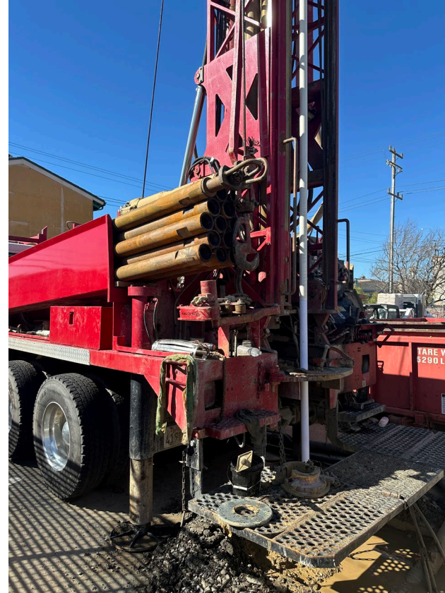
Groundwater Monitoring Well Installation
