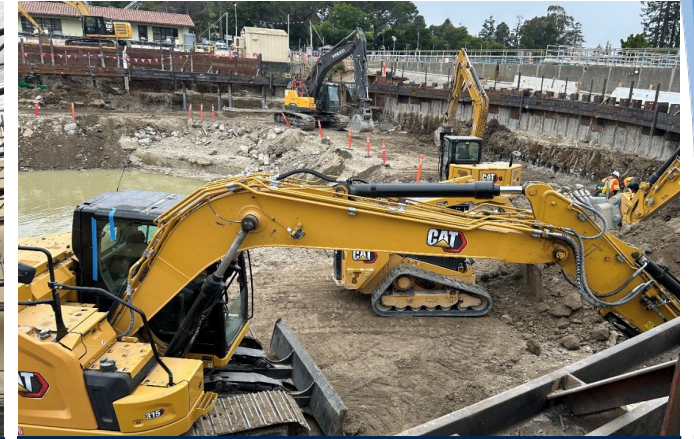
Excavation for New CCB
