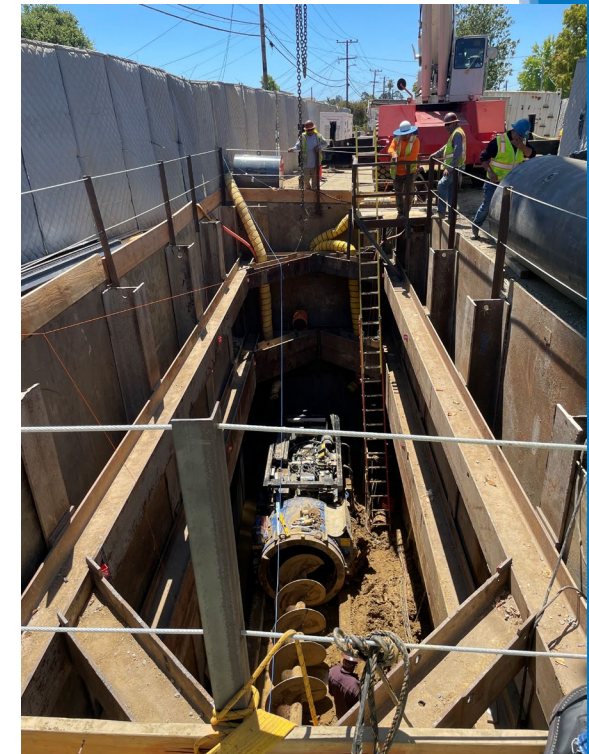
Typical Trenchless Installation
