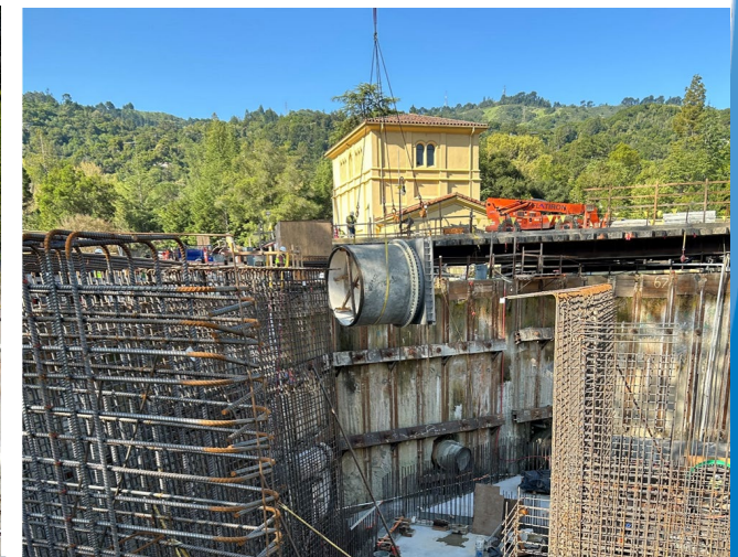
UV and CCB Structure Rebar and Piping
