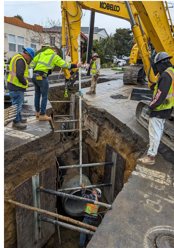
Typical Transmission Pipe Installation
