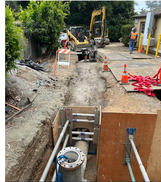
Rehabilitation of Yard Piping Palo Seco PP
