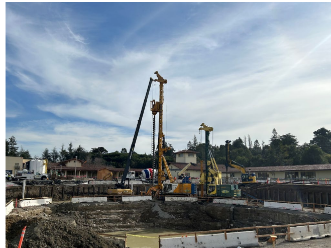
Installation of Drilled Shoring System
