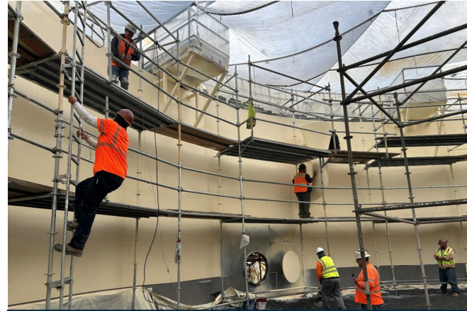
Workers Recoating Interior Tanks
