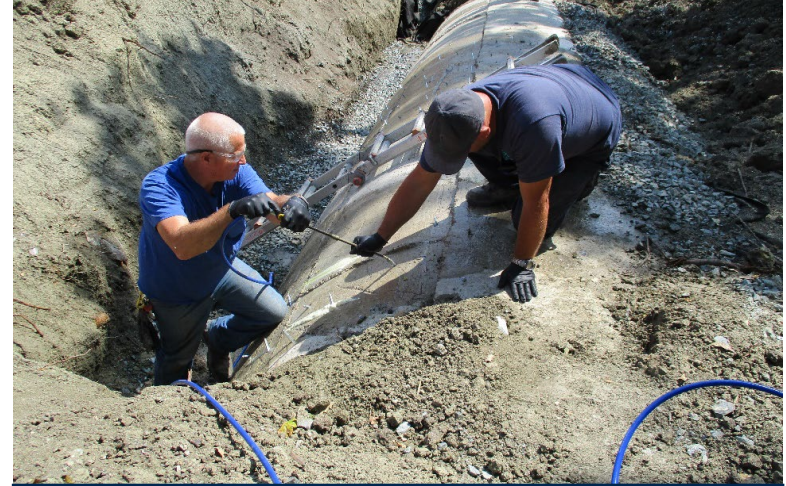
District Forces Repairing Leak on LAF 1 Pipeline
