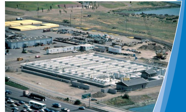
Oakport Originally Constructed in 1991
