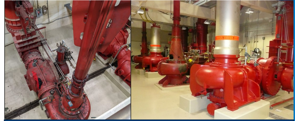
Replace Obsolete Pumps and Motors
