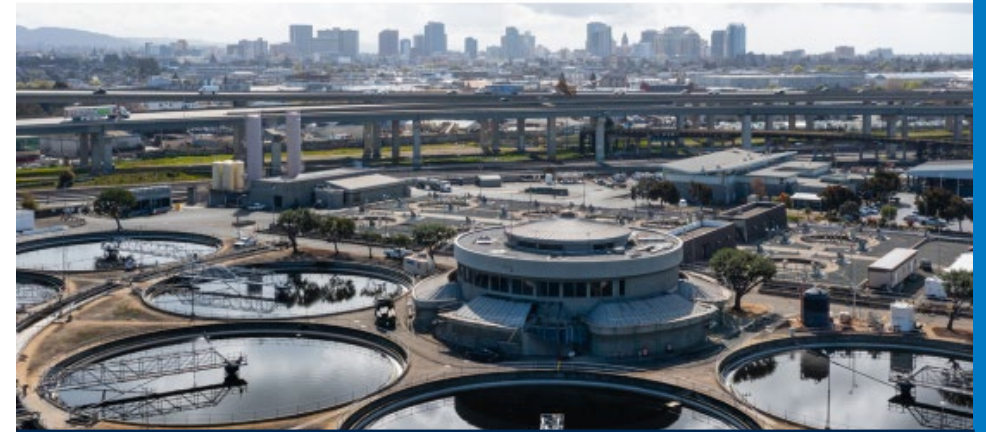
Secondary Treatment System Installed in the 1970s
