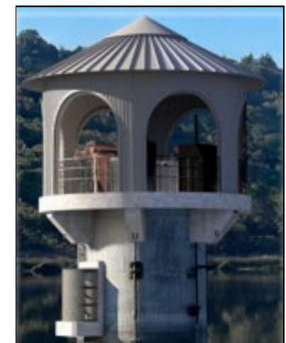
Metal Operating House
