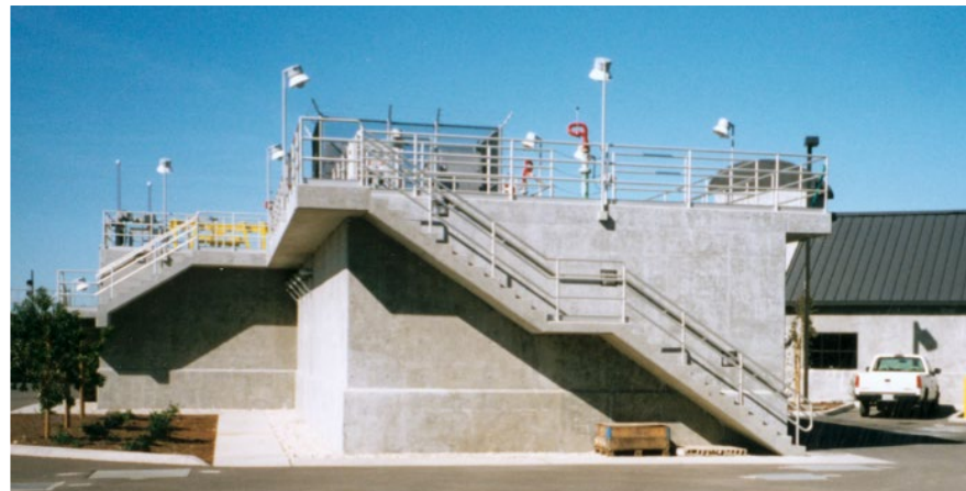
San Antonio Creek Originally Constructed in 1992
