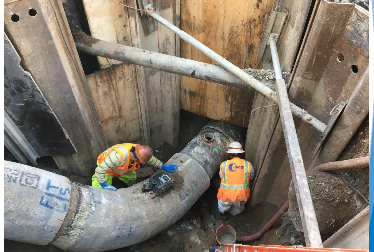
Typical 24-inch Transmission Pipe Installation
