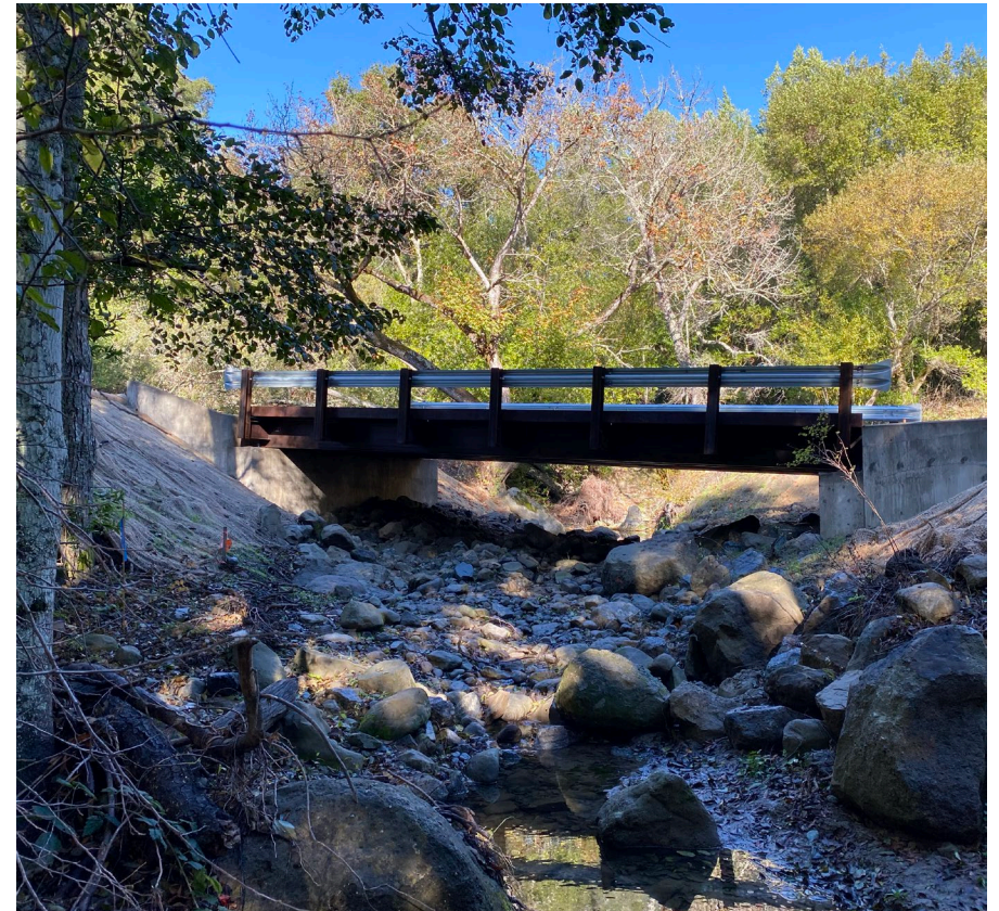
Two Dog Bridge Fish Passage Project
