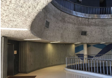
Interior Lobby – Original
