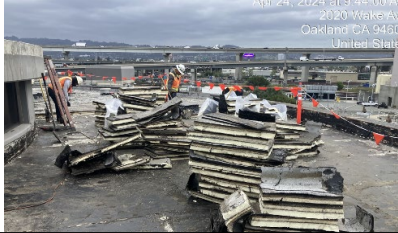
Demo Existing Roof
