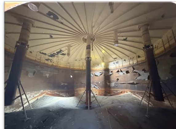
Remove and Replace Existing Interior Coatings
