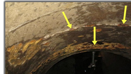
Corrosion on Welded Steel RAS Pipe Seams.
