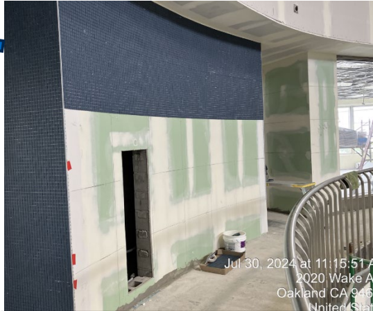
Interior 2nd Floor Tile Replacement
