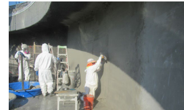
Concrete Wall Resurfacing
