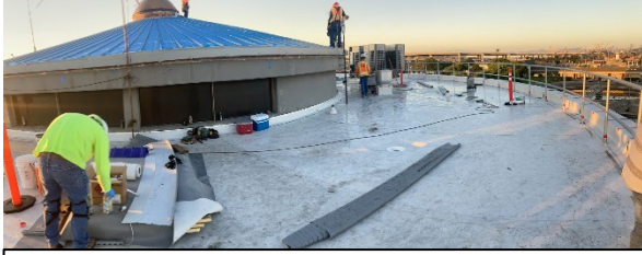
Install New Membrane Roofing
