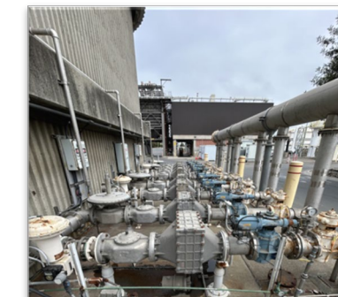
New Wiring and Controls for Flares
