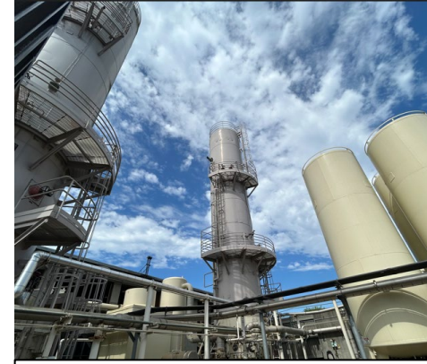
Cold Box Instrumentation Upgrades & Recoating
