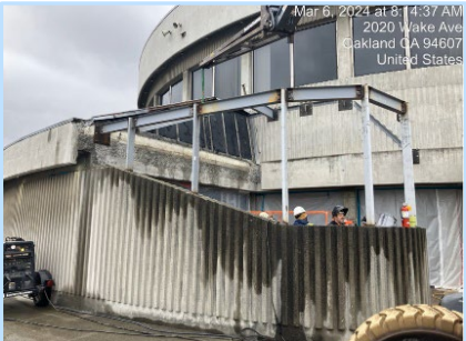
Exterior Framing for Expanded Lunchroom
