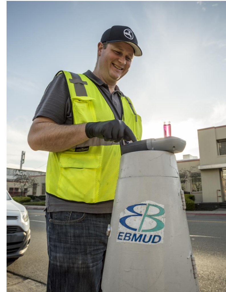
Water System Inspector sampling for chlorine
